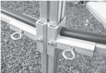
Install (1) allen bolt, (1) eye bolt and (2) brass nuts onto each of the (8) arm brackets. Loosely install the allen and eye bolts onto the arm brackets (do not tighten them).
