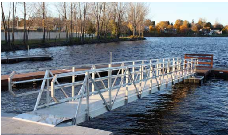
Steel Truss Floating Dock Plattsburgh, NY
