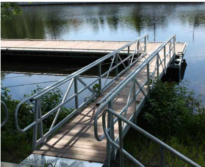
Commercial Steel Truss Floating Dock System Northumberland, NY
