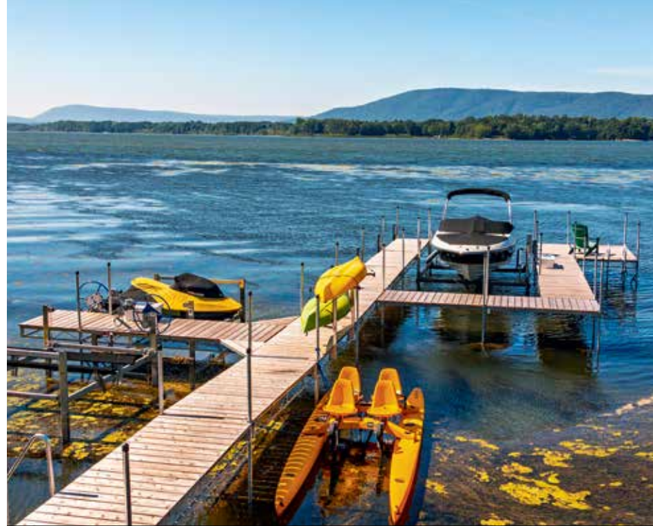
Docks in a "U-shape" configuration with 6,000 lb. vertical boat lift.
