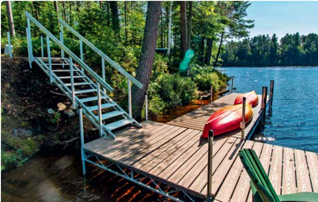
Above: Aluminum stair system on a site with a steep shoreline with 3' x 4' platforms as landings for each section of stairs.
