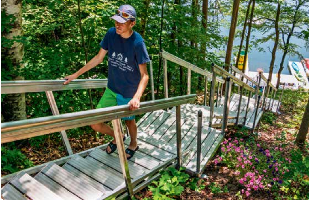
Above: Aluminum stair system on a site with a steep shoreline with 3' x 4' platforms as landings for each section of stairs.
