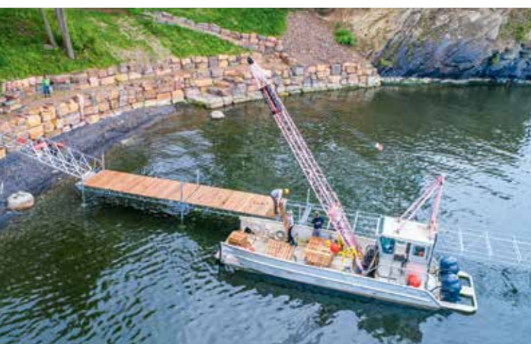
Mega dock system being installed by one of our crews.
