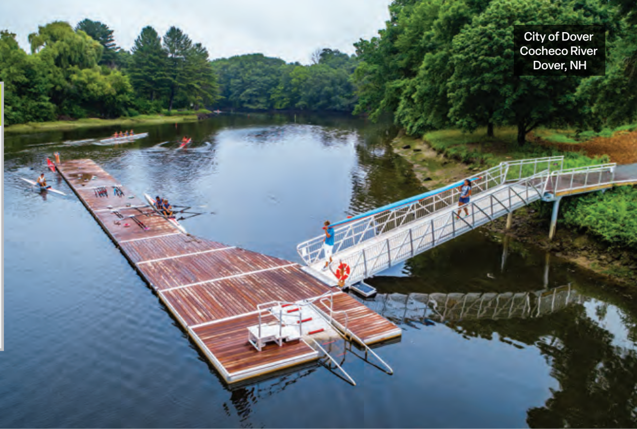
Above: Heavy duty aluminum frame Rowing Dock with 38' × 7' aluminum gangway and commercial kayak launch with ADA transfer platform (see page 57). Our custom pile dock serves as a shore anchor.
