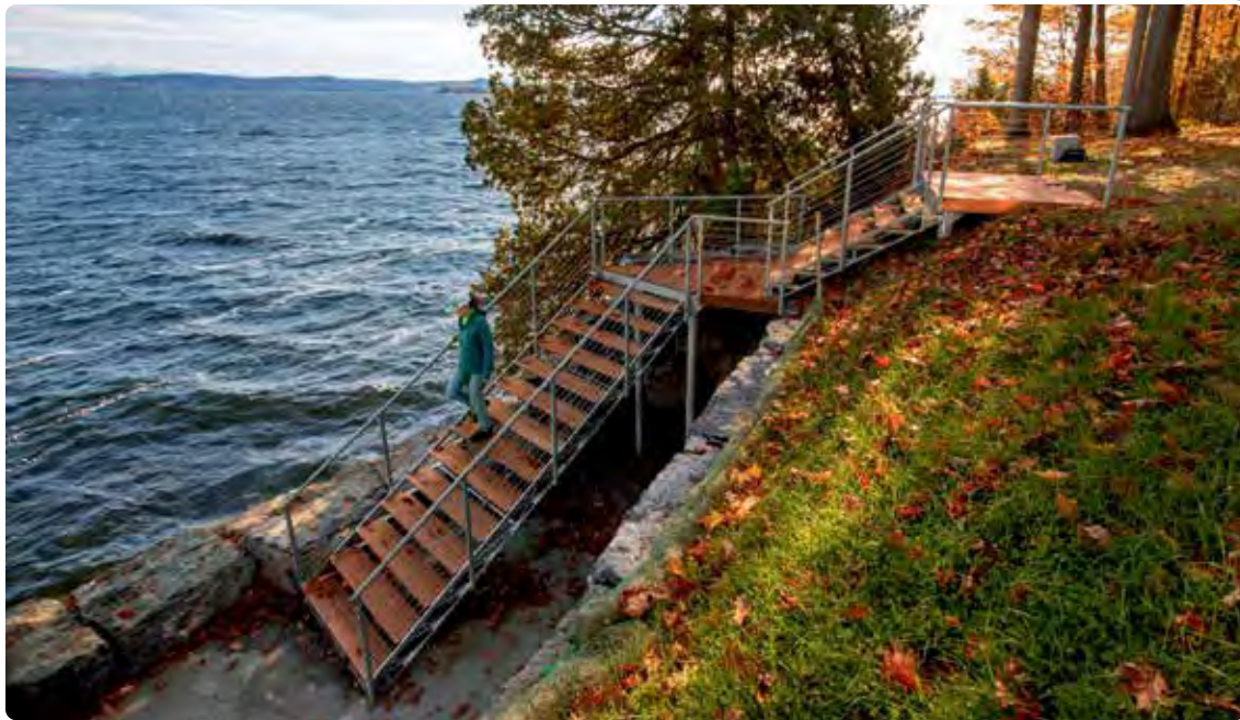
Above: Stairs with stainless steel cable rail and Ipe stair treads.
