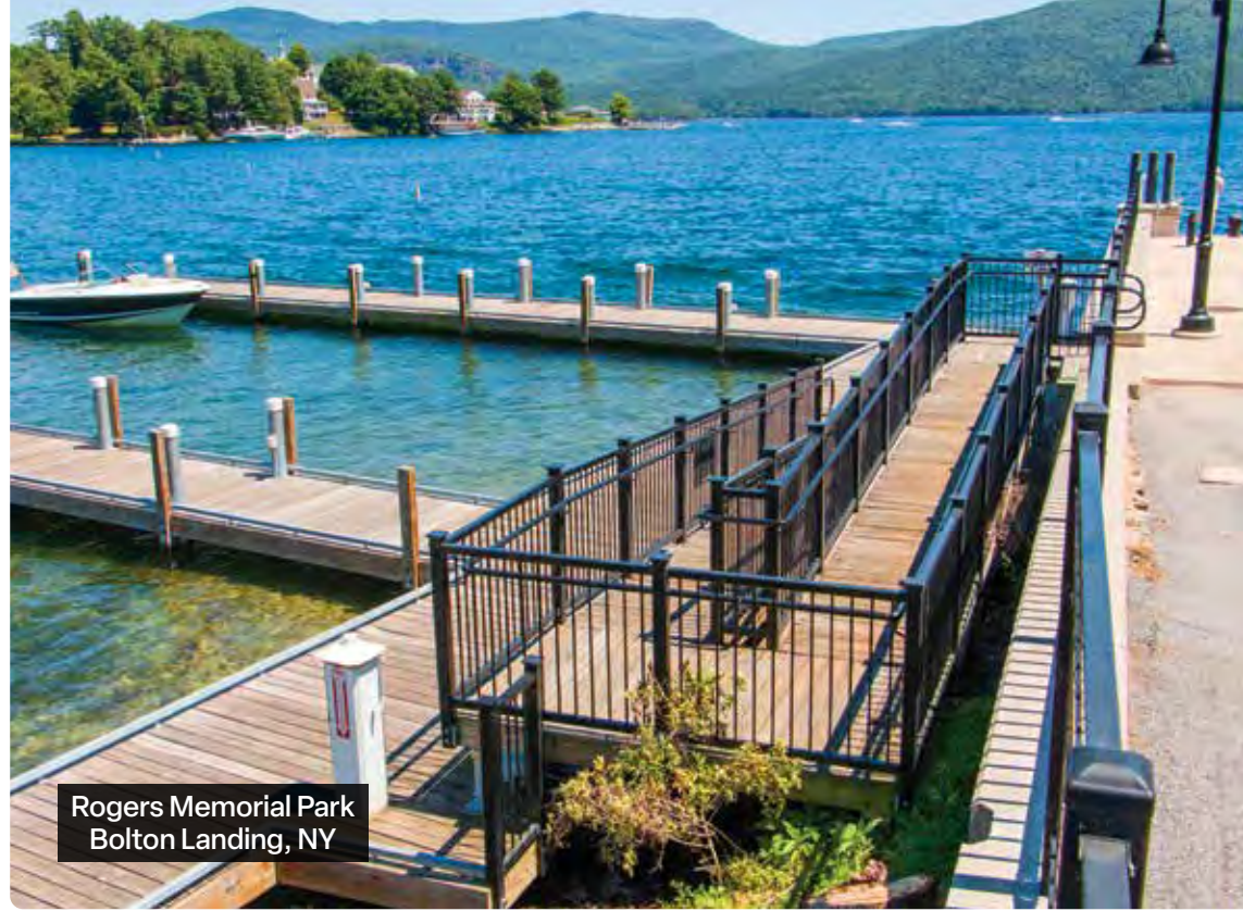
ADA access ramp transitions from the upper pier area to our commercial pile dock.
