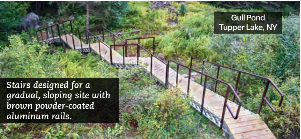
Stairs with stainless steel cable rail & shoreside platform for a site with no shoreline.
