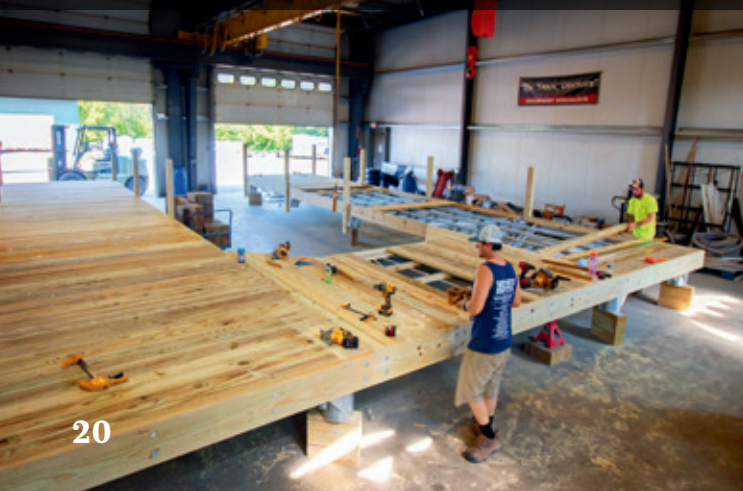
Final decking being applied in our workshop.
