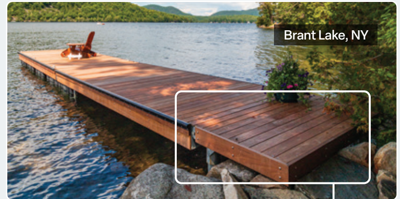
Permanent pile platform shore anchor.
