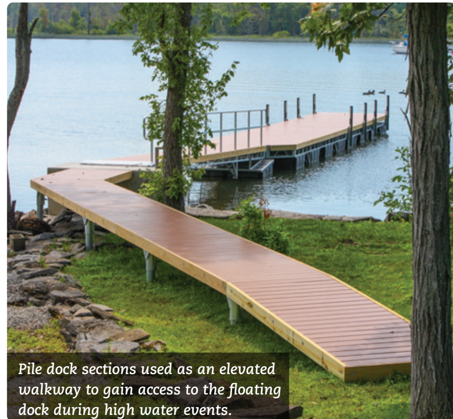
Heavy duty aluminum floating dock with Ipe decking.
