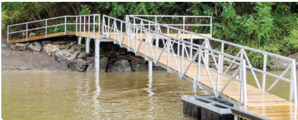
Above Top: T-shaped steel truss floating dock system. Above: Our shoreside platform as the shore anchor.
