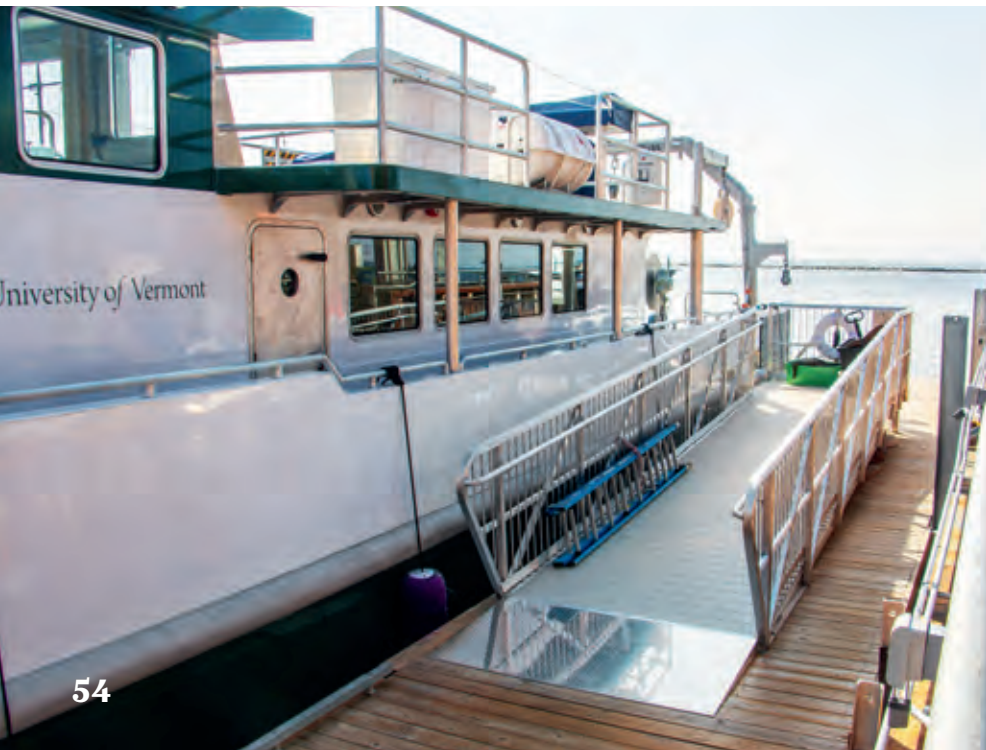
Above: 6' x 48' aluminum gangway to steel truss floating dock designed for a high freeboard marine research vessel. Below Left: ADA access boarding gangway with spindle rail. Below Right: Both gangways during fabrication in our workshop.
