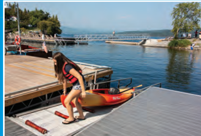
Launch ramp with rollers & non-slip decking.
