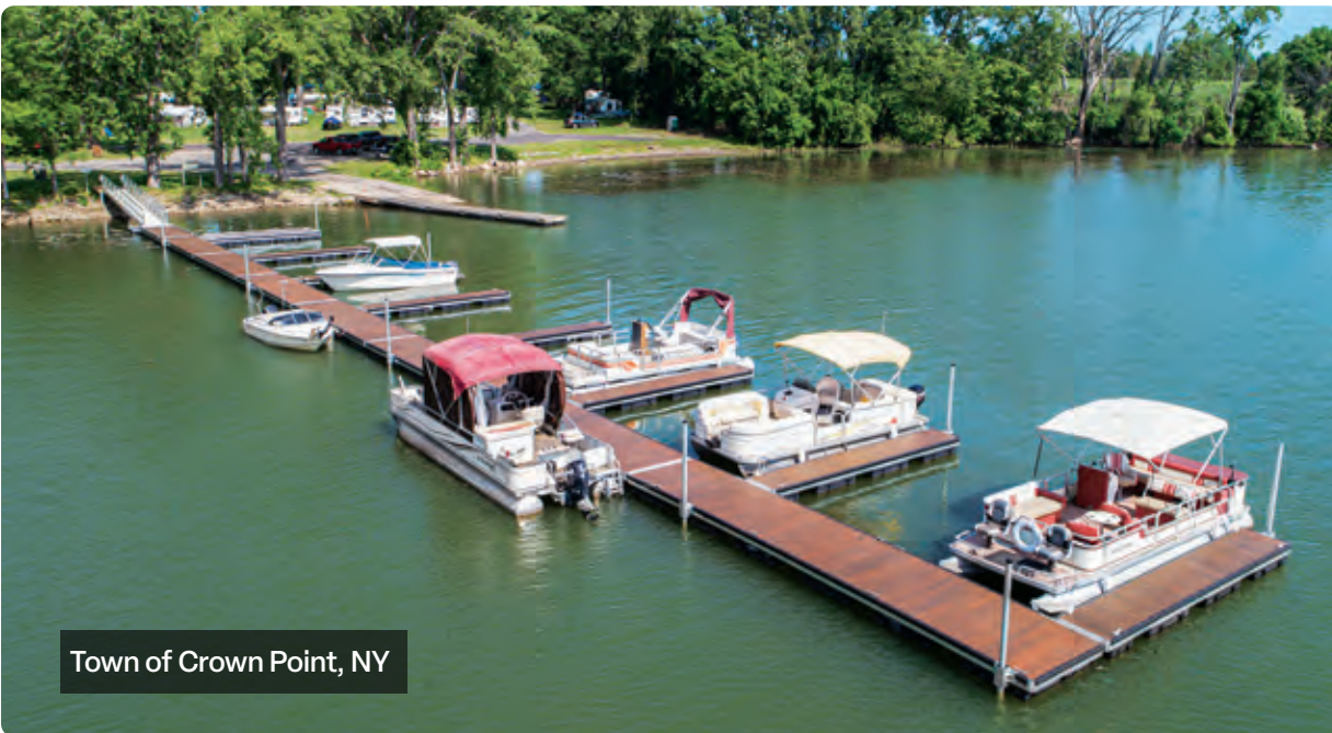
Heavy duty aluminum floating "paddle" dock with low freeboard, designed for easy entry for kayaks, canoes and other crafts.
