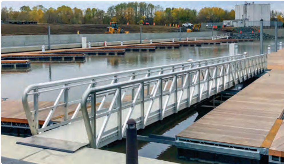
5' x 80' ADA compliant commercial aluminum gangway
