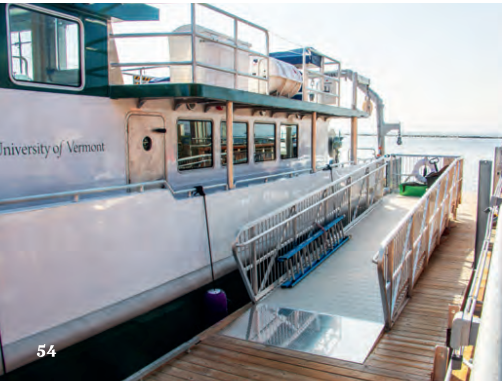
Above: 6' x 48' aluminum gangway to steel truss floating dock designed for a high freeboard marine research vessel. Below Left: ADA access boarding gangway with spindle rail. Below Right: Both gangways during fabrication in our workshop.
