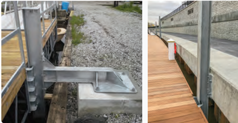
Above: Vertical beam shore mounts.
