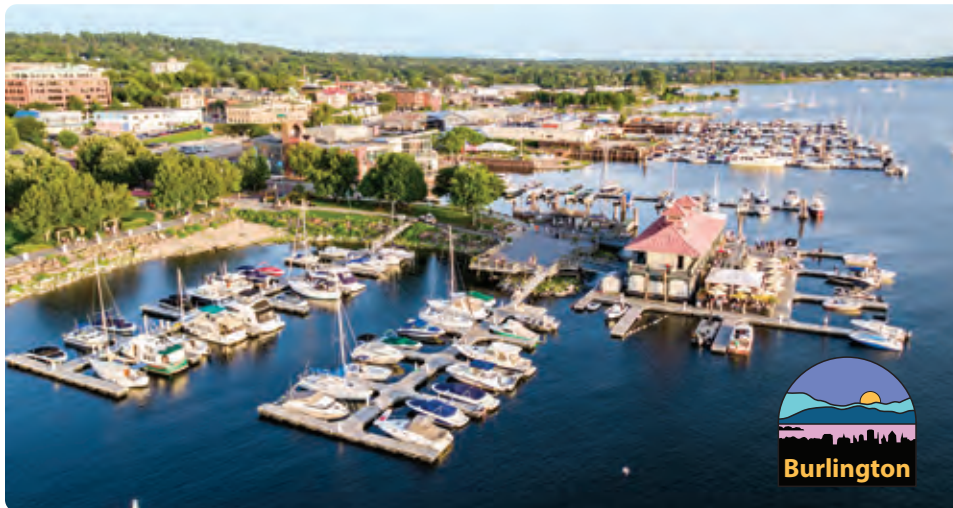
Commercial Marina Floating Dock System City of Burlington, Lake Champlain, VT
