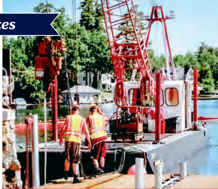
Pile driving from 4" to 12" in diameter (larger if necessary)
