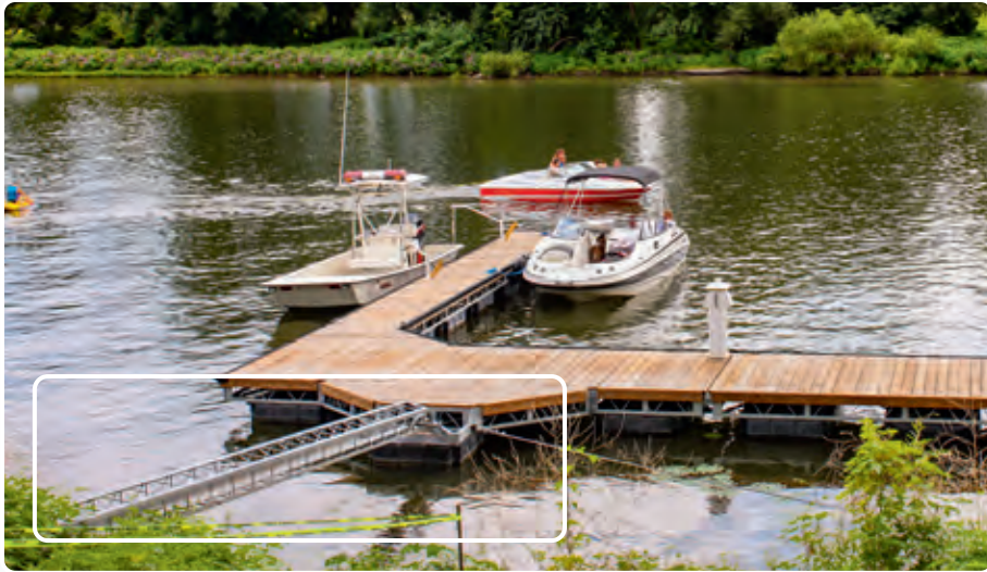
Above: Stiff arm anchoring example.
