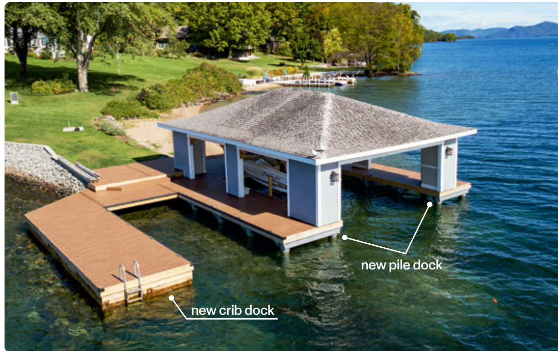
Above: New boathouse foundation complete. Above Right: Lifting and securing the existing boathouse to install new pile dock.
