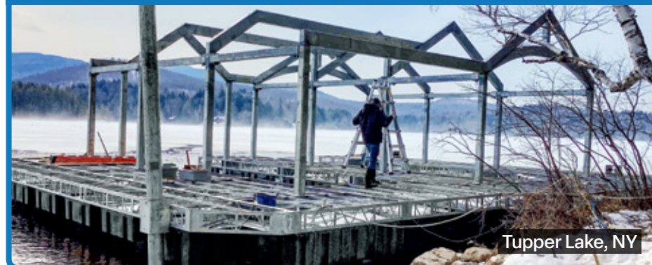
Above: Floating boathouse foundation and support structure during production in our shop. Below: Support structure being assembled on site.
