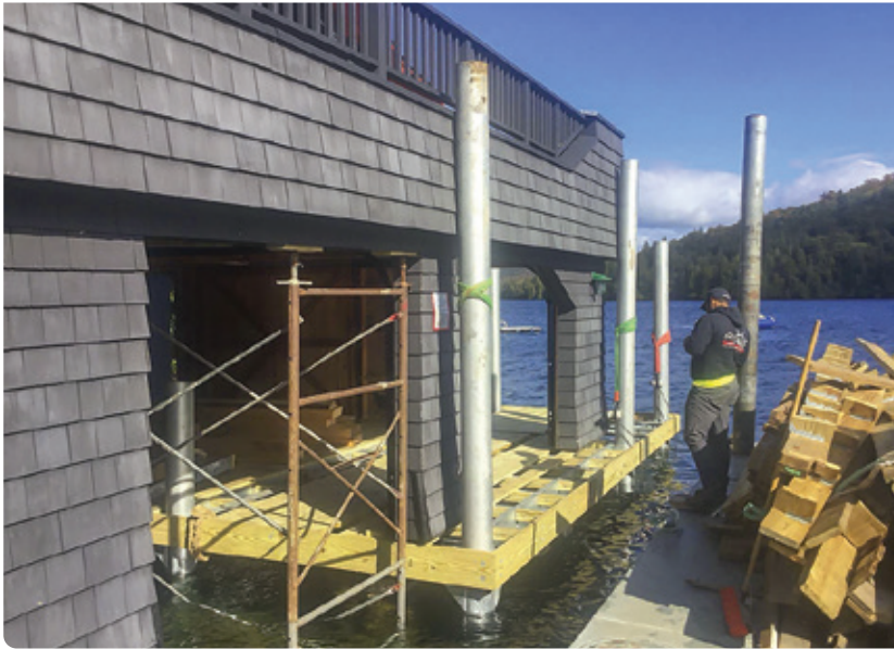
Installing new pile dock under the existing boathouse structure.
