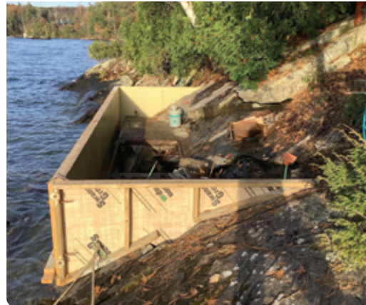
Above Left: Forms in place for concrete pad.
