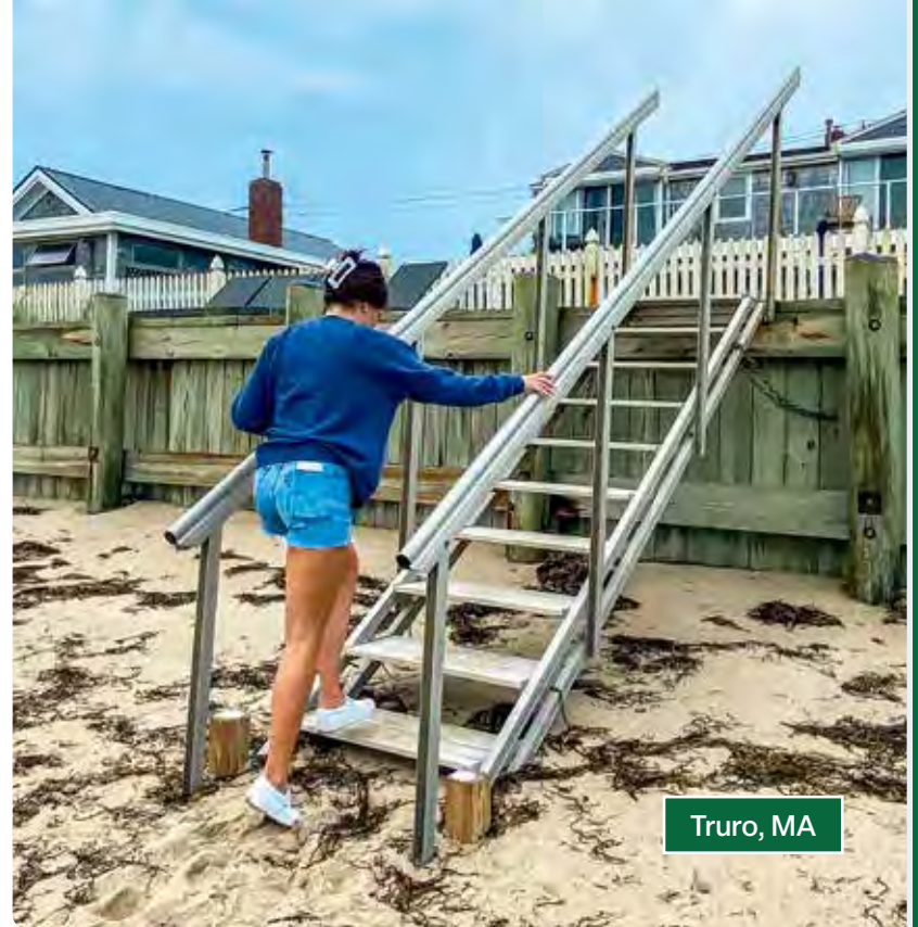
Above: Stair system on an oceanfront property can be easily removed in winter to protect the stairs.
