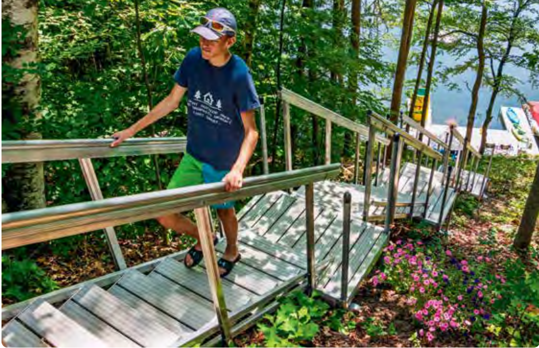
Above: Aluminum stair system on a site with a steep shoreline with 3' x 4' platforms as landings for each section of stairs.
