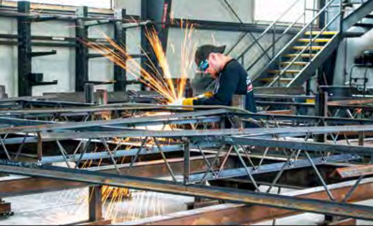
Dock frames being manufactured in our Vermont Facility.
