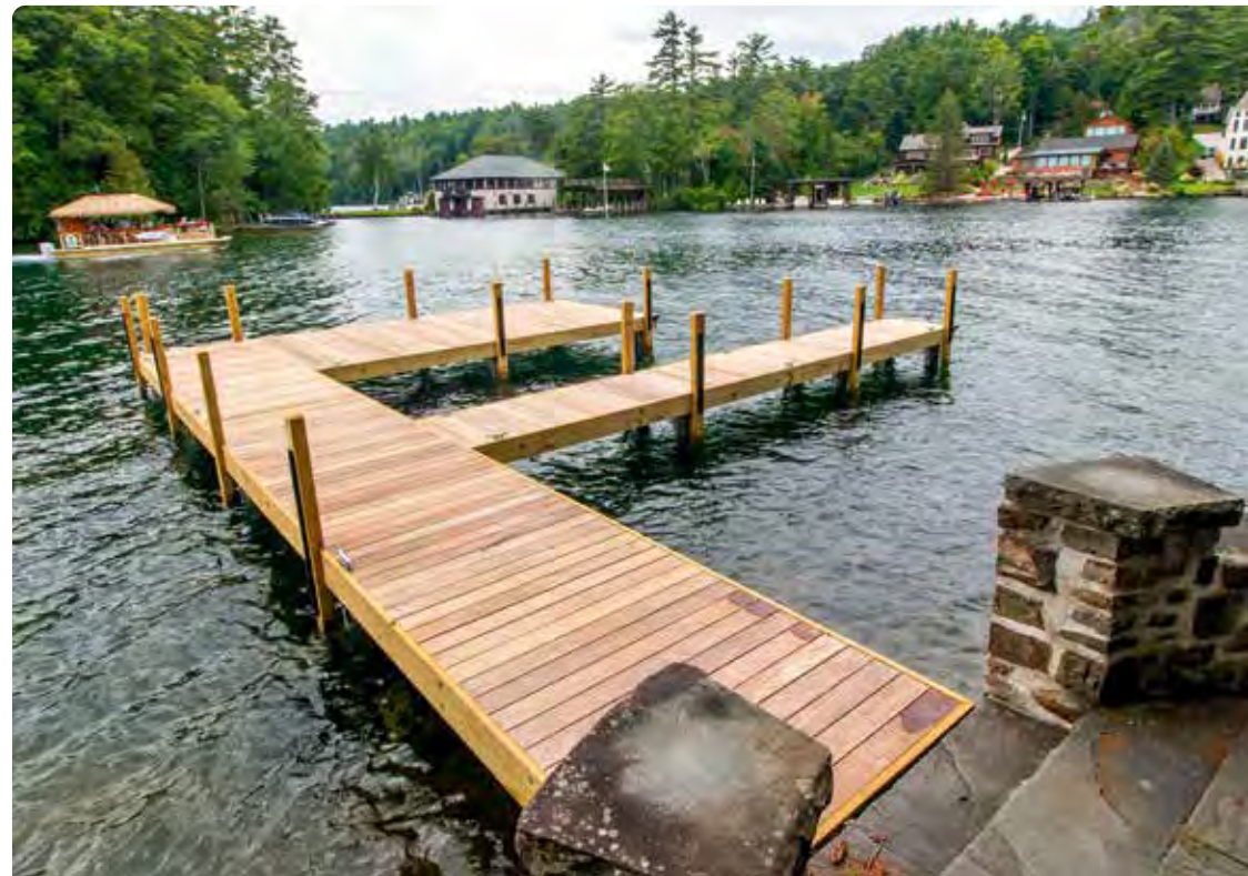
Above: Pile Dock with rub strakes and piles cut below the decking. Below: Pile Dock with Ipe decking and rub strakes.
