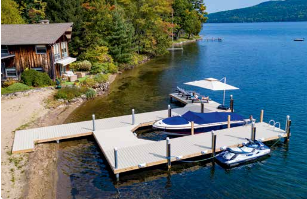
Above: U-shaped pile dock with WearDeck decking in Barefoot Sand and piles above the decking.
