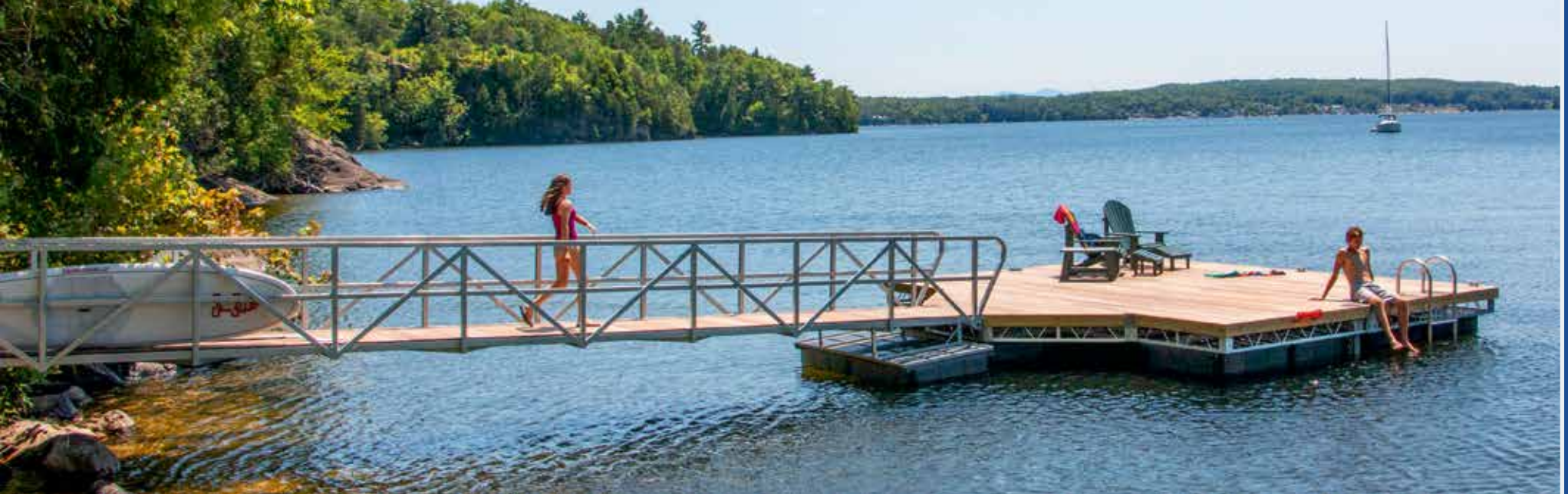
Above: Galvanized steel truss floating dock and gangway with Ipe decking.
