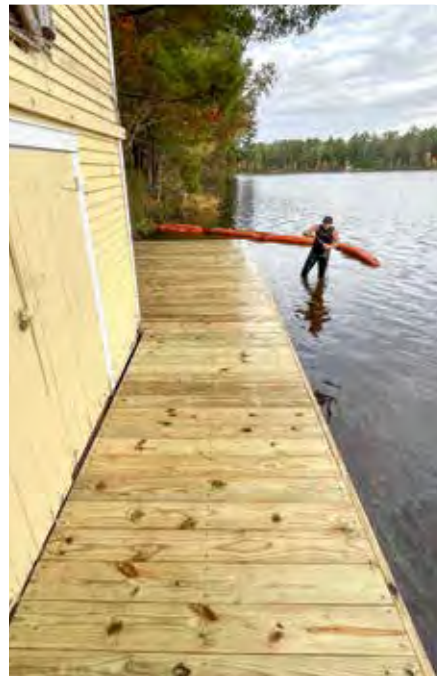
Crib rehabilitation: The top 5' of timber was removed and replaced, along with new decking.
