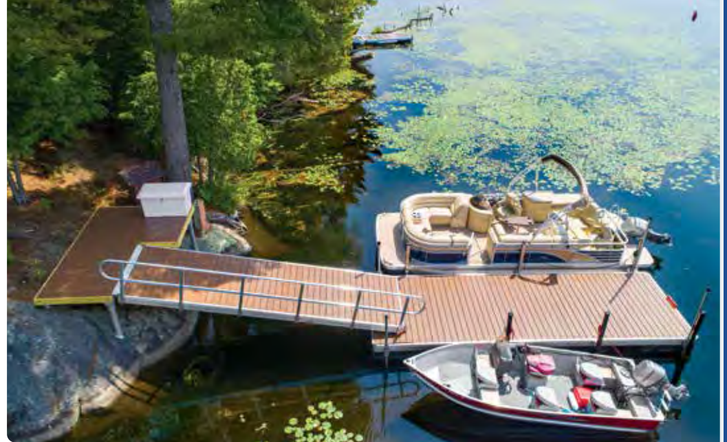
Above: Our pile platform serves as a shore anchor for a gangway ramp and a floating dock.
