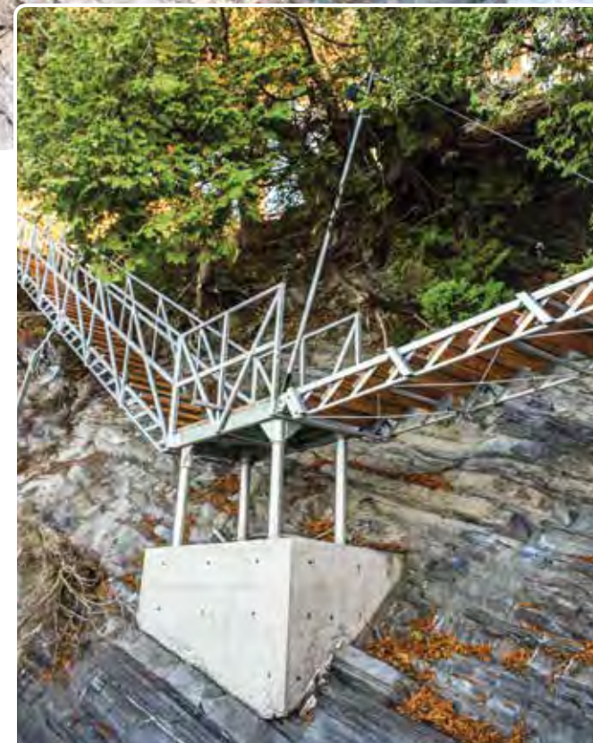
Freespan stairs with lower section that hinges for winter storage.
