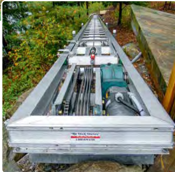
Electric Direct Drive Motor during installation without drive cover.
