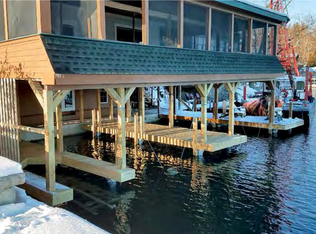
Above: New permanent pile foundation in place.
