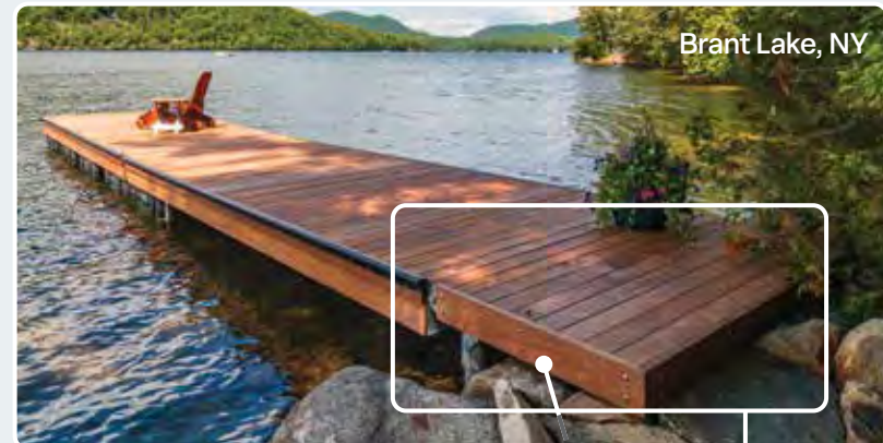
Permanent pile platform shore anchor.
