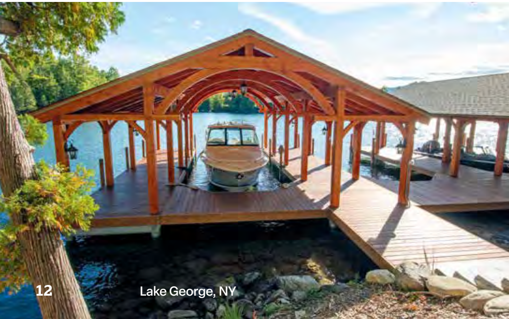
Three-slip permanent pile dock with Ipe decking serves as the foundation for this boathouse. Post and beam roof structures completed by others.
