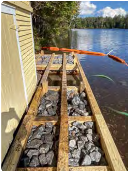
Crib rehabilitation: The top 5' of timber was removed and replaced, along with new decking.
