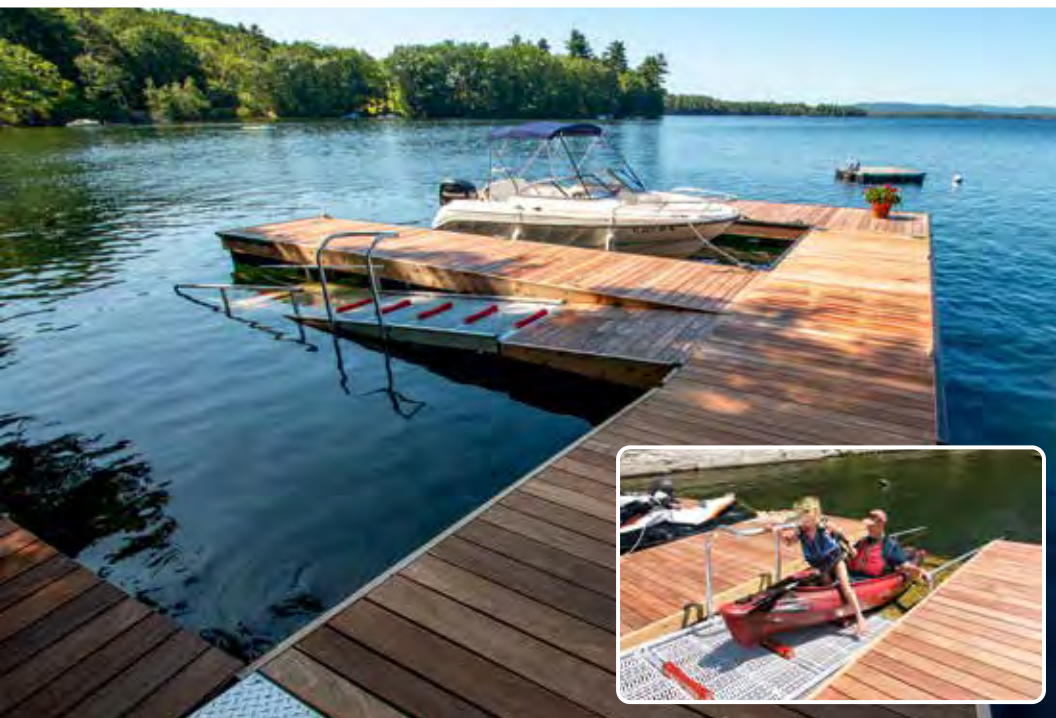
Galvanized steel truss floating dock with launch ramp and Ipe decking.
