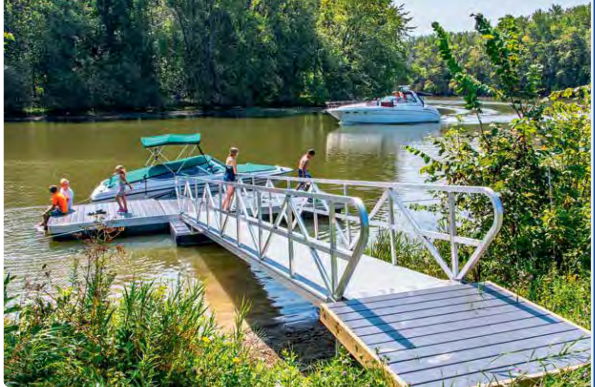
Above: Our pile platform as a shore anchor for gangway and floating dock.
