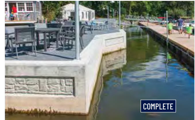
Shoreline Restoration and new Marina at the iconic Basin Harbor Resort
