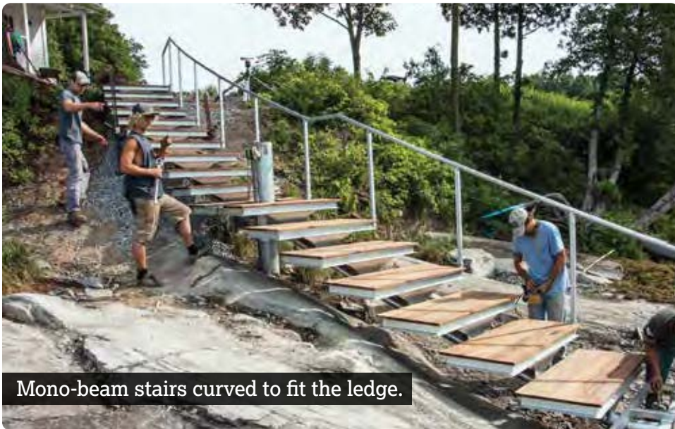
Stairs with stainless steel cable rail and black powder coated railings. Integrated with our shoreside platform for a site with no shoreline.
