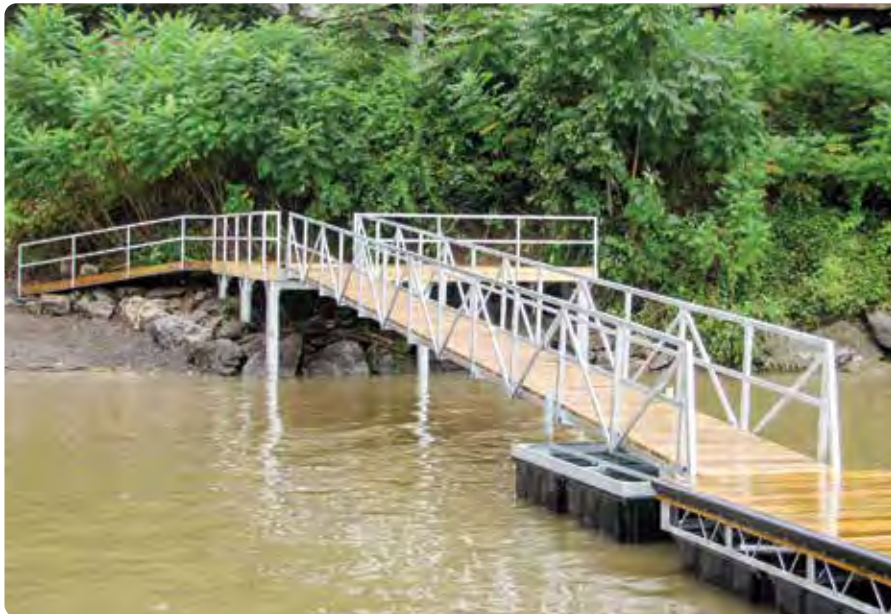
T-shaped steel truss floating dock system (above right) with our shoreside platform (above left) as the shore anchor.
