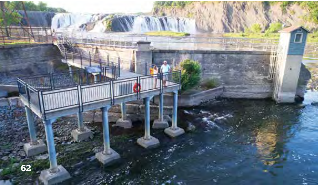
112' long industrial freespans stairs and public viewing platform (below left) at Brookfield Hydro-power Plant, Cohoes, NY
