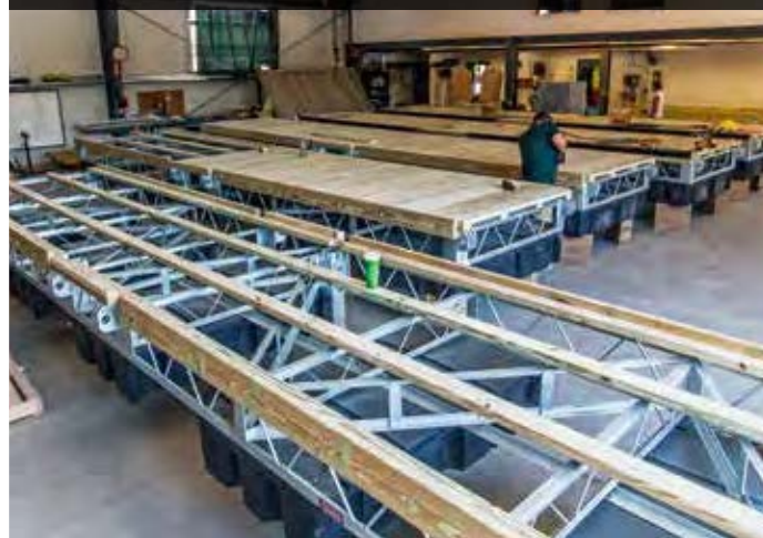
Decking being installed in our woodshop.
