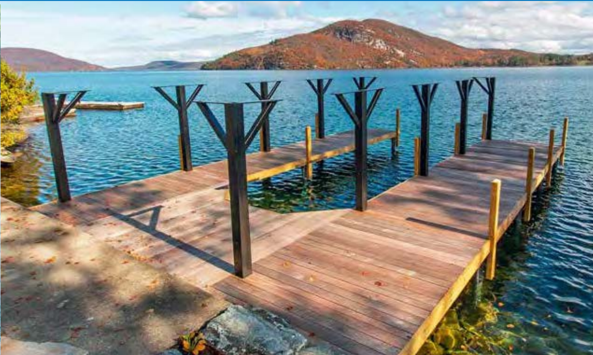
Pile dock boathouse foundation with Ipe decking and powder coated support posts in place for future roof.
