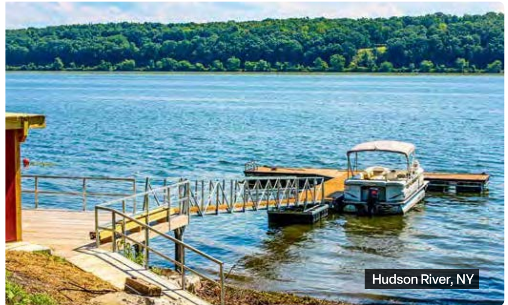
T-shaped steel truss floating dock system (above right) with our shoreside platform (above left) as the shore anchor.
