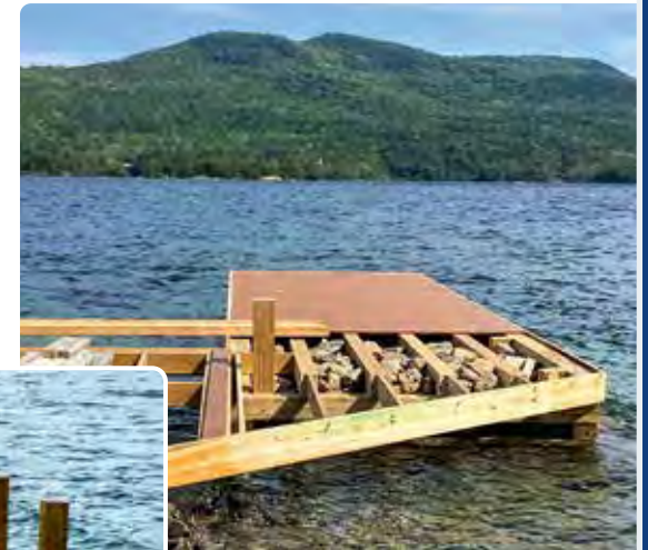
Above: New crib dock and pile dock boathouse foundation for an existing boathouse. Boathouse was lifted and secured to install new pile dock.
