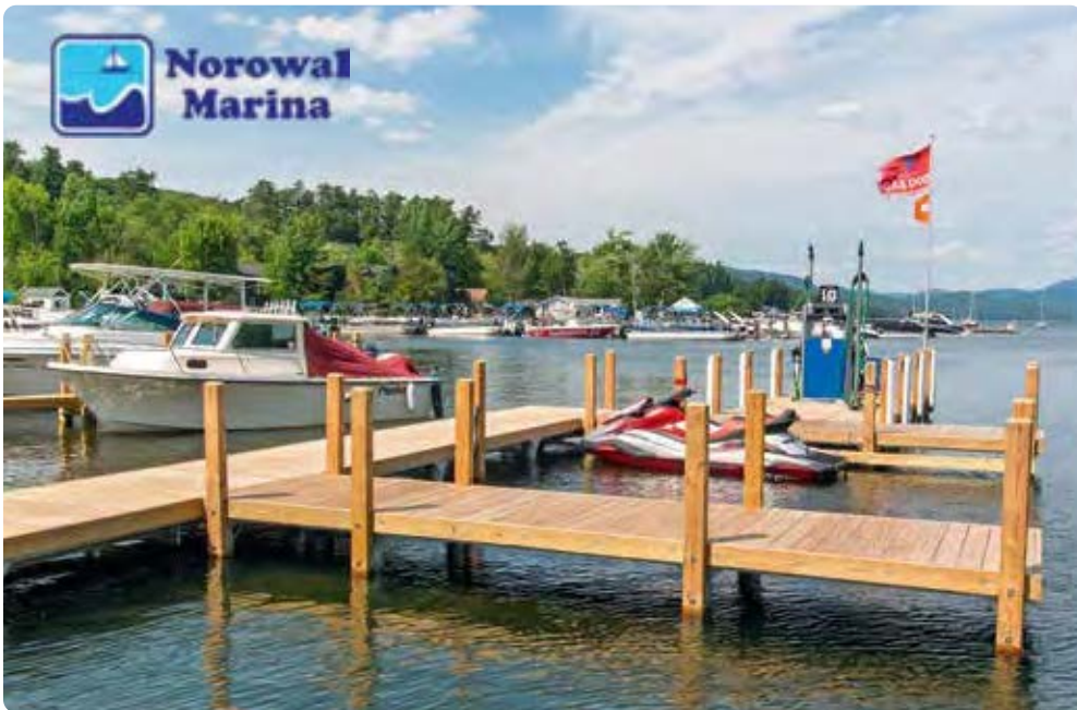
Above: Pile Docks at Norowal Marina on Lake George. See more of our Commercial Products on pages 54-63.
