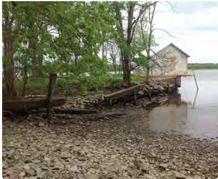
Condition of historic pier prior to preservation.
