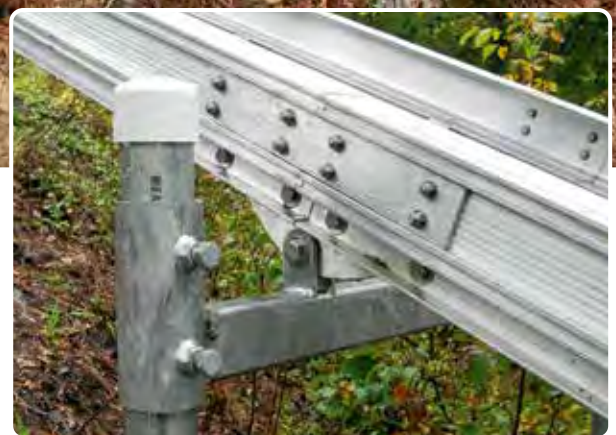
Example of one-piece track support & splice connection.
