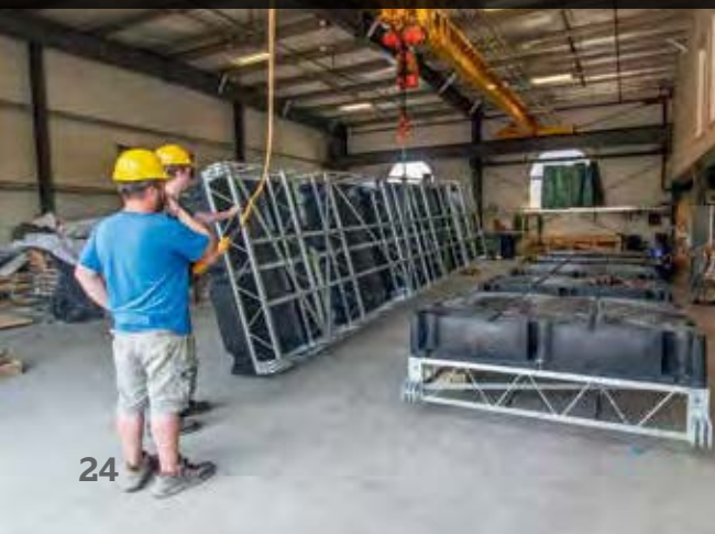
Flotation being installed onto dock frames.
