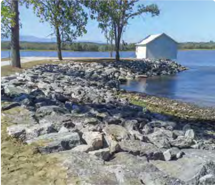
Historic pier preservation, Hudson River, NY
