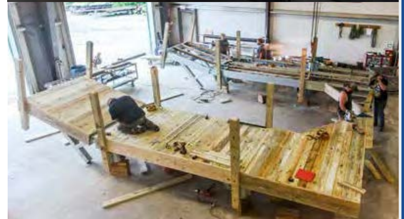
Decking being applied in our woodshop.
