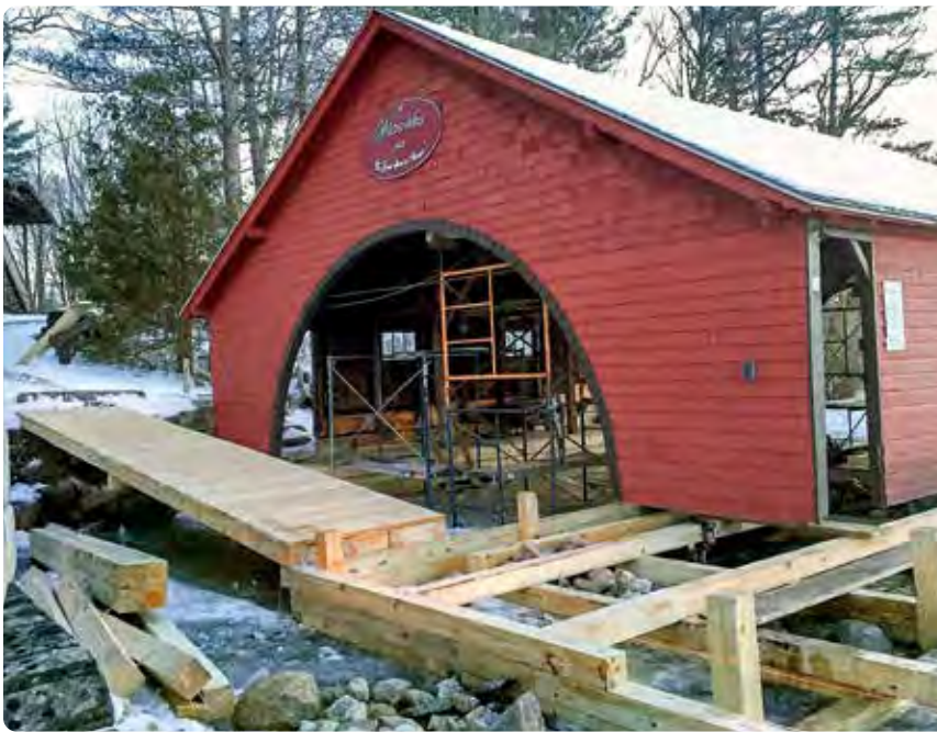
Above Left: Foundation replacement for historic boathouse. Right: Completed foundation and dock replacement.
