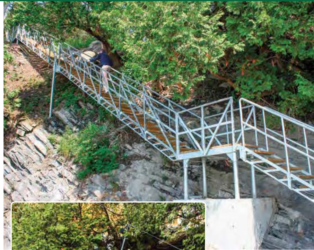
Freespan stairs with lower section that hinges for winter storage.
