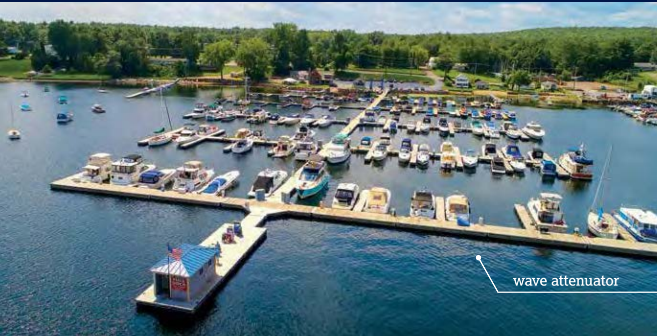
Above Left: Commercial marina system with wave attenuators incorporated into the dock system. Above Right Top: Wave attenuator section during final production in our shop. Above Right Bottom: wave attenuator section during initial installation.
