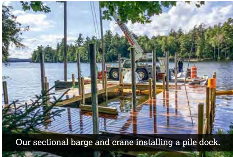
Pile dock boathouse foundation with Ipe decking and powder coated support posts in place for future roof.
