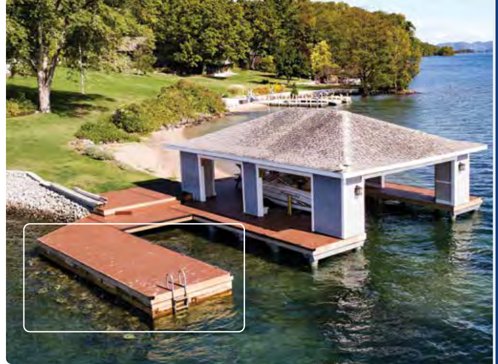
Above: New crib dock and pile dock boathouse foundation for an existing boathouse. Boathouse was lifted and secured to install new pile dock.
