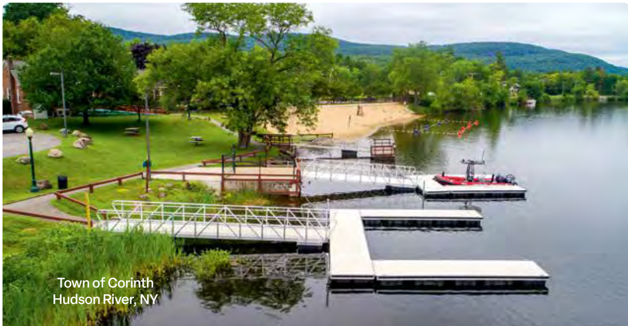
Aluminum floating "paddle" dock with low freeboard for easy entry for kayaks and other crafts.
