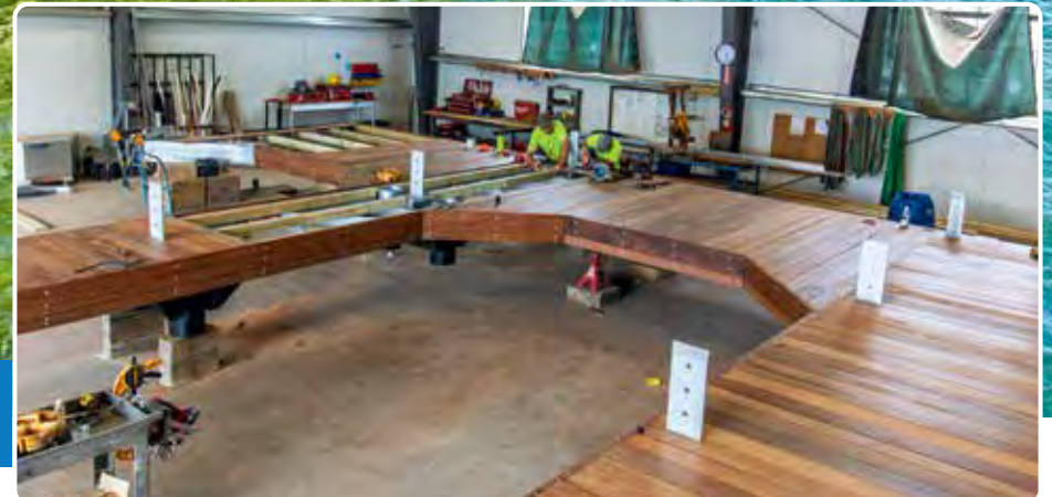
Pile dock in our woodshop with boathouse support mounts in place for future sundeck structure posts.
