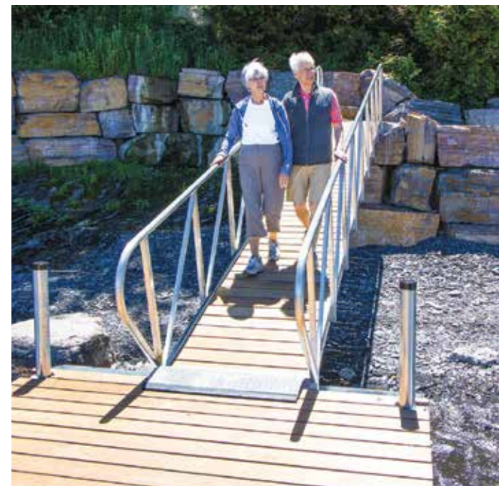
Our Mega dock used as a shoreside access / shore mount for a custom floating dock at a site that experiences heavy seasonal water fluctuation.
