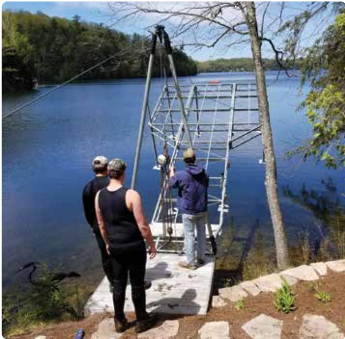
Above: One of our crews raising an articulating dock for winter storage.
