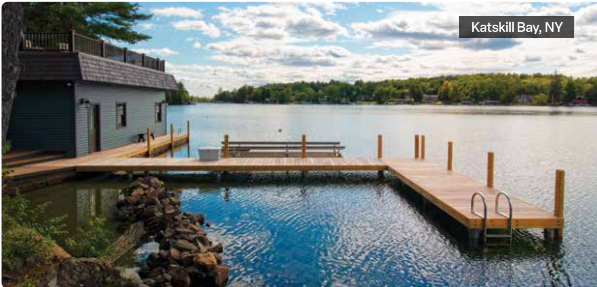
Above: Pile dock with Ipe decking, rub strakes and two boat slips. Below: L-shaped pile dock as an extension to an existing boathouse.
