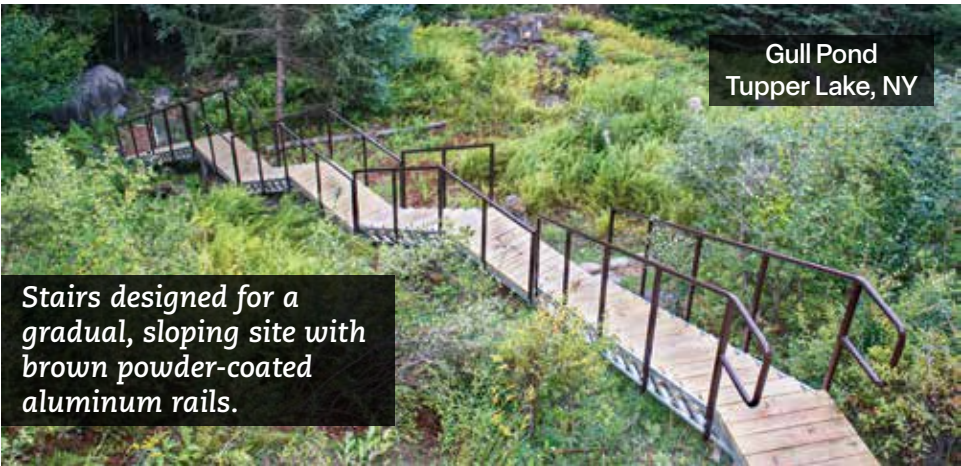
Freespan stair system & shoreside platform for a site with no shoreline
