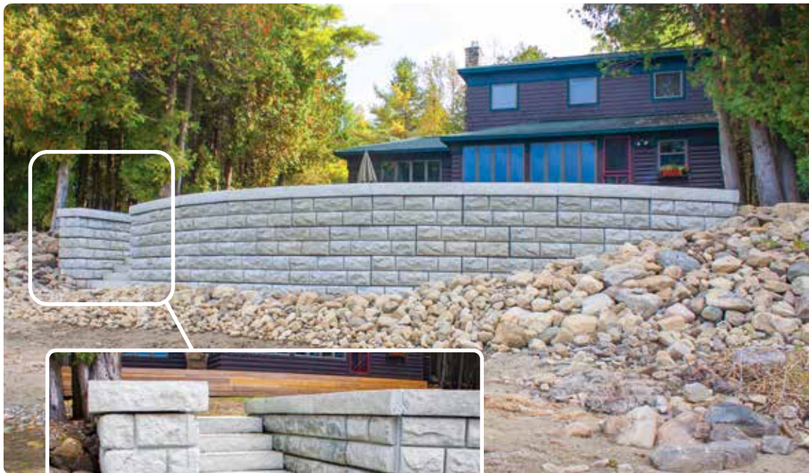
Above: Stacked decorative concrete retaining wall with integrated stairs.
