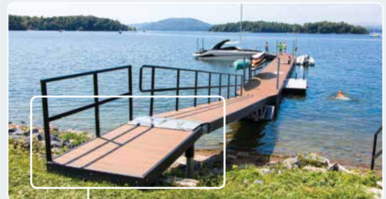
Permanent pile platform shore hitch.
