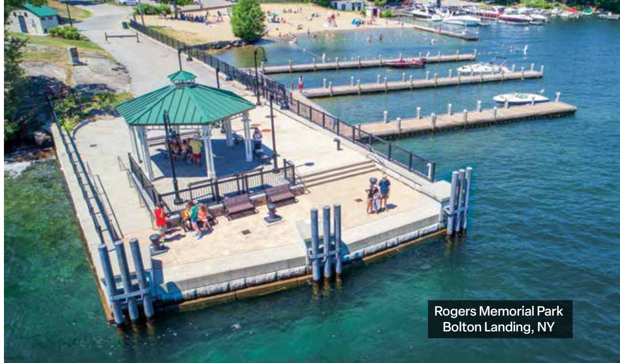
Above: Complete pier replacement and new pile dock.
