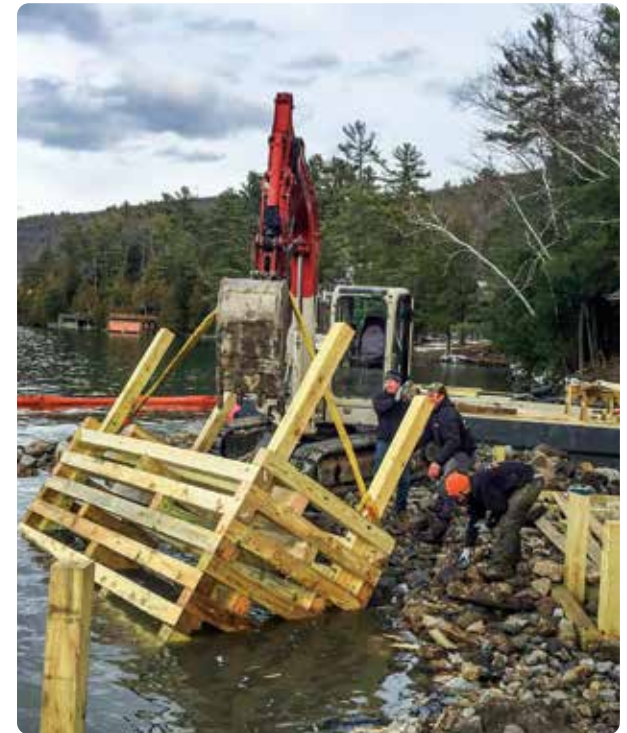
Crib dock replacement in progress
