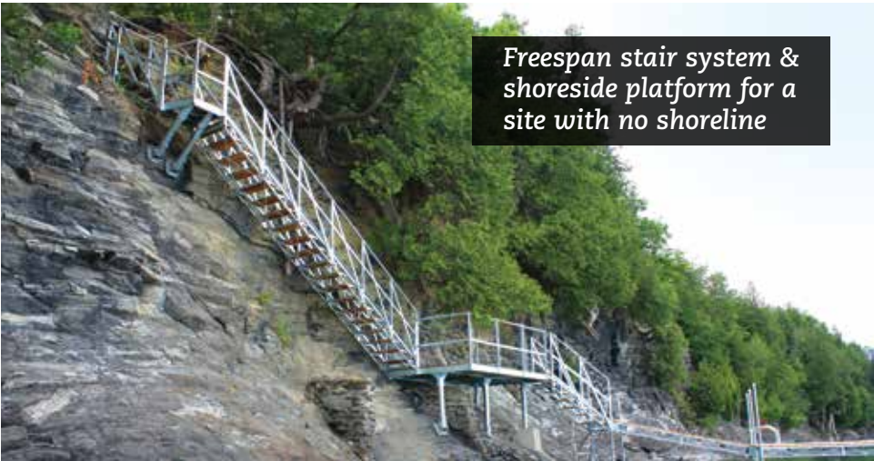
Stairs with stainless steel cable rail connected to our shoreside platform
