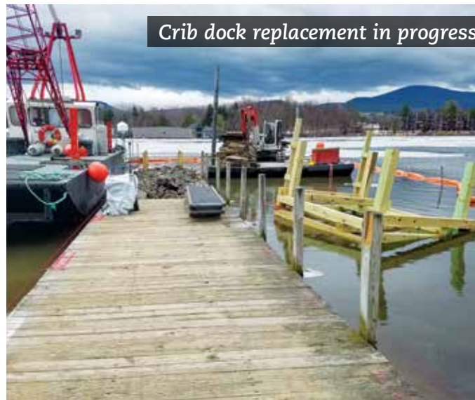
Old cribs being removed
