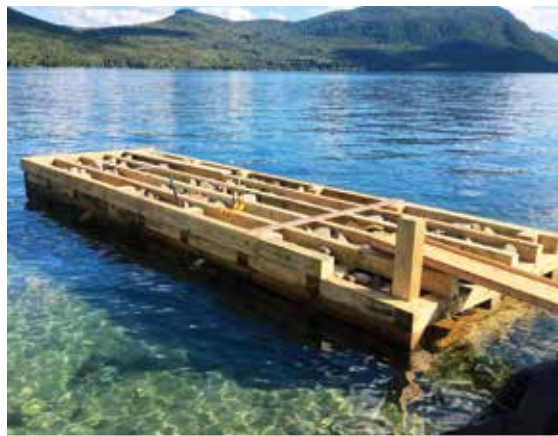
Crib dock replacement in progress.
