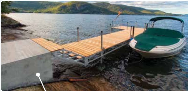
Concrete pad as a shore hitch.
