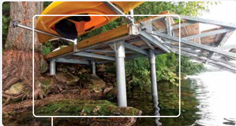
Permanent pile platform shore hitch.
