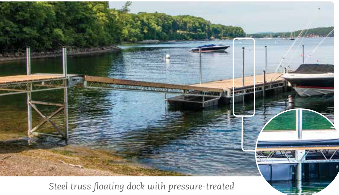
Steel truss floating dock with pressure-treated decking. Inset: Example of internal mounted anchor chain tube - shown with deck access plate removed.
