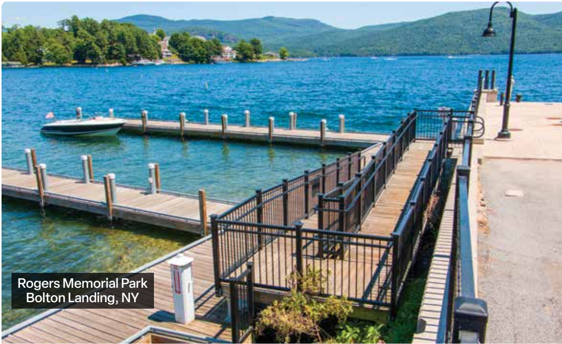
ADA access ramp transitions from the upper pier area to our commercial pile dock.
