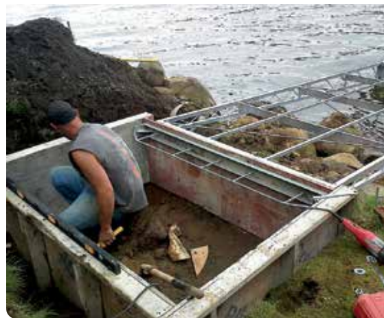
Above Top: Straight articulating dock with cedar decking. Above Left and Right: Concrete pad being formed then shown completed to serve as the shore hitch for an articulating dock.
