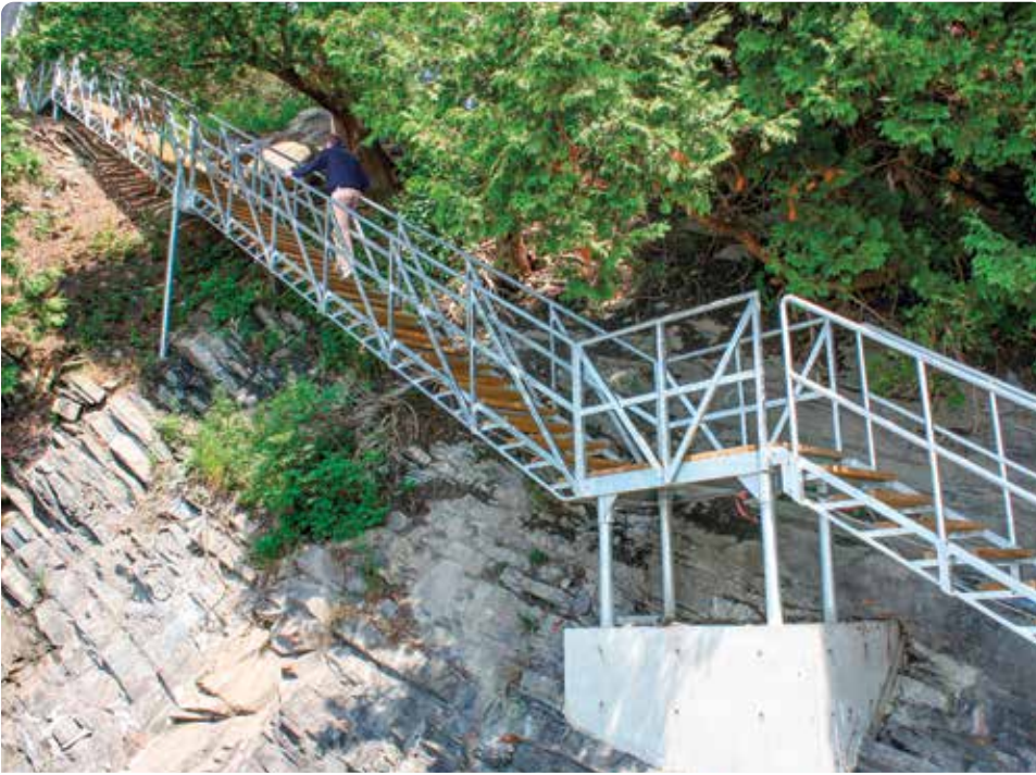
Freespan stairs with lower section that hinges for winter storage.
