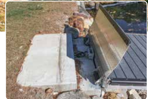
Heavy duty aluminum docks at homeowners association with concrete pads as shore hitches.
