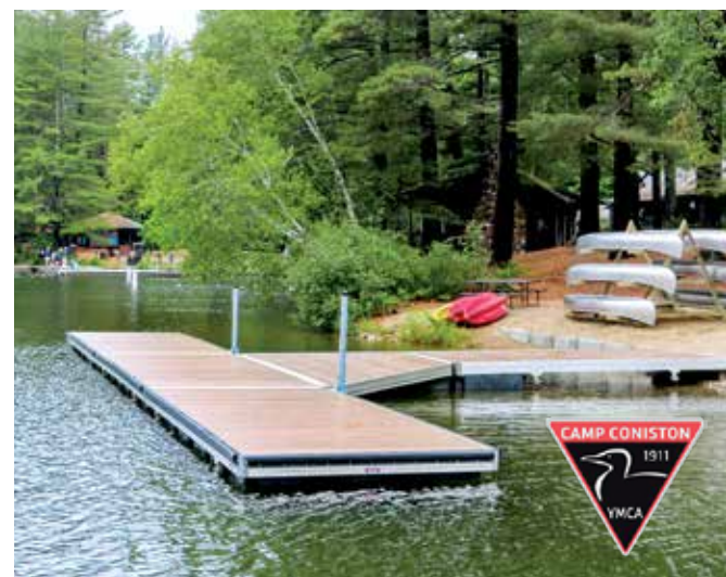
Custom 16' wide ramp.
