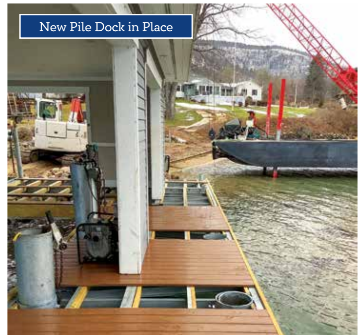
Above: New boathouse foundation complete. Above Right: Lifting and securing the existing boathouse to install new pile dock.
