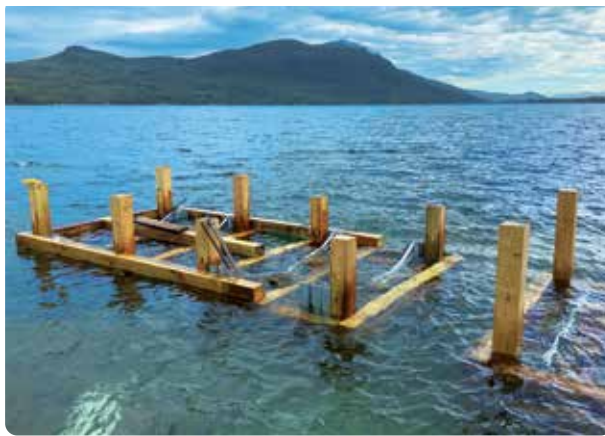
Crib dock replacement in progress.
