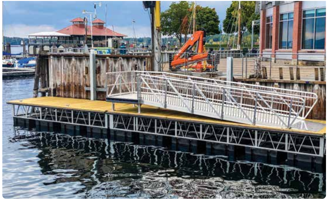
Above: Boarding gangway with spindle rail – gangway designed for ADA access to a high freeboard marine research vessel.
