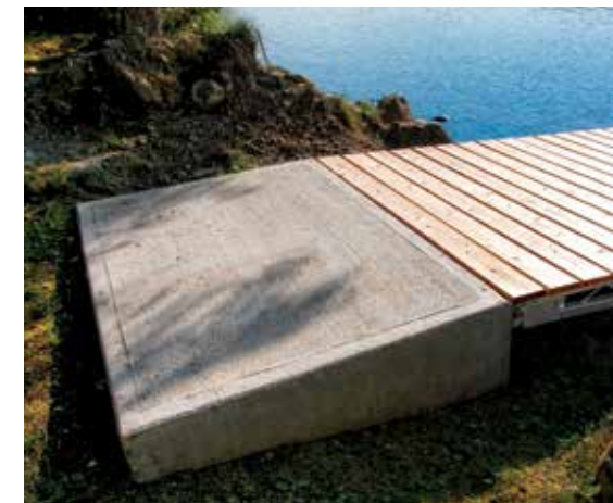
Above Top: Straight articulating dock with cedar decking. Above Left and Right: Concrete pad being formed then shown completed to serve as the shore hitch for an articulating dock.
