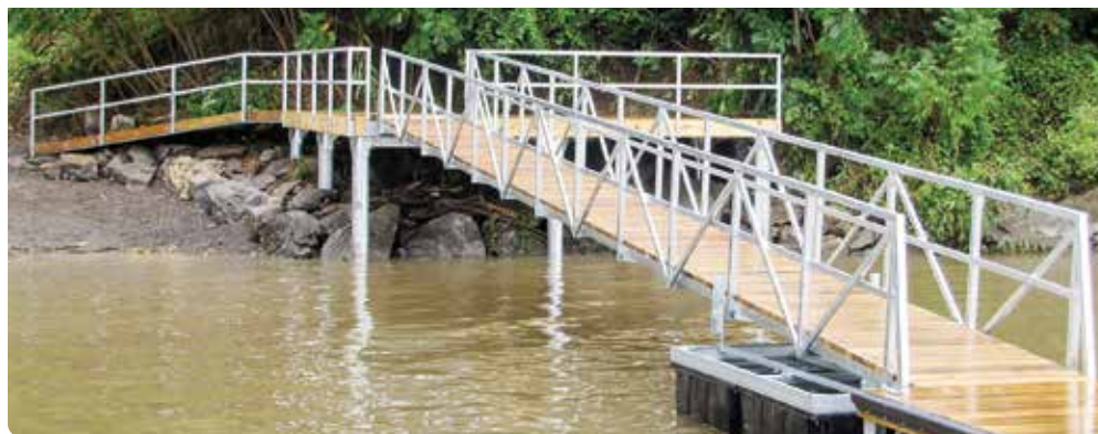
Above: Shoreside platform used for shore attachment system.
