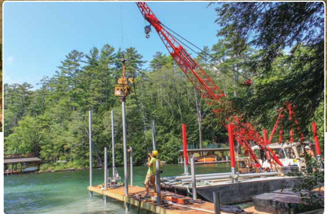
One of our crews installing a pile dock.
