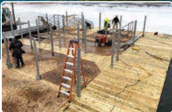
Inset: Multi-slip pile dock foundation in place – crew prepping to build boathouse.
