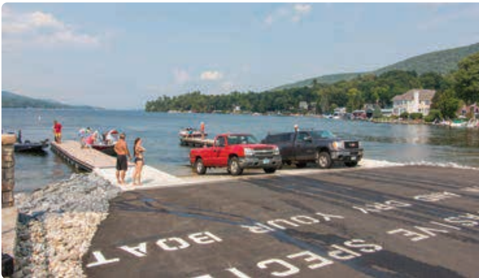
Commercial steel truss floating docks with black powder coated finish for public boat access launch at the Village of Lake George, NY
