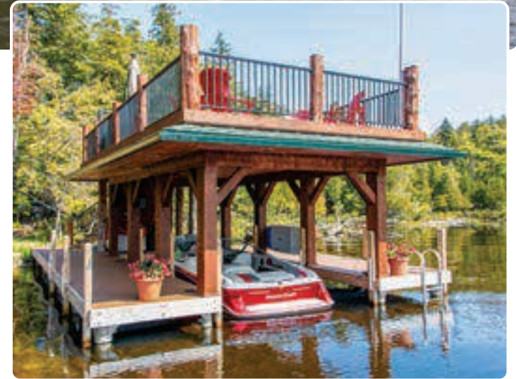
Top: Pile dock foundation by The Dock Doctors with vertical columns in place for sundeck structure.
