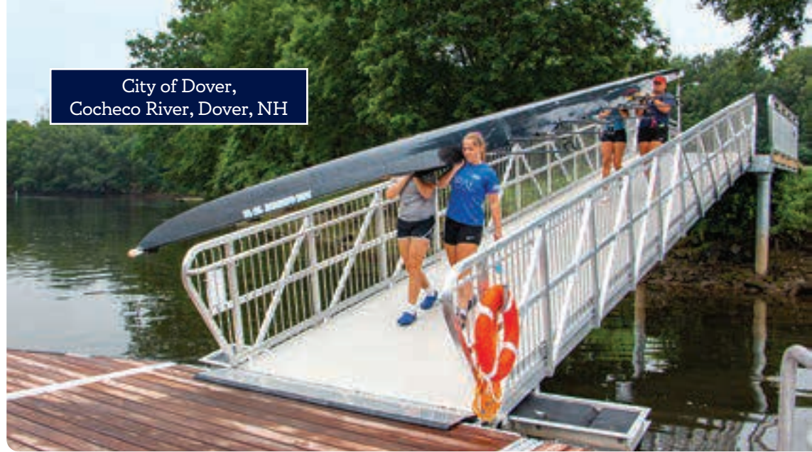
7' wide gangway designed to accommodate rowing sculls.
