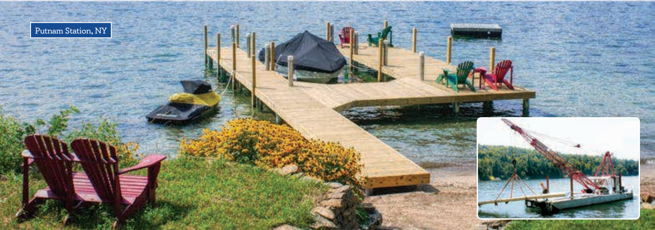
Above Left: Pile dock with pilings above the deck surface. Inset: One of our workboats "Doc" transporting a pile dock section.
