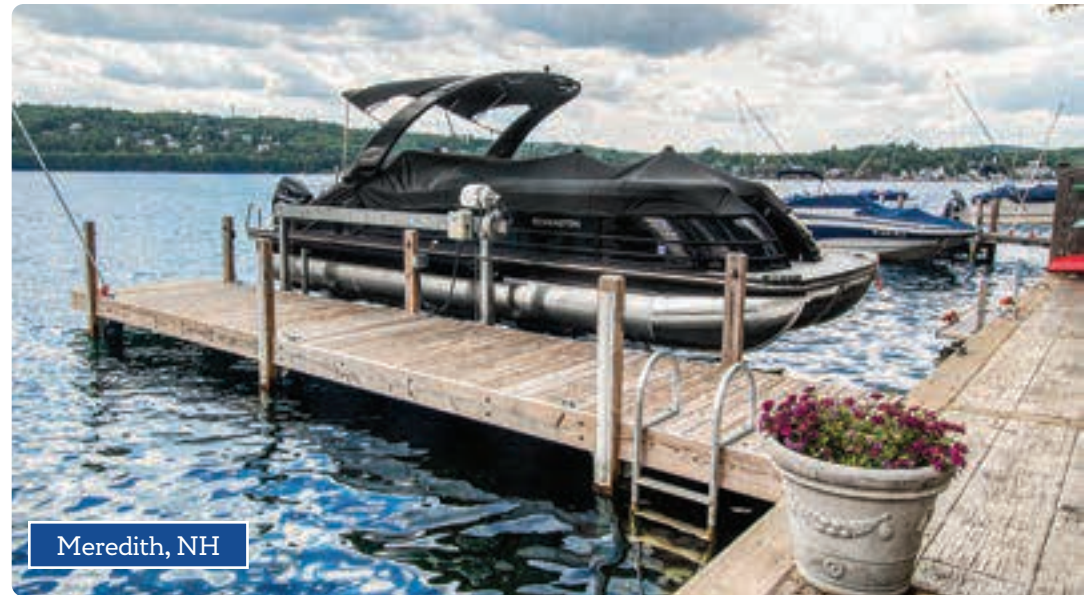
Above: Pile dock with rub strakes attached to a concrete seawall.
