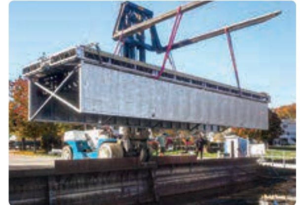
Wave attenuator being installed.
