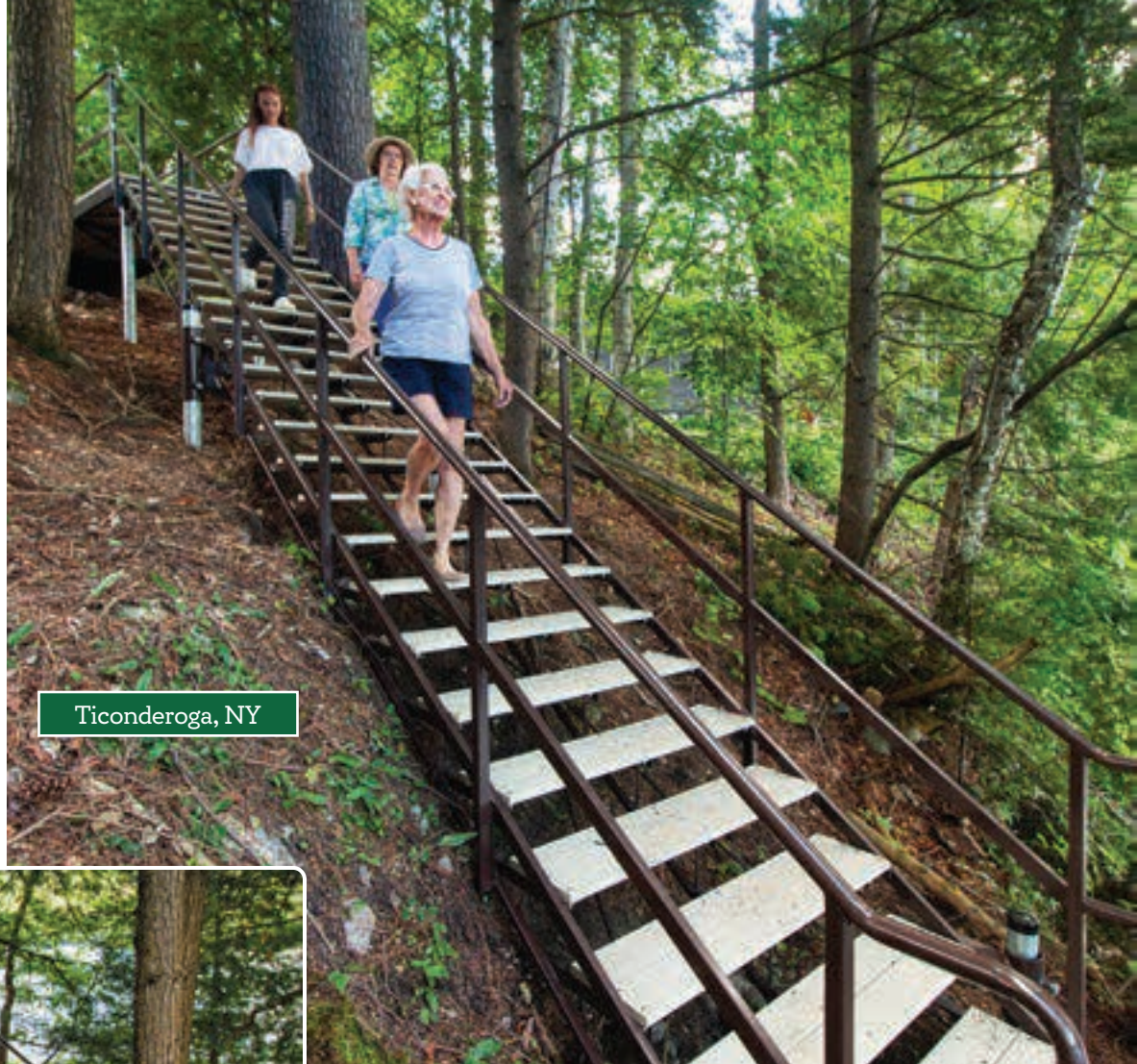
Above: Brown powder coated stairs with composite stair treads.
