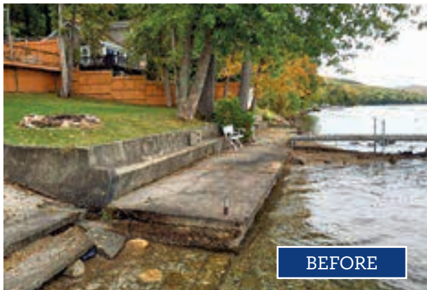
Above: 100' long concrete seawall and patio repair on Lake George, including a new concrete boat ramp and stairs.
