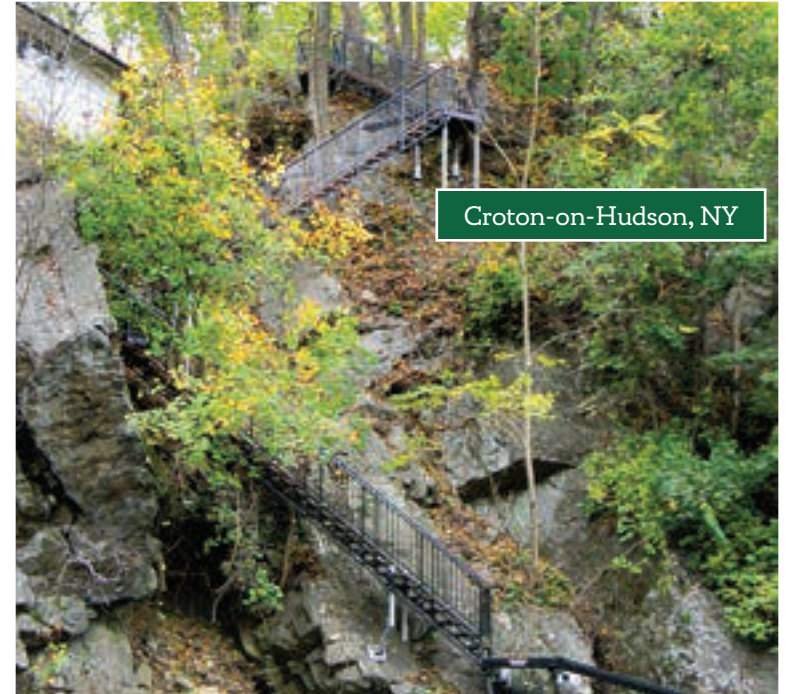
Free span stairs with black powder coating and Ipe treads traversing a vertical drop of approximately 60 feet.
