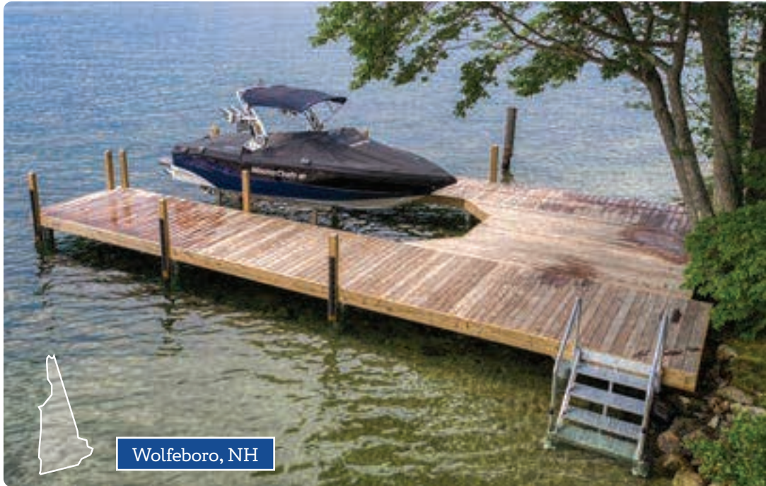
Above: Pile dock with single angled boat slip, Ipe decking and custom swim stairs.
