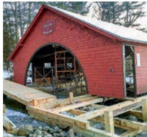
Boathouse stabilized with a new foundation – located at a recognized facility on Lake George.
