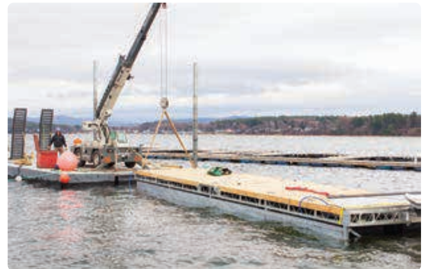
Transporting an attenuator section to installation location.
