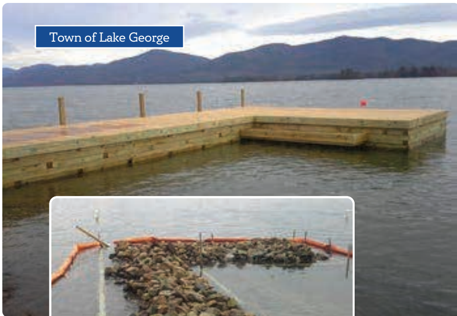
Crib dock replacement in progress
