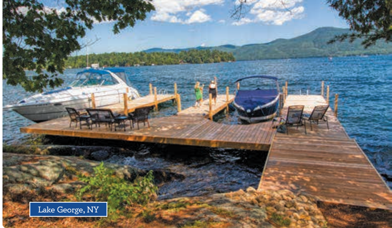
Above: Pile dock with Ipe decking, rub strakes and two “angled” boat slips.
