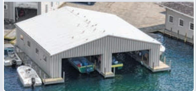
Above: Fabricated and installed an industrial pile support structure with deep water bracing and erected metal building for NYSDEC Green Island Boat Facility.
