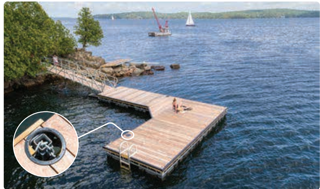
Steel truss floating dock with Ipe decking. Inset: Example of internal mounted anchor chain tube - shown with deck access plate removed.
