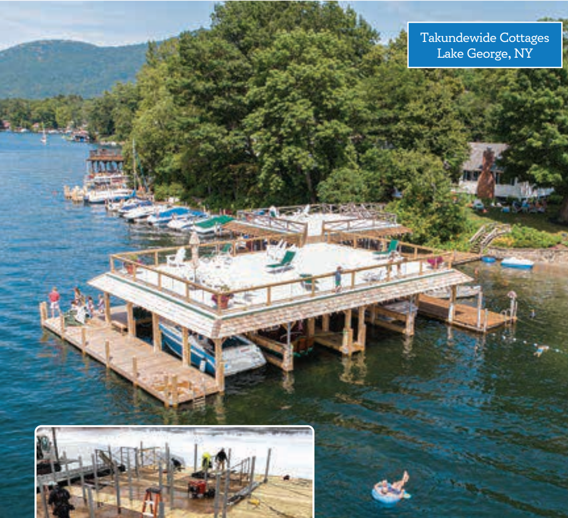
Inset: Multi-slip pile dock foundation in place – crew prepping to build boathouse.
