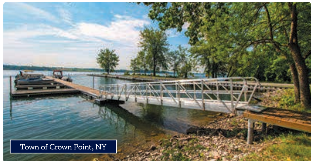
Below Right: Our permanent pile platform with shore hitch to connect gangway to the heavy duty aluminum floating dock system.
