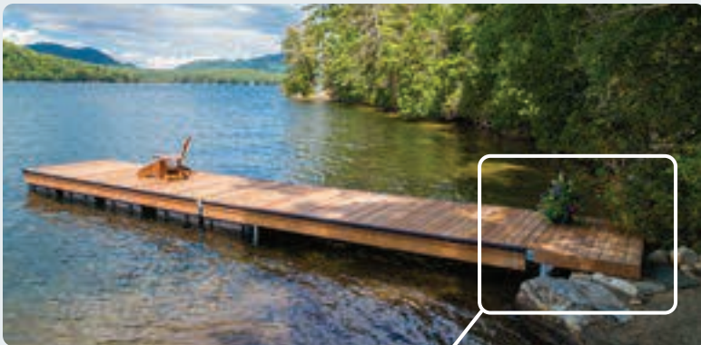
Permanent pile platform shore hitch.
