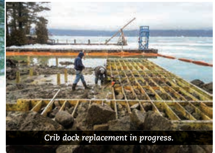
Cribs being moved into place.
