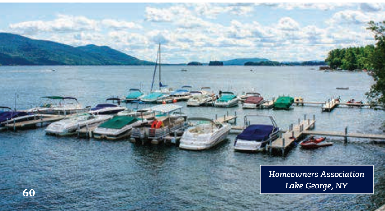
Commercial association pile dock designed for a deep water site with 12" mono piles on ends of the dock fingers with linking underwater truss for stability.
