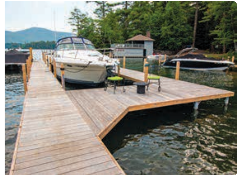
Above Left: U-shaped pile dock with Ipe hardwood decking. Above Right: Angled corner for more deck space and a wider walkway.
