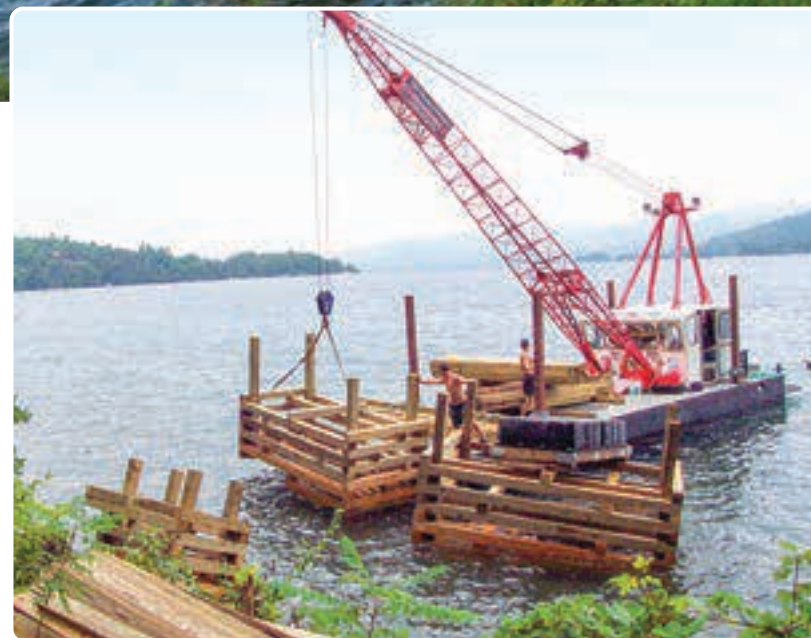
New cribs being moved into position.
