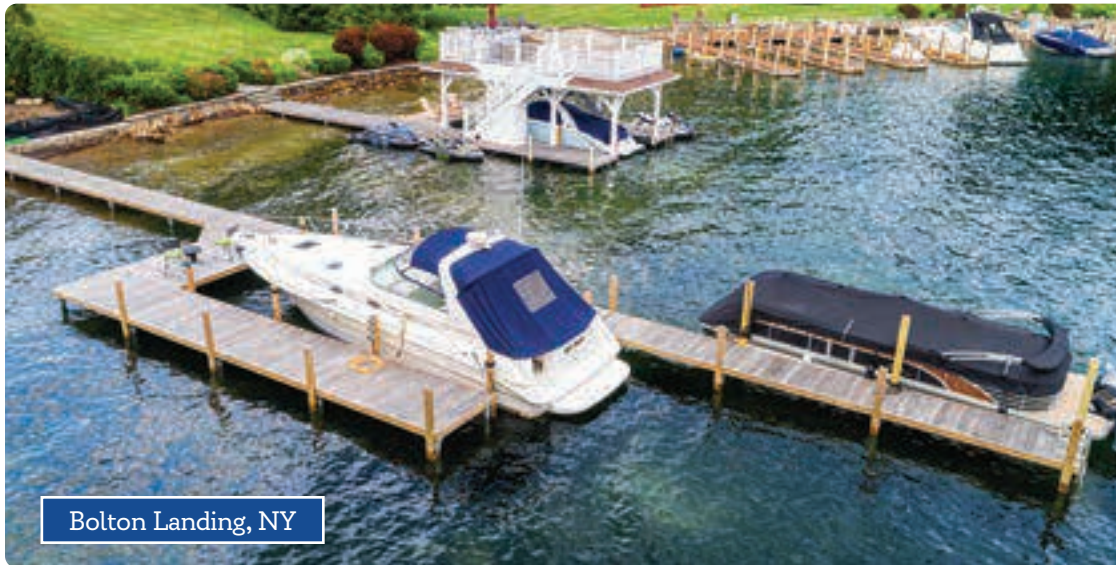
Above Left: U-shaped pile dock with Ipe hardwood decking. Above Right: Angled corner for more deck space and a wider walkway.
