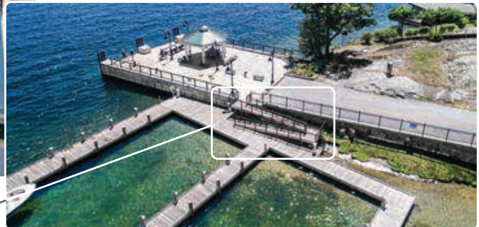
ADA access ramp transitions from the upper pier area to our commercial pile dock.
