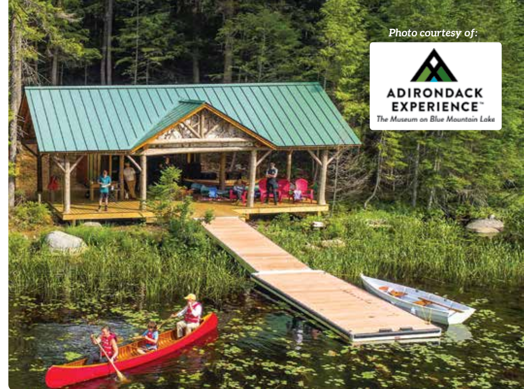
10' x 16' paddle dock and 8' x 16' ramp section with Ipe decking.
