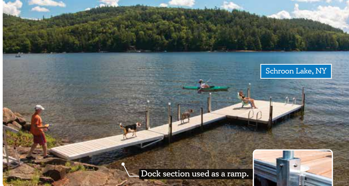
Above: Aluminum floating dock with WearDeck composite decking and solar post lites (see p. 16). 4' x 12' dock section used as a ramp.
