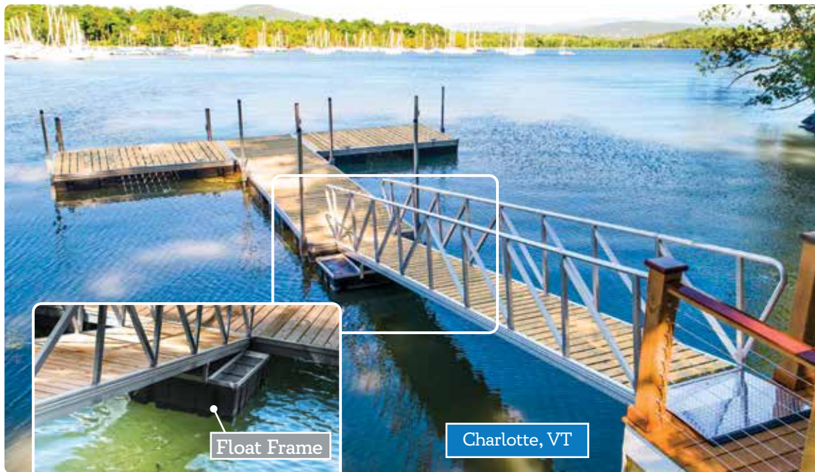
Above: Aluminum floating dock and 3' x 24' aluminum gangway with cedar decking.
