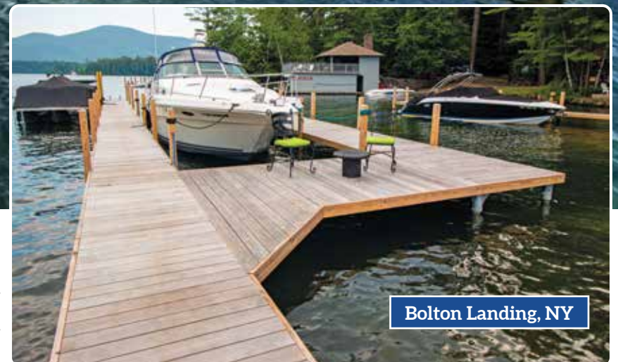
Above: U-shaped pile dock with Ipe hardwood decking. Right Inset: Angled corner for more deck space and a wider walkway.
