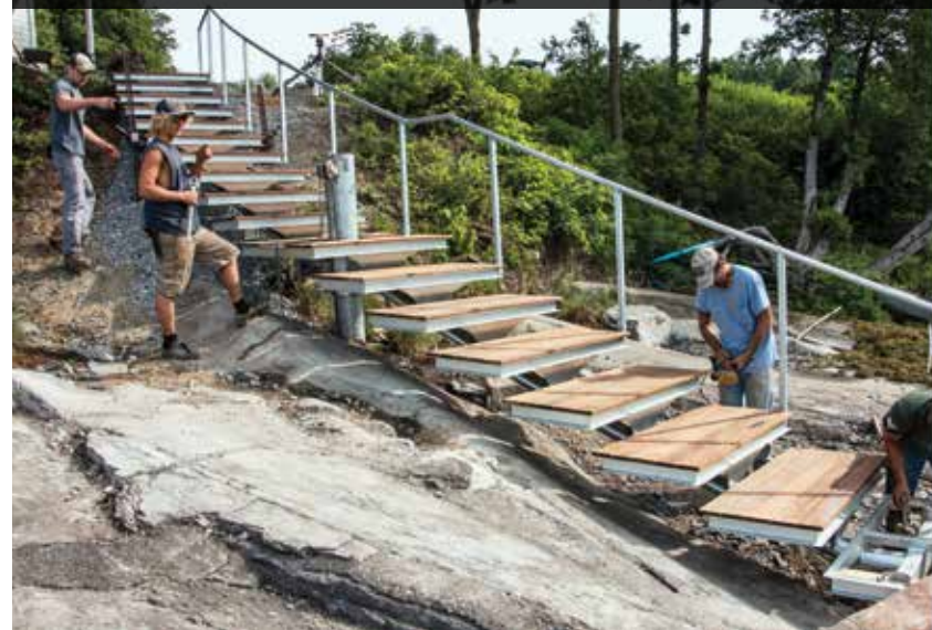
Curved mono-beam stairway during installation
