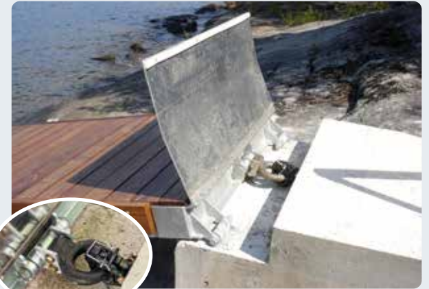
Concrete hitch pad with aluminum tread plate and pintle hitch.
