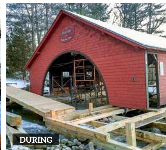
Above: New pile dock foundation installed. Above Right "During": Boathouse lifted with original crib dock foundation removed.
