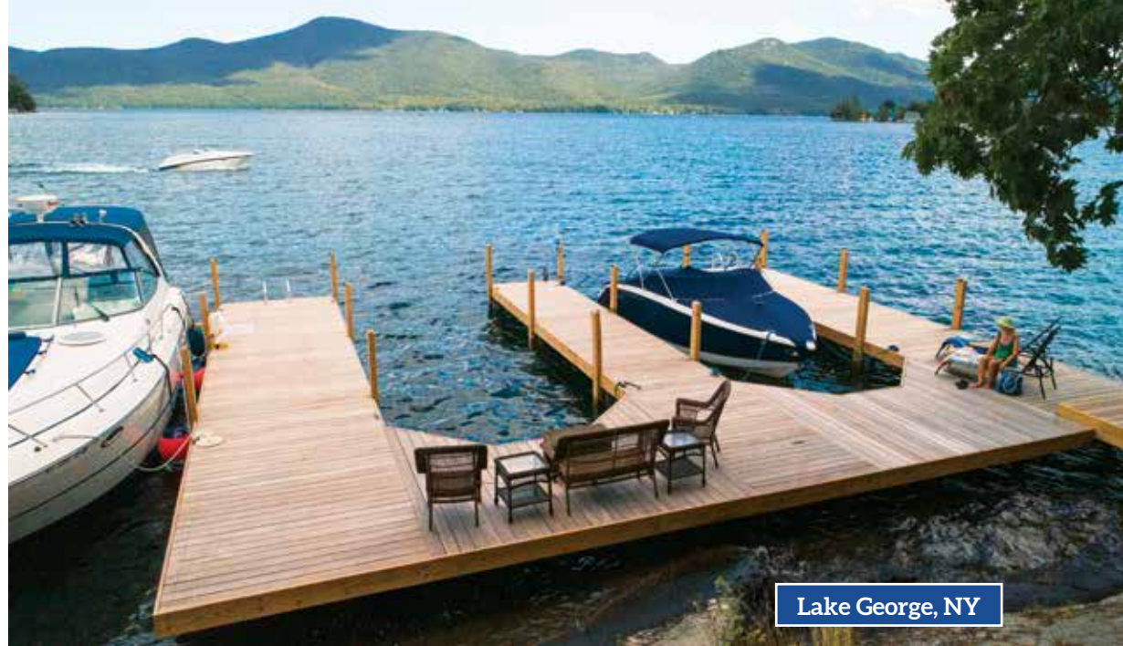
Above: Pile dock with Ipe decking, rub strakes and two “angled” boat slips.
