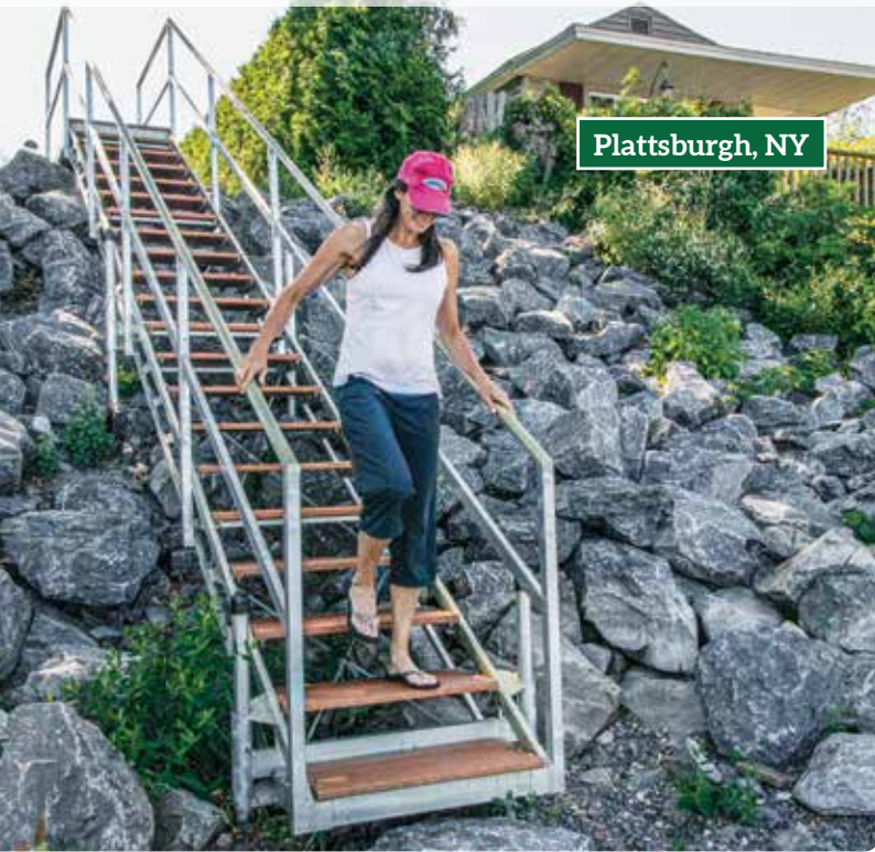
Above: Stair system to traverse a rocky shoreline.
