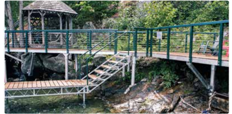
Shore connection for articulating style dock
