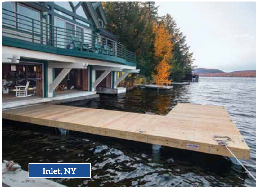
Above: L-shaped pile dock attached to an existing boathouse.
