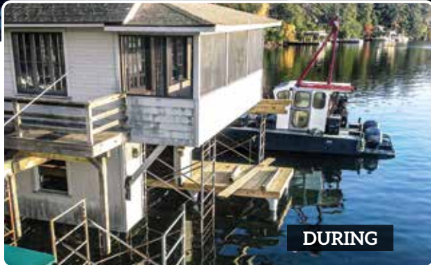
Above: New pile dock foundation installed. Inset: Boathouse lifted with original crib dock foundation removed.
