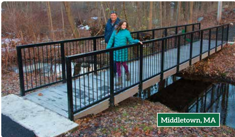
Pedestrian bridge with black powder coated railings.
