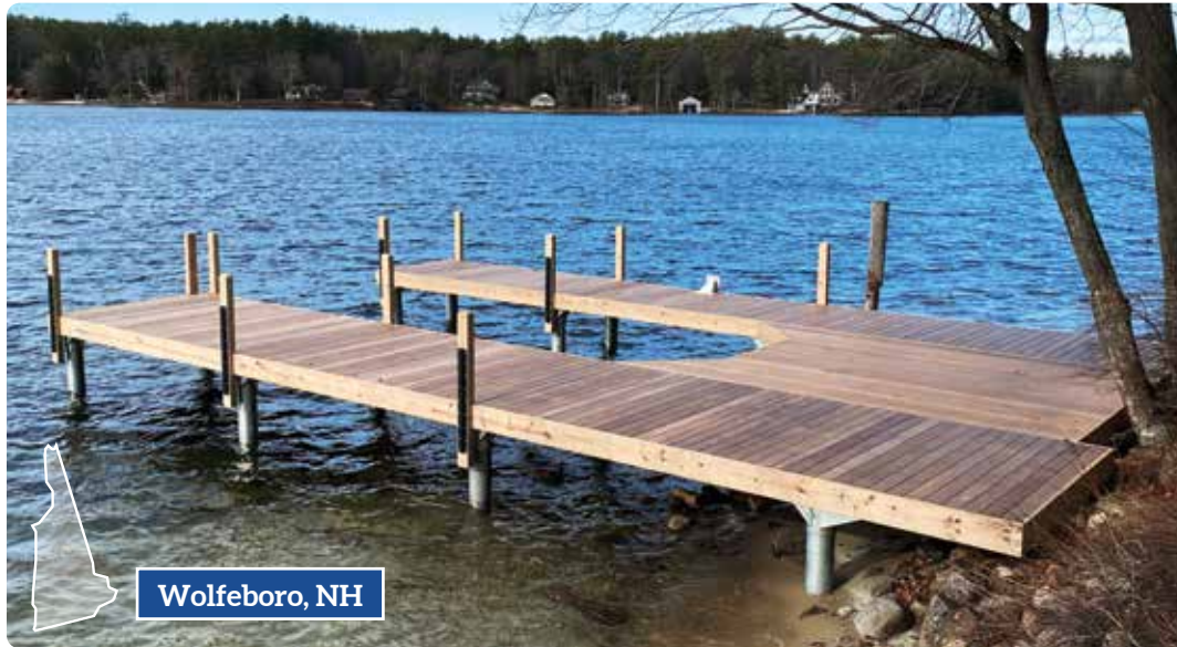
Above: Pile dock with single boat slip and Ipe decking.
