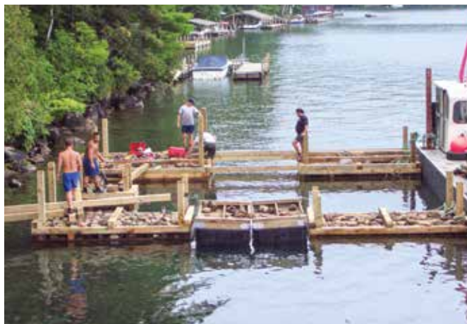
Crib dock in progress.
