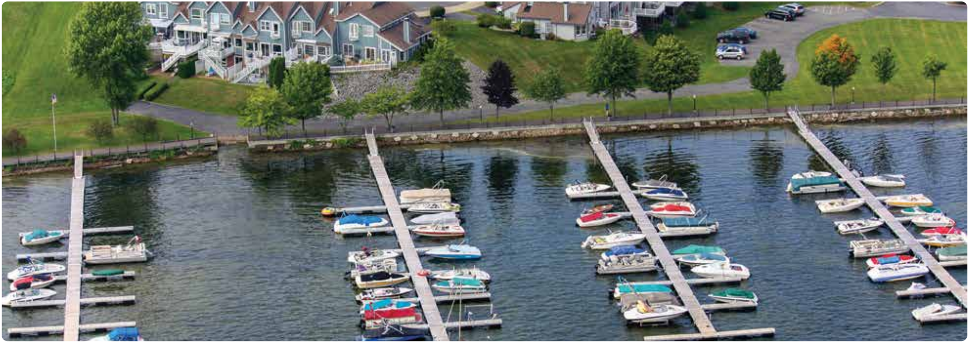
Association dock system using our heavy duty aluminum floating docks.
