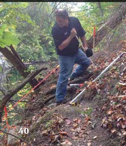
Measuring for a new stair system.
