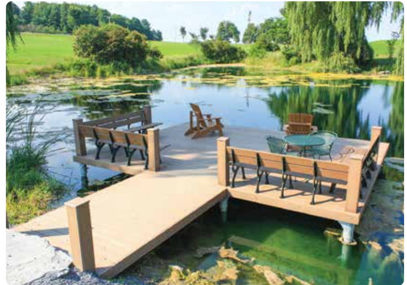
Above: Pile dock on a pond.
