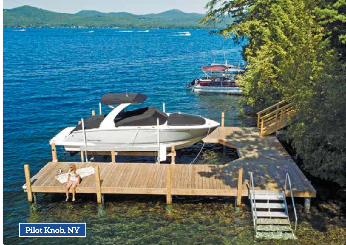
Above: "U-shaped" pile dock with 8" diameter piles and underwater bracing for protection from ice.
