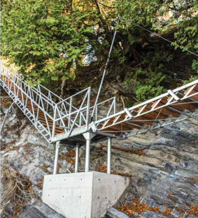
Left: Hinged lower section of the above stairs raised for winter storage using our T-pole and cable lift system.
