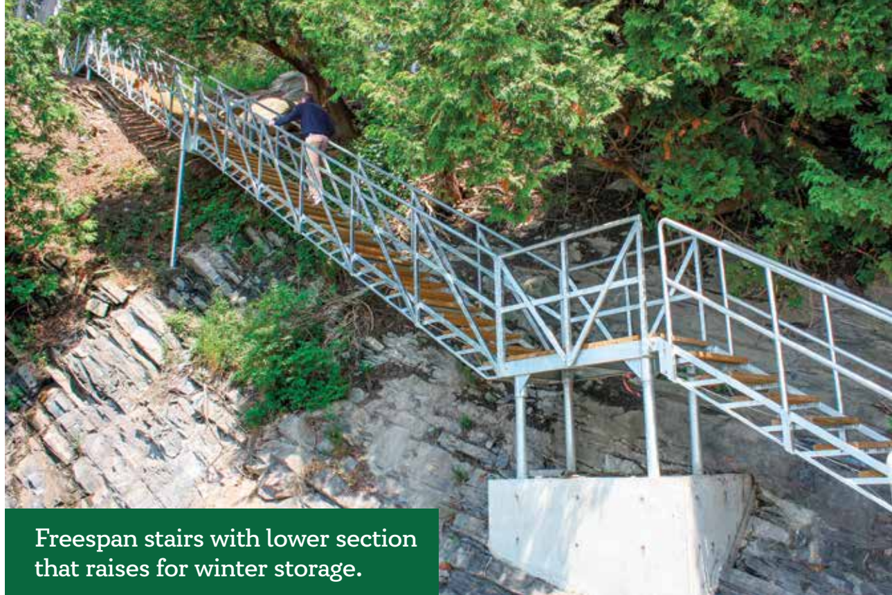
Left: Hinged lower section of the above stairs raised for winter storage using our T-pole and cable lift system.
