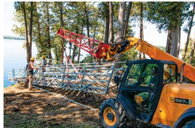
Stairs being installed.
