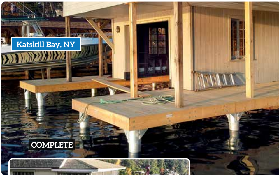
Above: New pile dock foundation installed. Inset: Boathouse lifted with original crib dock foundation removed.
