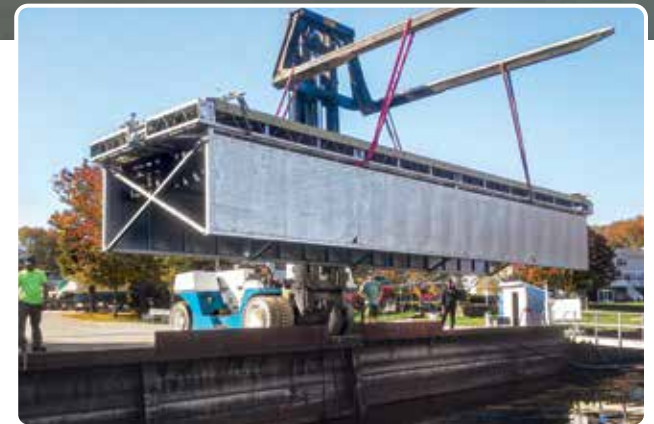
Wave attenuator being installed.
