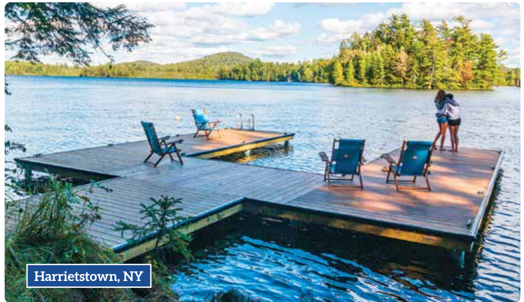
Above: U-shaped pile dock with Ipe decking and vinyl edge fender. The pilings are cut below deck surface.
