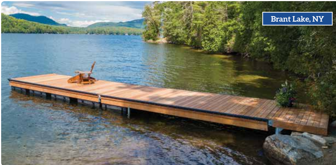
Straight floating dock with Ipe hardwood decking, vinyl edge fender and truss skirt board to camouflage the frame. Our pile platform is used as a shoreside hitch.
