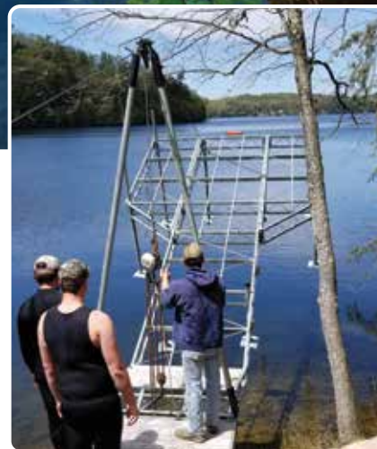
Above: Articulating dock with our shoreside pile platform used as shore mount.
