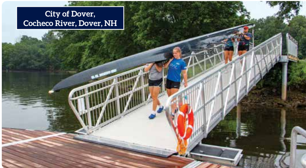
7' wide gangway designed to accommodate rowing sculls.
