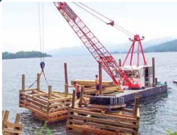
New cribs being moved into position.
