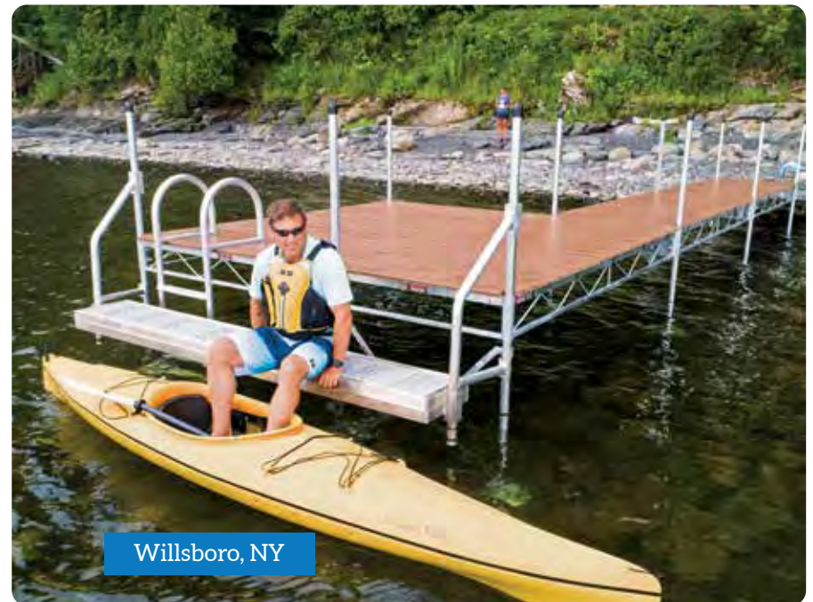
Steel truss leg docks with composite decking and our lower access platform (see page 9).
