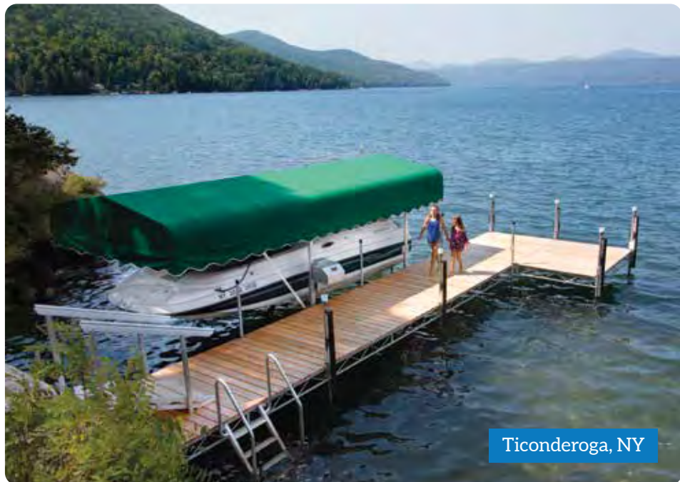
Steel truss leg docks with 6' wide sections, cedar decking, and 5,000 lb. vertical boat lift with Sunbrella Canopy.
