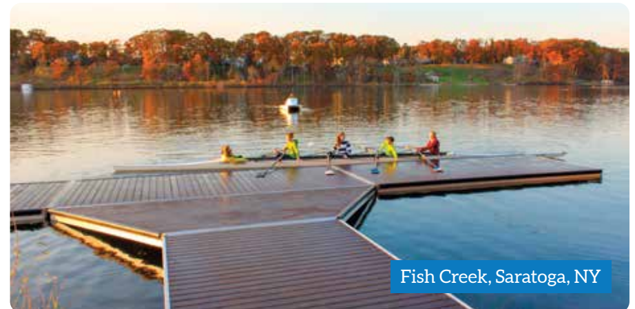
Heavy duty aluminum frame rowing docks with composite decking.
