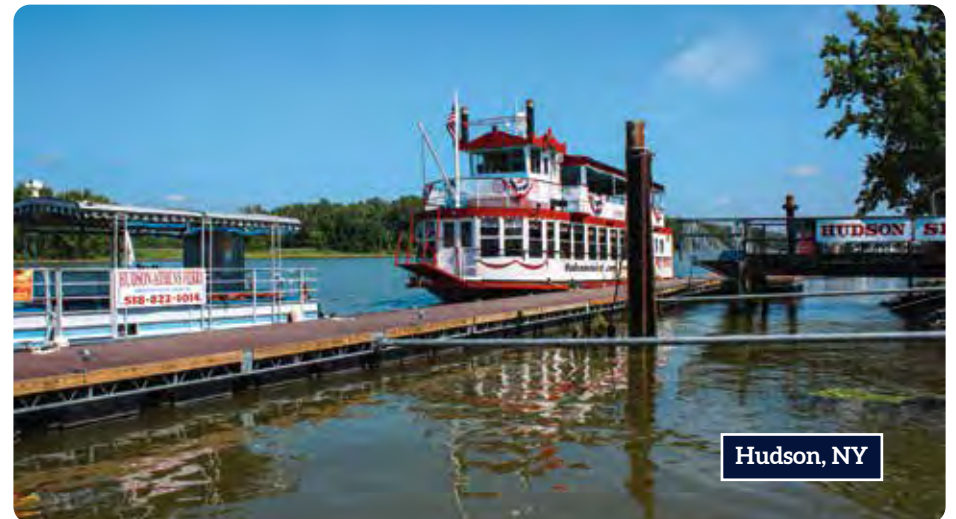
Below: Commercial steel truss floating docks for tour boats at a municipal park.
