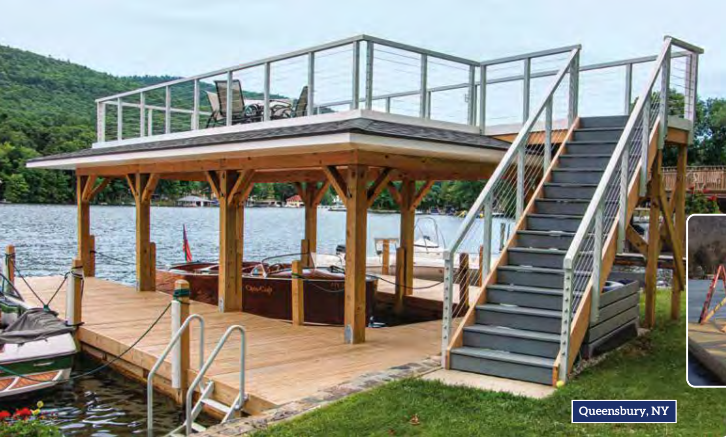
Above: Completed boathouse with crib dock foundation and sundeck.
