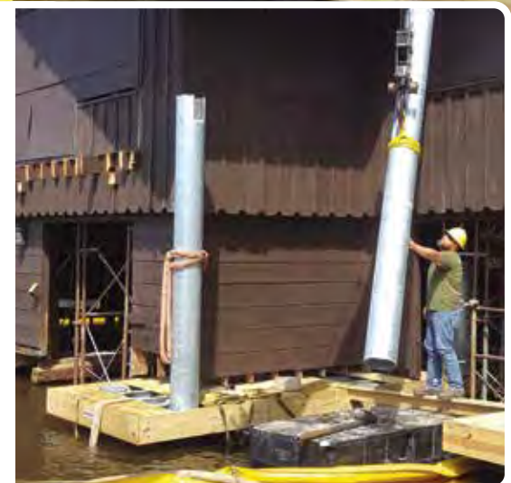
Piles being placed for the new pile dock foundation.
