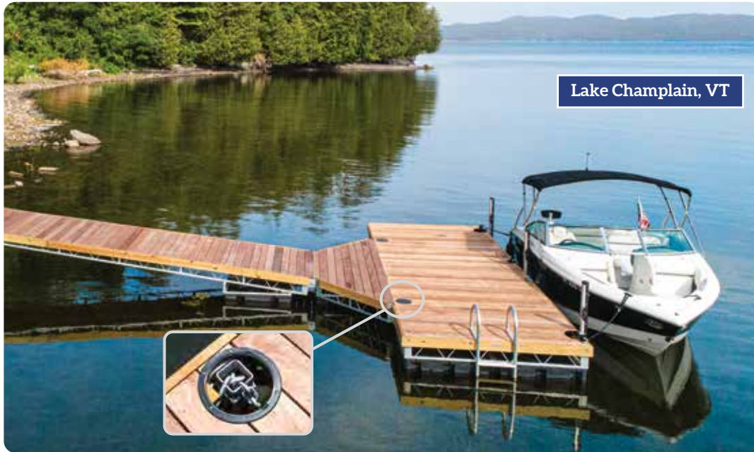
Steel truss floating dock with Ipe decking. Inset: Internal mounted anchor chain tube – shown with deck access plate removed.
