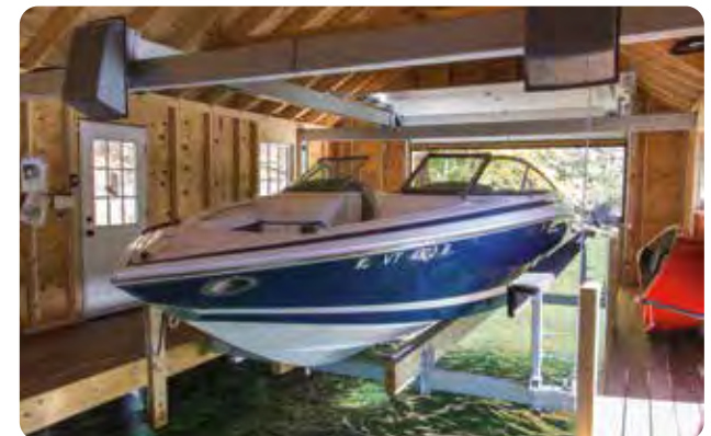
Boathouse lift installed in a boathouse. See custom boat lift section pages 30-31.
