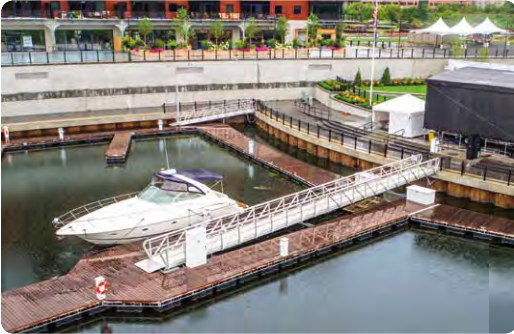
5' x 80' ADA compliant commercial aluminum gangway.
