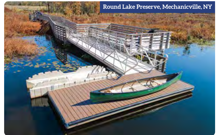
Heavy duty aluminum floating dock with composite decking and aluminum gangway with aluminum decking.
