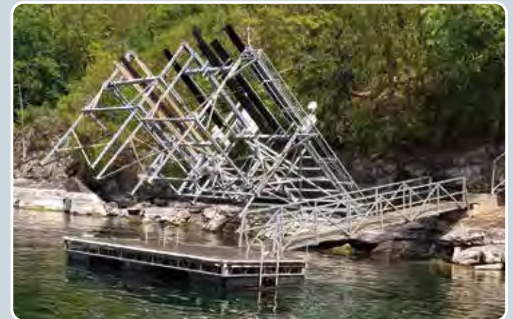
Our Ultimate Boat Lift customized with galvanized lift arms attached to the shore, which allow it to be raised for winter storage.
