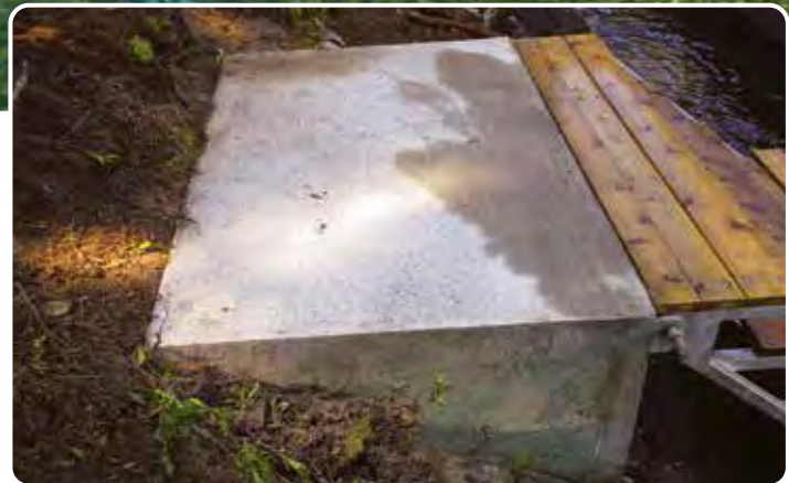
Above Top: Articulating dock with vertical fenders and Hydraulic Boat Lift. Above Bottom: A concrete pad serves as the shore hitch for the above articulating dock.
