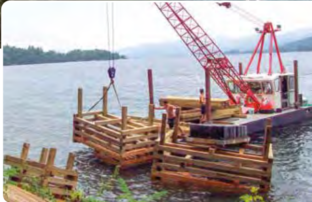
New cribs being moved into position.
