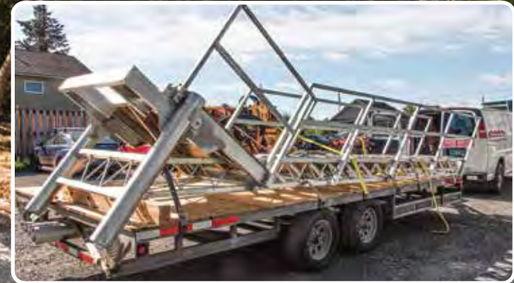
Stairs loaded for delivery and installation.
