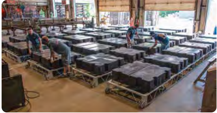
Installation of floats onto galvanized dock frames.
