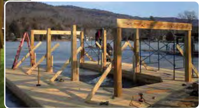
Cribs completed and boathouse structure in progress.
