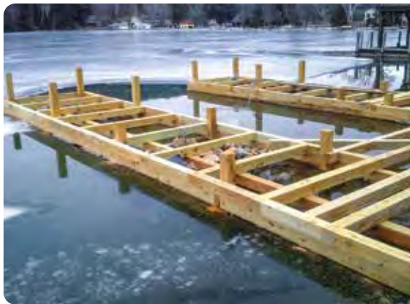
Left: New crib dock being constructed. Middle: Ready for boathouse roof structure. Right: Boathouse sundeck style roof complete.
