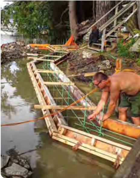
Left: Forms for seawall footings being constructed. Middle: Base of seawall complete. Right: Seawall complete with decorative caps.
