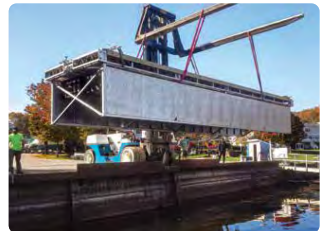
Wave attenuator being installed.
