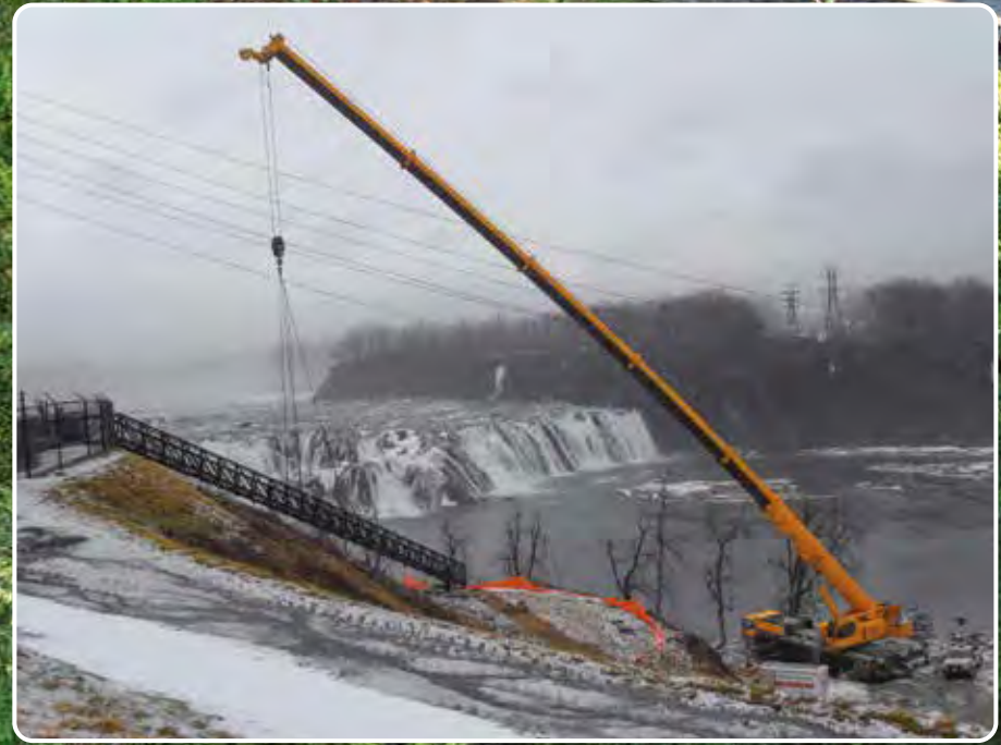
112' long industrial free span stairs for a hydro-power plant.
