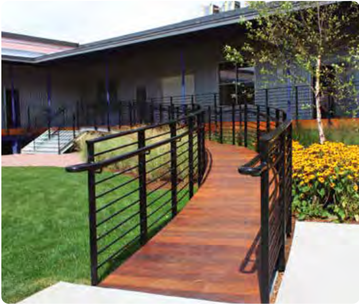
Above: ADA commercial grade galvanized steel curved ramp with Ipe decking & powder coated rails.
