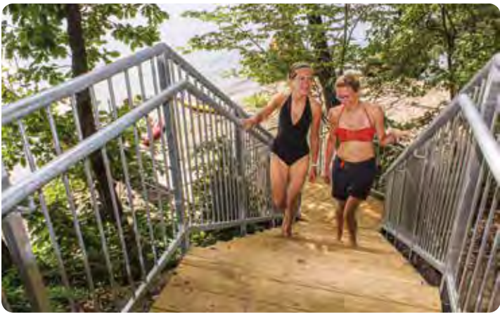
Above: Commercial galvanized steel stairs with pressure treated treads and spindle rails for a children's summer camp.
