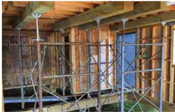
Left: Lifting and supporting the boathouse structure prior to foundation removal and replacement. Right: Installation of new pile dock foundation.
