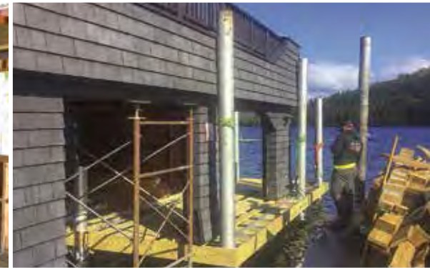
Left: Lifting and supporting the boathouse structure prior to foundation removal and replacement. Right: Installation of new pile dock foundation.
