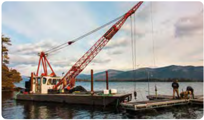
Installation with our workboat "Doc".
