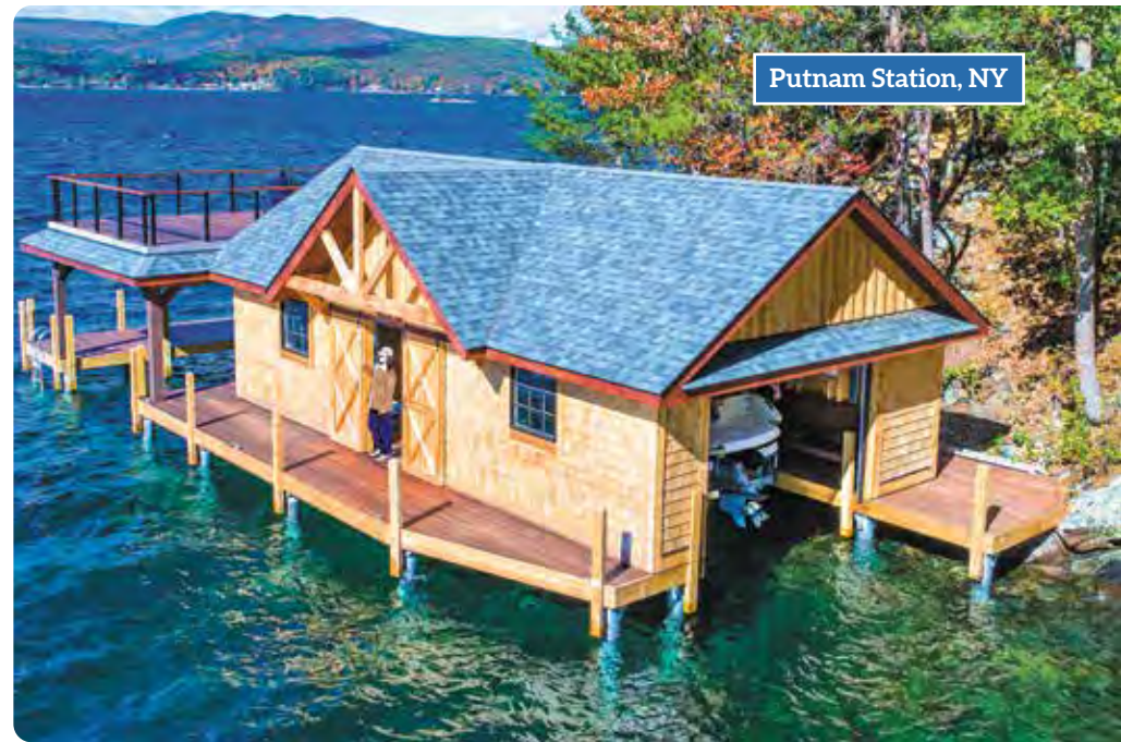
Pile dock foundation with enclosed boathouse and sundeck-style roof with stainless steel cable rails.
