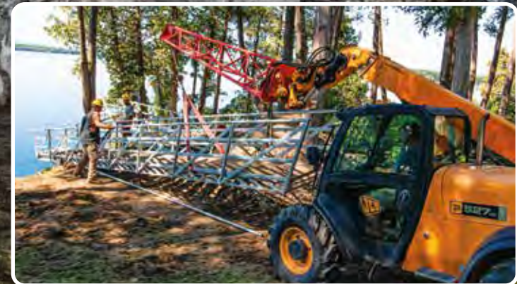
Stairs being installed.
