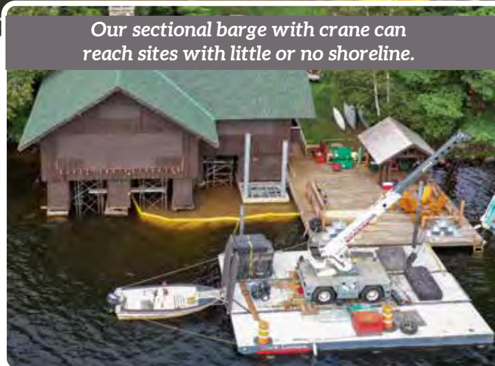
Lifting and supporting the boathouse structure prior to foundation removal and replacement.
