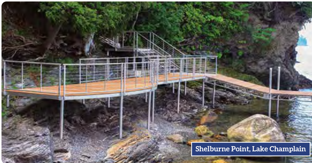
Curved shoreside platform with stainless steel cable rails.
