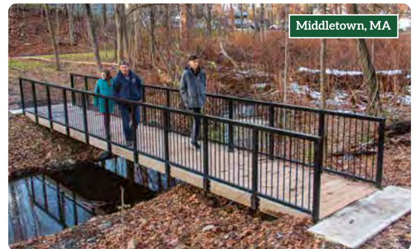
Pedestrian bridge with black powder coated railings.
