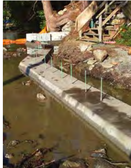
Left: Forms for seawall footings being constructed. Middle: Base of seawall complete. Right: Seawall complete with decorative caps.
