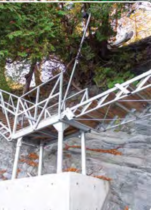
Left: Hinged lower section of the above stairs raised for winter storage using our T-pole and cable lift system.
