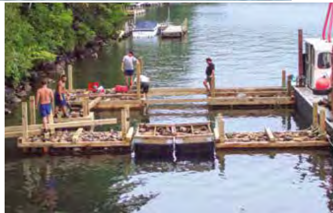
Crib dock in progress.
