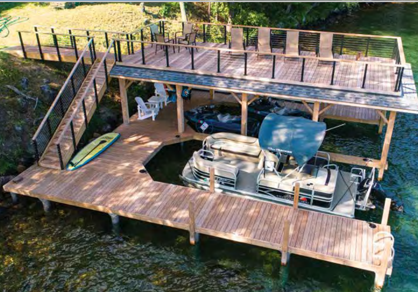
Above: Boathouse complete with “sundeck-style” roof with stainless steel cable rail. Top Right: Piles are driven into the lakebed. Bottom Right: Pile dock foundation complete with a slip divider / catwalk. Vertical columns in place for the sundeck boathouse roof.
