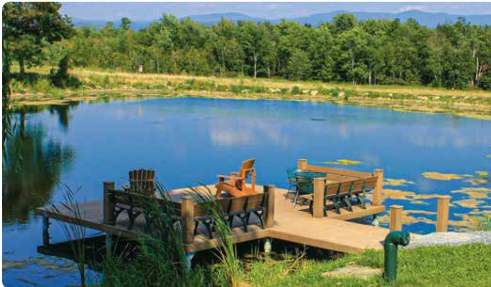
Above: Pile dock on a man made pond.
