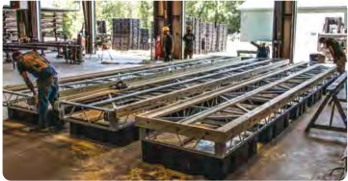
Installation of decking.
