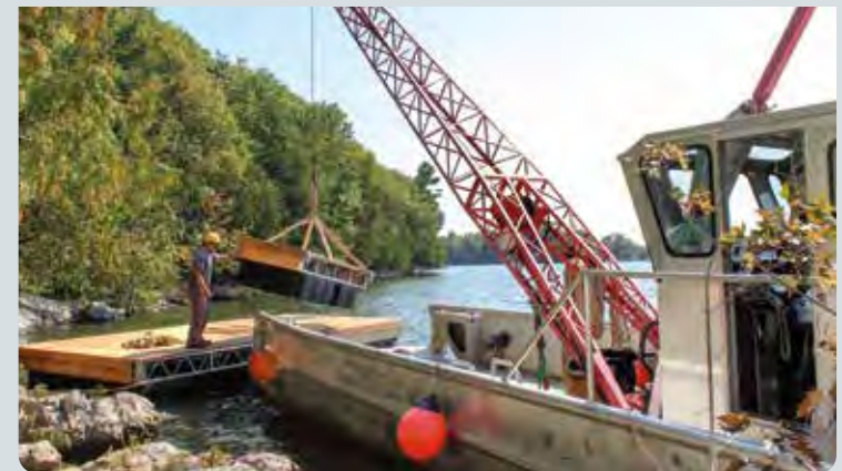
Installation with our workboat.
