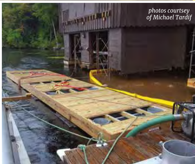
New pile dock section being floated into place.
