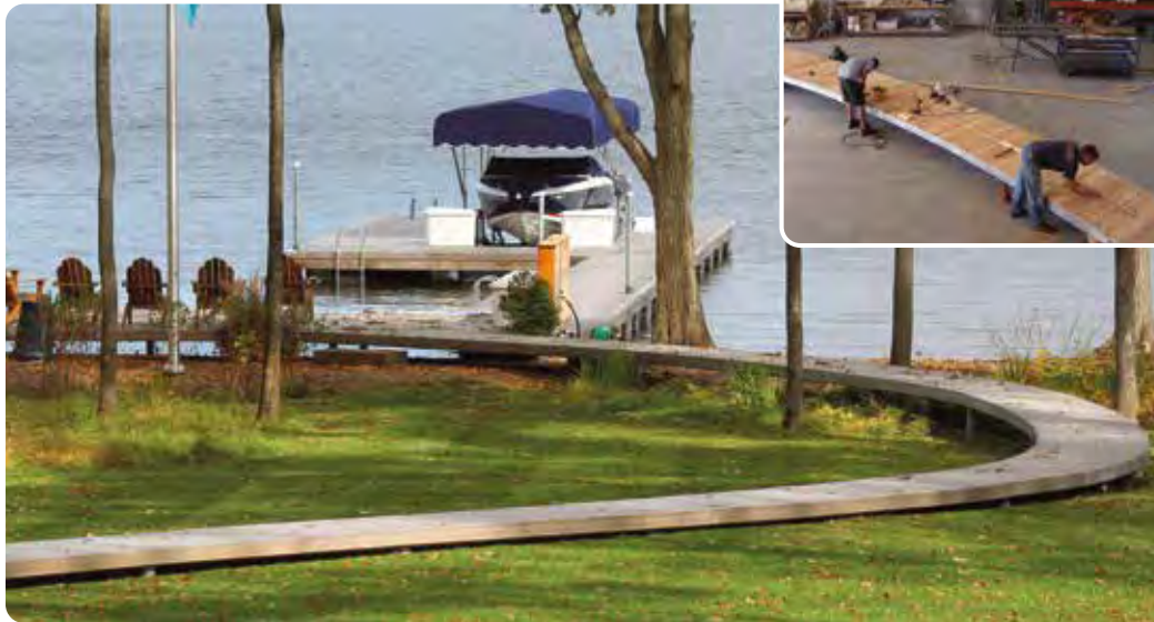
Above: Curved walkway using our galvanized steel permanent pile platform.
