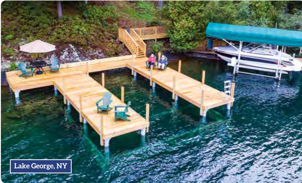
Above: Pile shoreside platform and pile dock with underwater bracing on a site with a steep shoreline.
