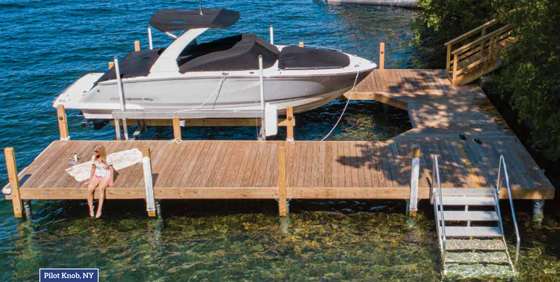
"U-shaped" pile dock with 8" diameter piles and underwater bracing for protection from ice.
