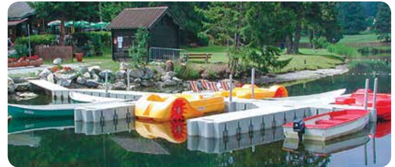
Above: "2000 Series" higher profile system at a state park.
