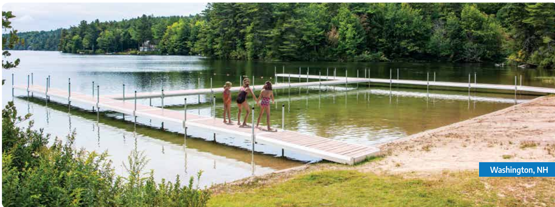
Medium duty aluminum leg docks with NyloDeck® decking at a town beach in Washington, NH.
