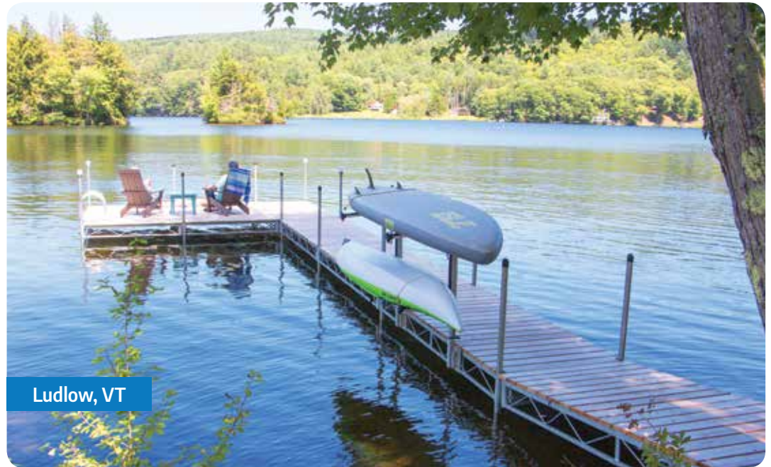
Above: Steel truss leg docks with dock-mounted 2-craft storage rack.
