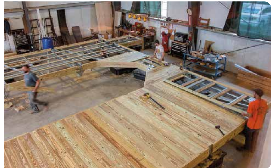
Above: Pile dock in final stages during decking installation.
