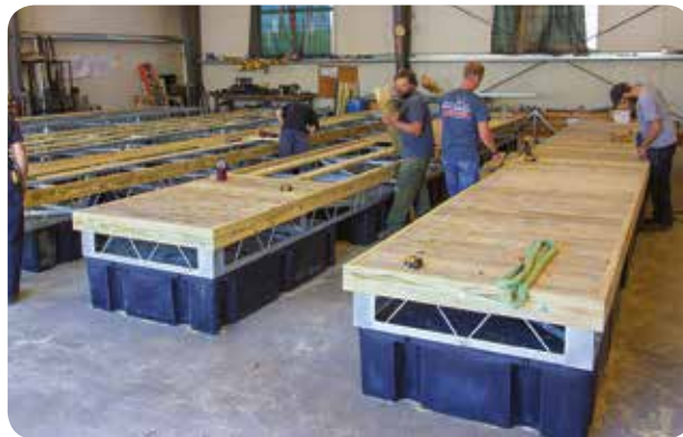
Decking being applied in our workshop.
