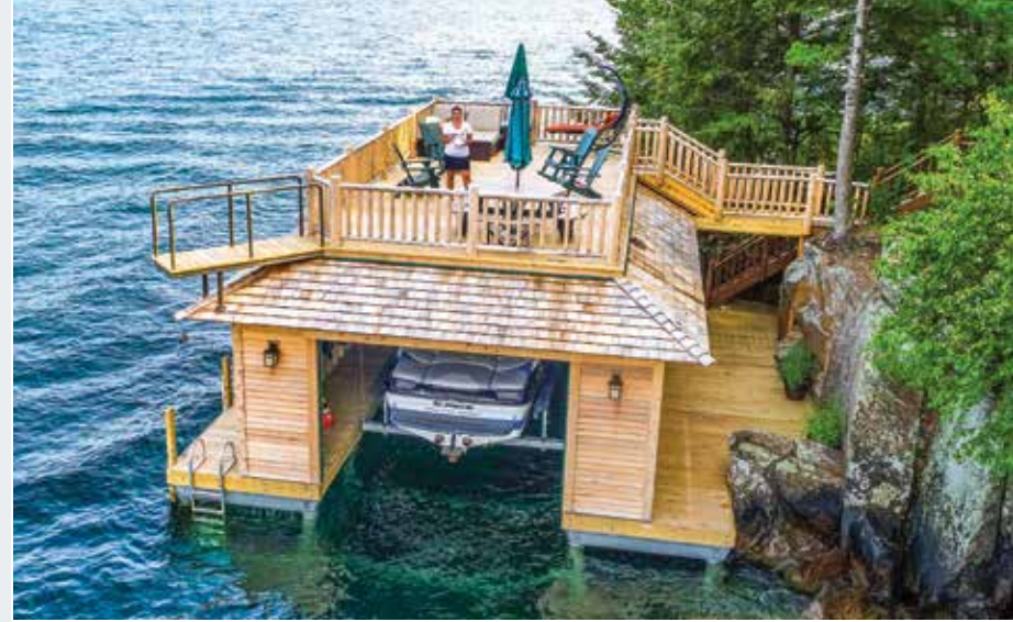
Boathouse lift installed in a boathouse (above).
