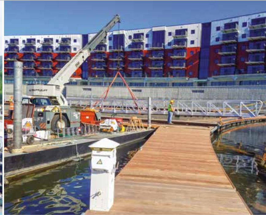
Our sectional barge and crane installing an 80' gangway at Mohawk Harbor.
