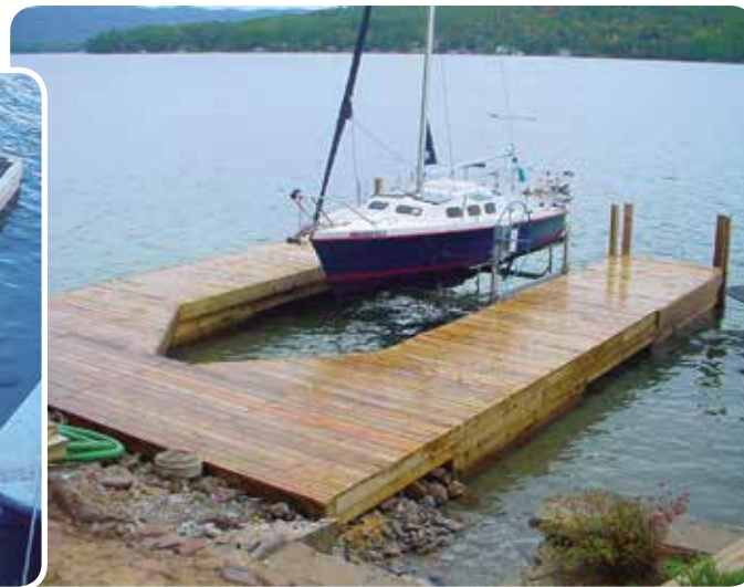
Inset: Crib dock in progress, before final decking installed. Above: Completed crib dock.
