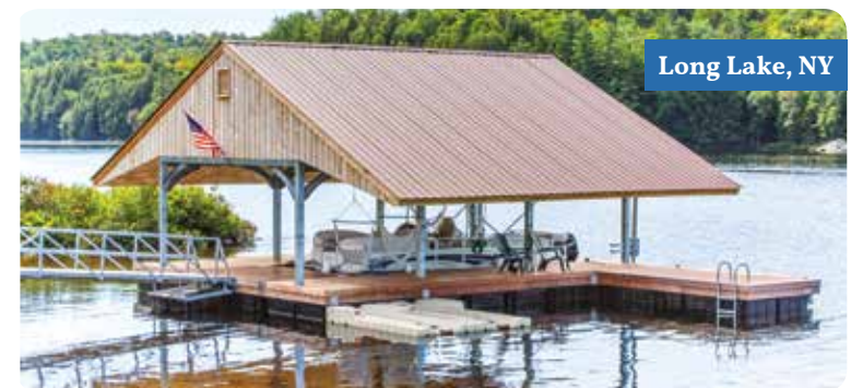
wooden boathouse structure by others
