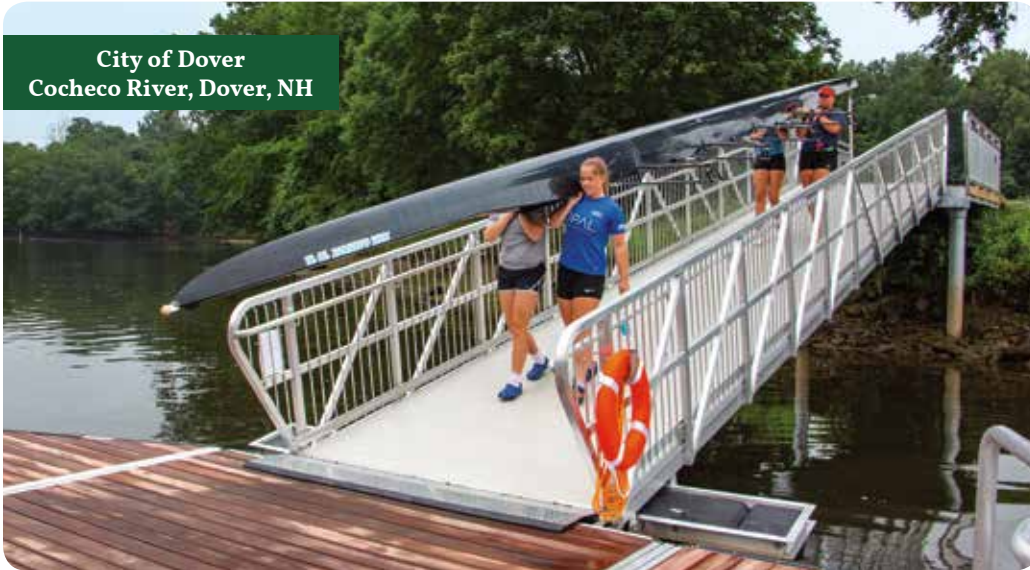
7' wide gangway designed to accommodate rowing sculls.
