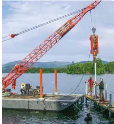
Workboat driving piles.
