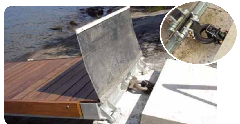
Concrete hitch pad with pintle hitch – aluminum tread plate in raised position.
