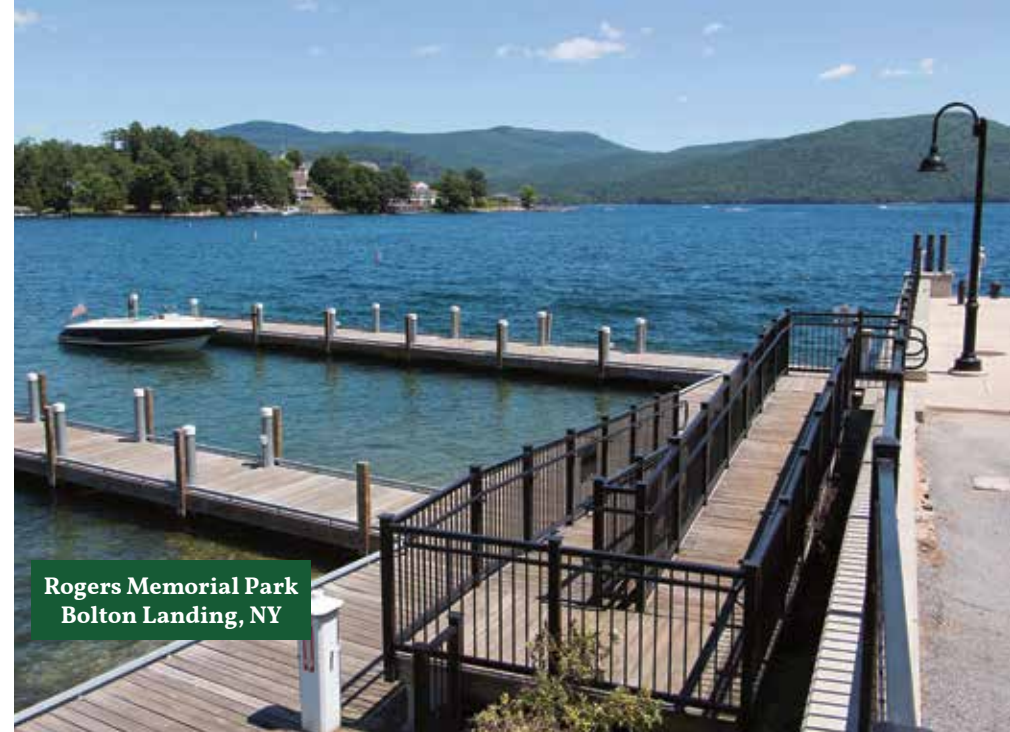
Above: ADA access ramp transitions from the upper pier area to our permanent pile dock at Rogers Memorial Park, Bolton Landing, NY.
