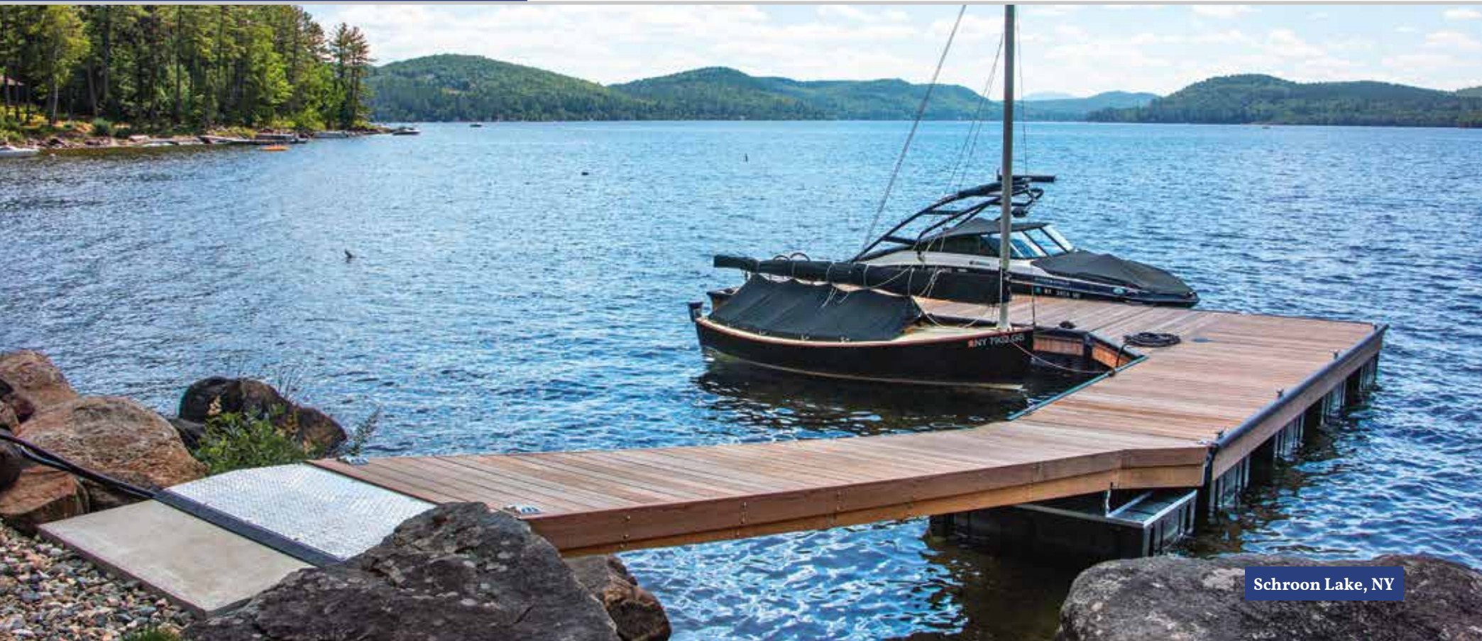
L-shaped floating dock with Ipe decking & truss skirt board to camouflage the frame.
