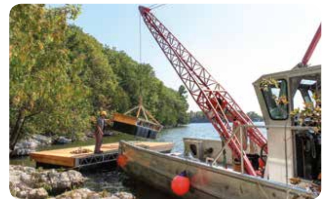
Delivery and installation with our workboat.
