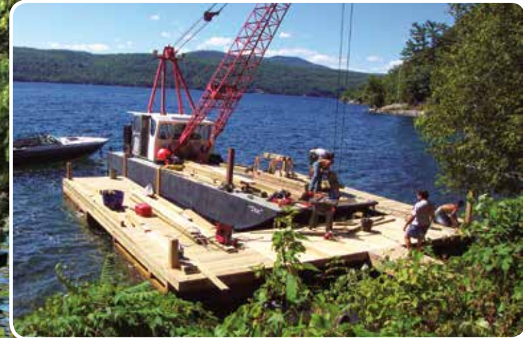
Left: Completed crib dock with rub strakes. Above: During construction with our work boat "Doc".
