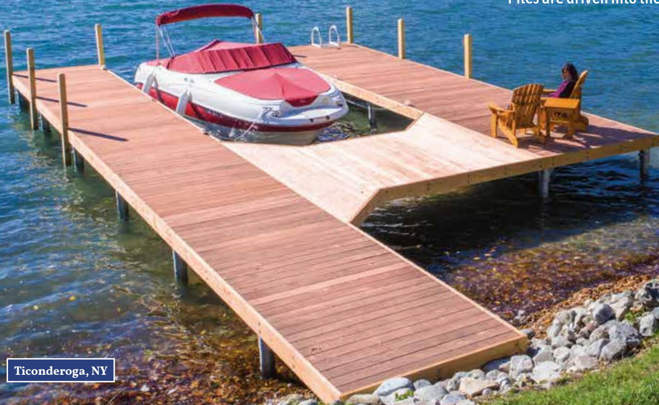
Piles are driven into the lakebed with our workboat and pile driver
