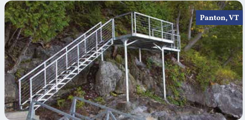
Shore connection system for a custom floating dock
