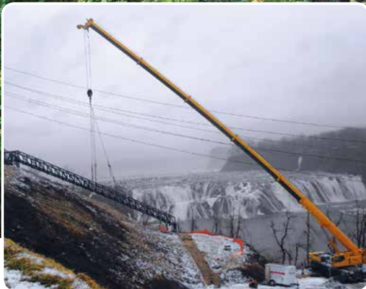
Above: 112' long industrial free span stairs for a hydro-power plant. Inset: Installation of the stairway with a crane.
