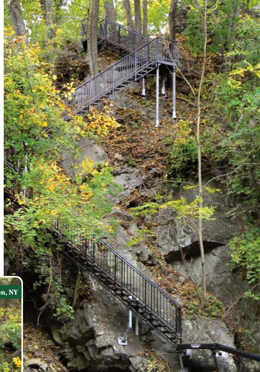
Free span stairs with black powder coating and Ipe treads traversing a vertical drop of approximately 60 feet.
