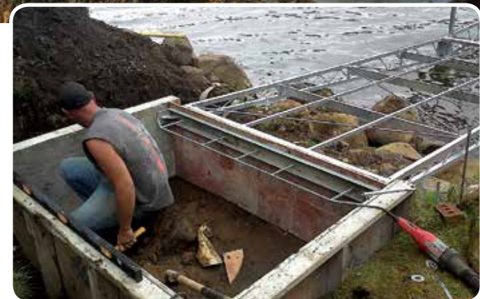
Concrete pad being installed for articulating dock shore connection (above).
