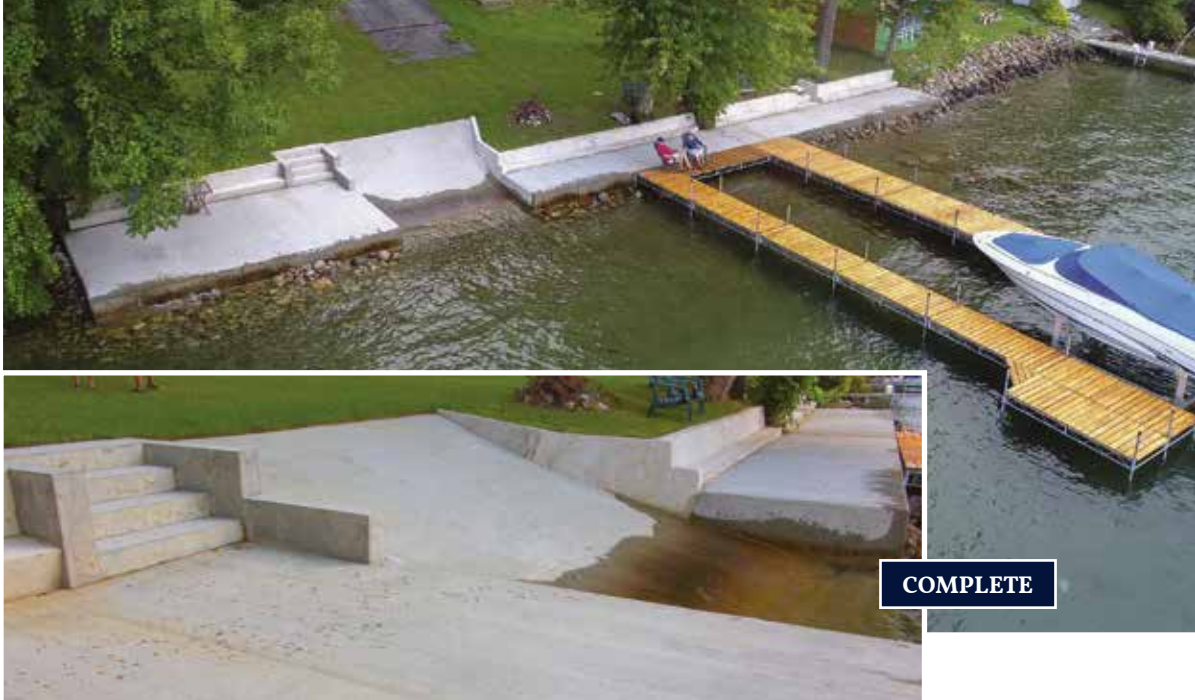
Above: 100' long concrete seawall and patio repair on Lake George, including a new concrete boat ramp and stairs.
