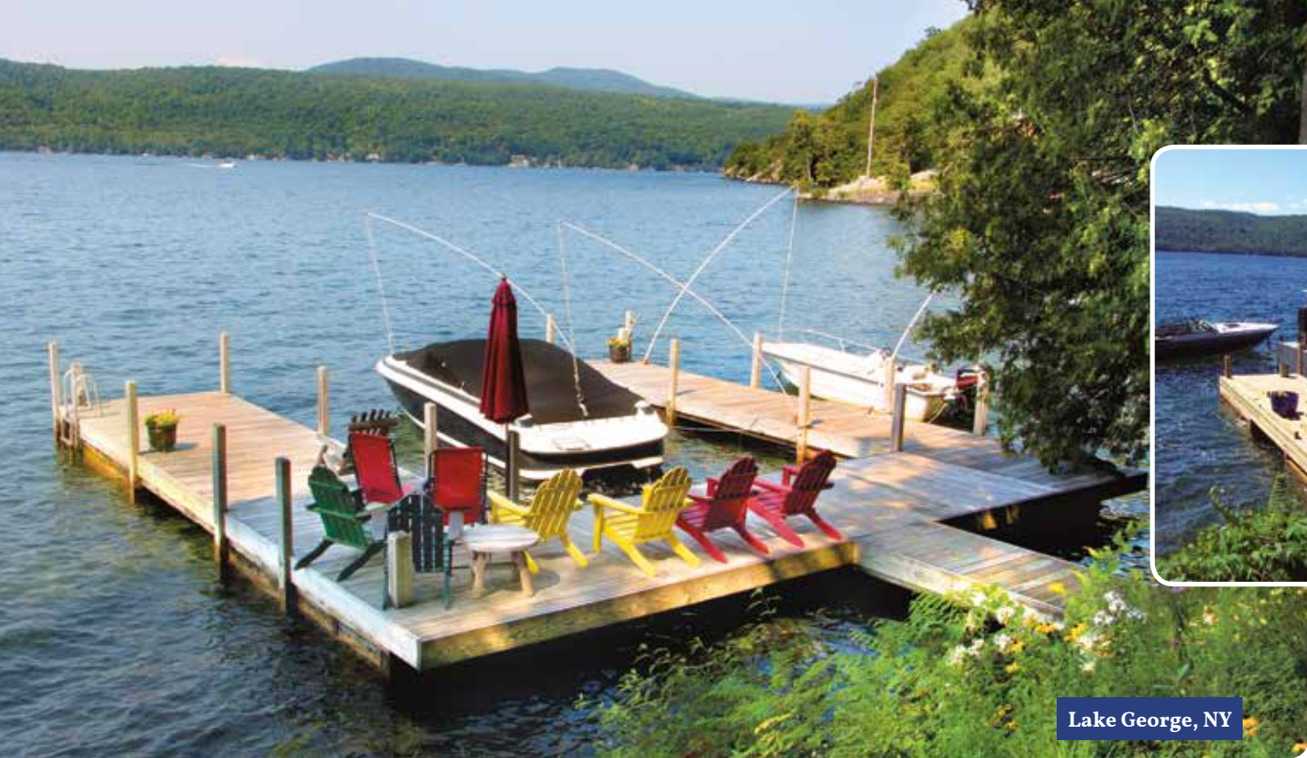
Left: Completed crib dock with rub strakes. Above: During construction with our work boat "Doc".
