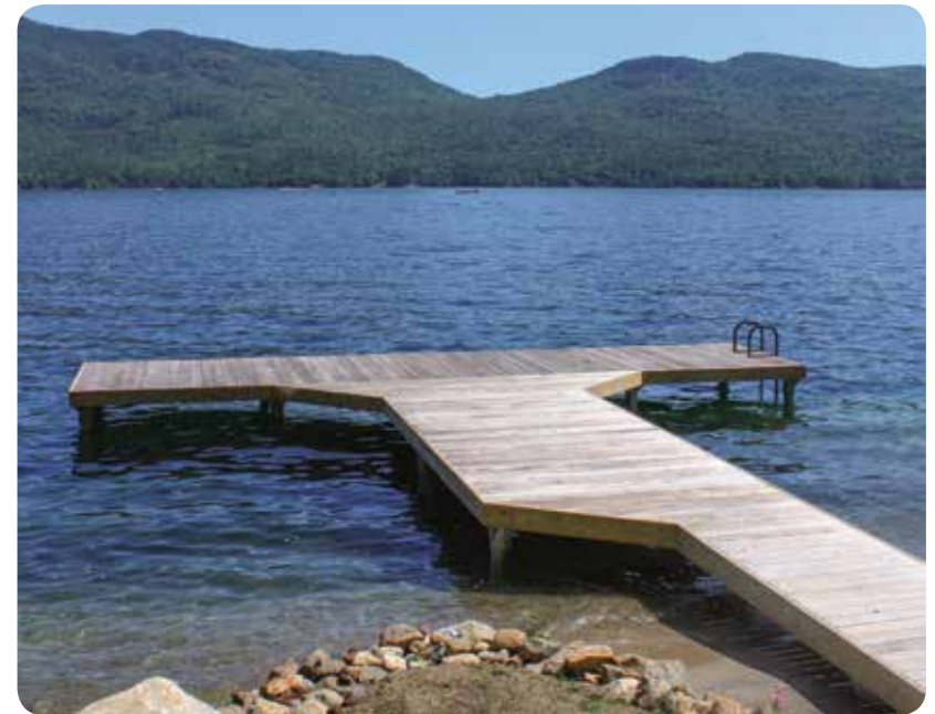
Above: Piles cut below the decking.
