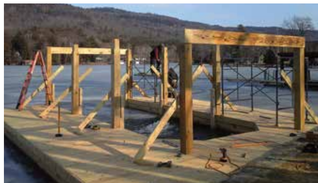
Cribs completed and boathouse structure in progress.
