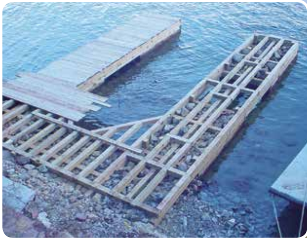
Inset: Crib dock in progress, before final decking installed. Above: Completed crib dock.
