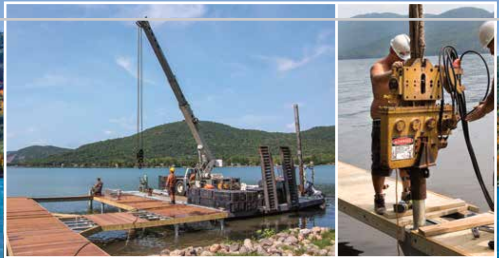
Piles are driven into the lakebed with our workboat and pile driver
