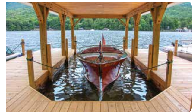
Completed boathouse with crib dock foundation and sundeck.
