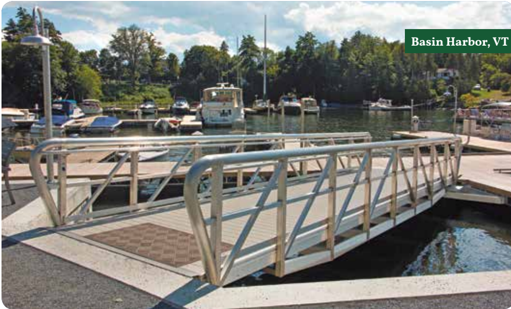
ADA compliant gangway designed to accommodate a golf cart.
