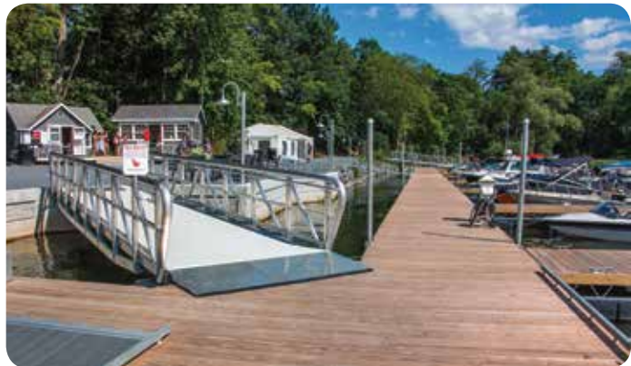
ADA compliant gangway, with golf cart access.
