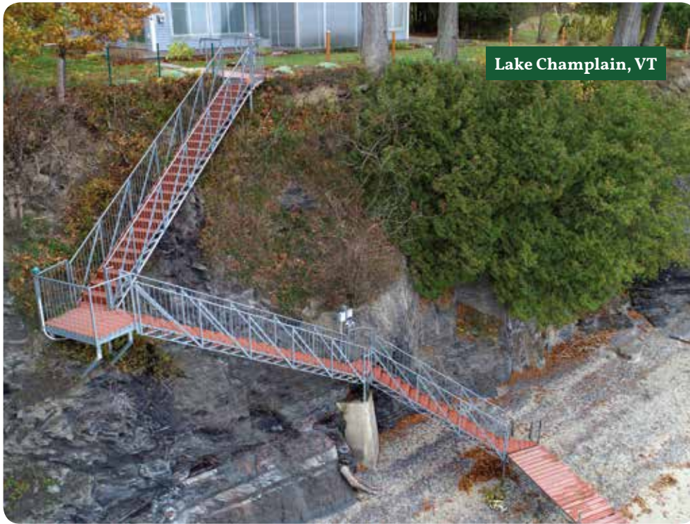
Free span stairs provide access to the water for sites without any shoreline.
