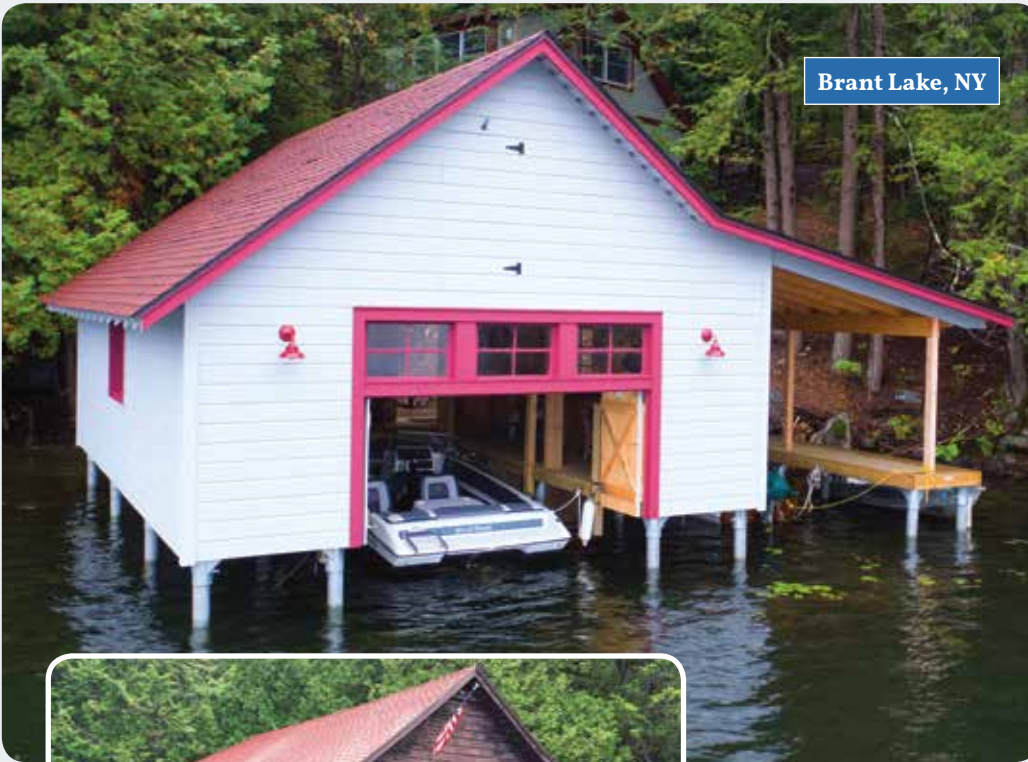
Above: Complete boathouse replacement with new pile dock foundation and designed to replicate the original 100 year-old design.
