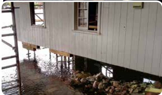
Above: New pile dock foundation installed. Inset: Boathouse lifted with original crib dock foundation removed.
