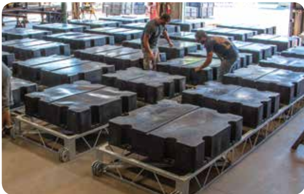
Floats being installed.
