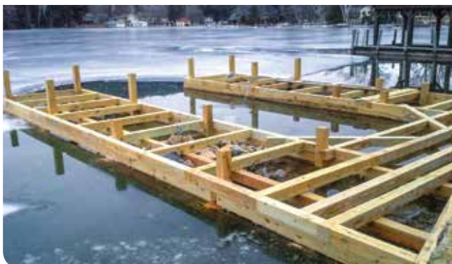
Cribs in place ready for upper timber and decking installation.
