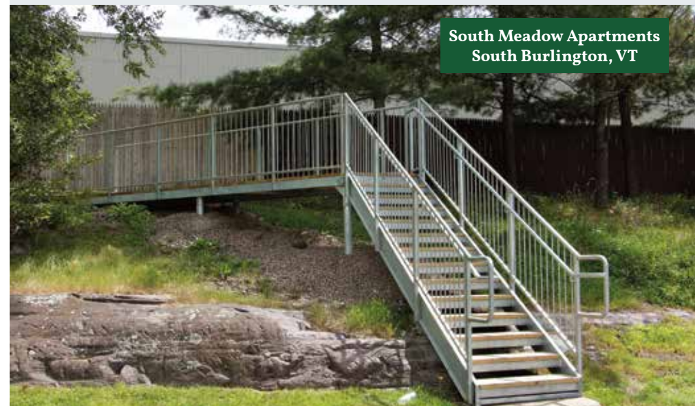
Below: Commercial galvanized steel stairs and walkway with pressure treated treads and spindle rails.
