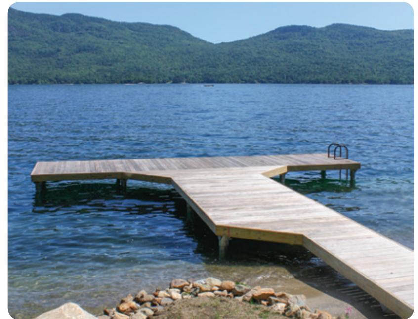
Above: Piles cut below the decking.
