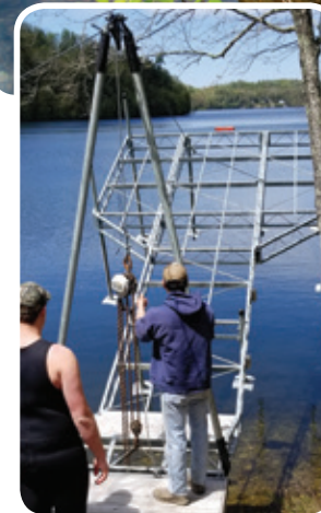
Above: Articulating dock with our shoreside pile platform used as shore mount.
