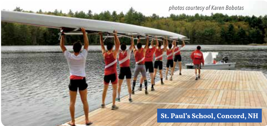
Heavy duty aluminum frame rowing docks with Ipe decking.
