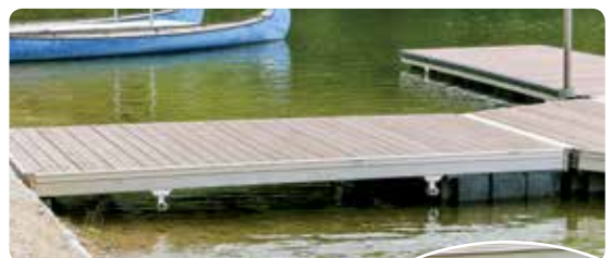
YMCA Camp Coniston, Croydon, NH Axle & Wheel mounts for seasonal installation and removal.
