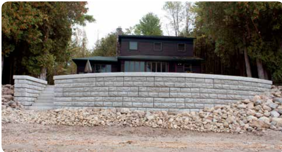
Precast decorative stacked concrete wall.
