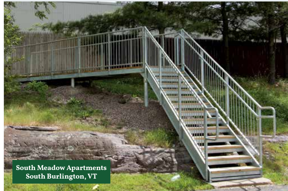
Above: Commercial galvanized steel stairs with pressure treated treads.
