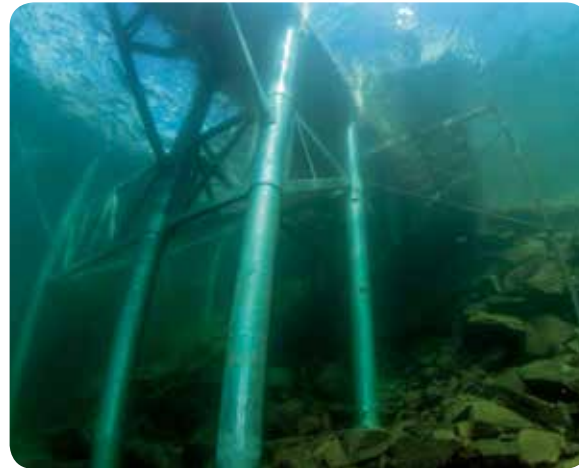
Specialty underwater tooling to install complex permanent structures.
