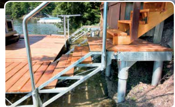
Above: Articulating dock with our shoreside pile platform as a shore mount (inset).
