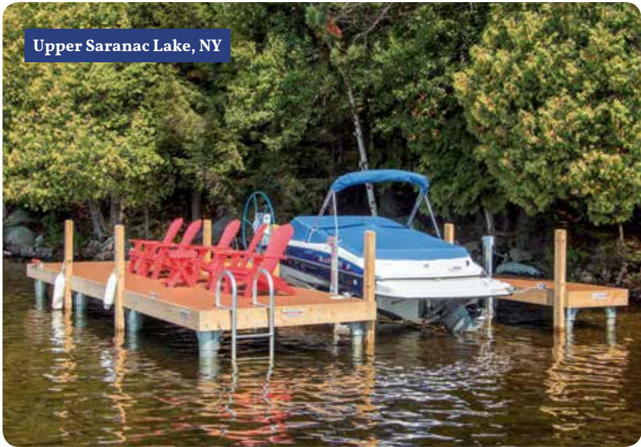
Pile dock with 8" diameter piles on outer supports for protection from ice on exposed side of dock.
