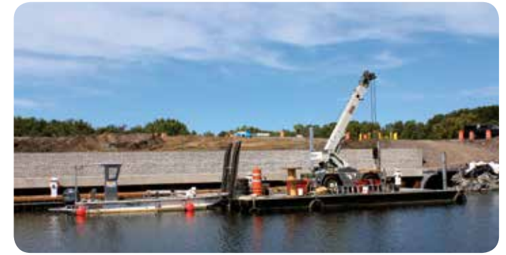
Portable Barge with Crane (above) or Excavator (below)
