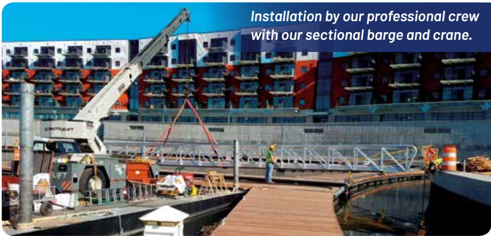
Our sectional barge and crane installing an 80' gangway at Mohawk Harbor.
