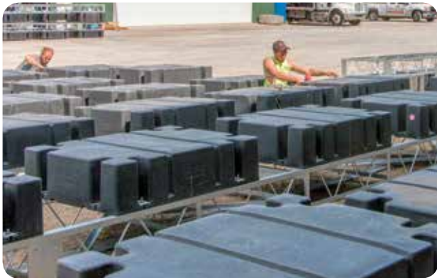
Floats being installed.
