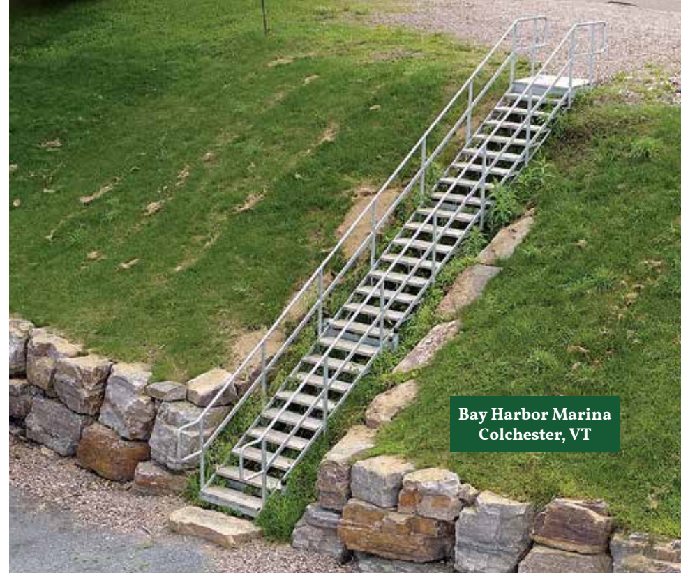
Above: Commercial galvanized steel stairs with pressure treated treads.
