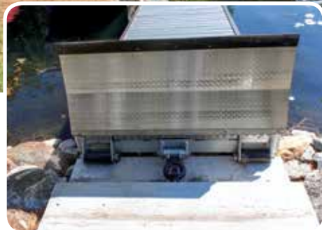
Inset: Concrete hitch pad with pintle hitch. Aluminum tread plate in raised position.
