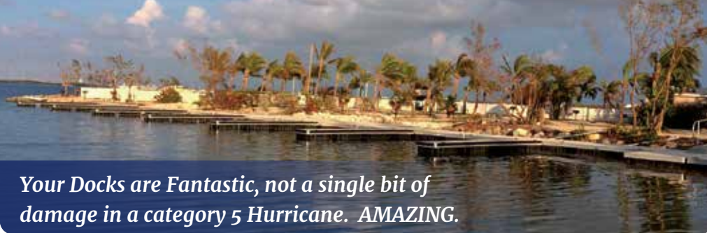
Boyd's Campground, Key West, Florida - AFTER Hurricane Irma
