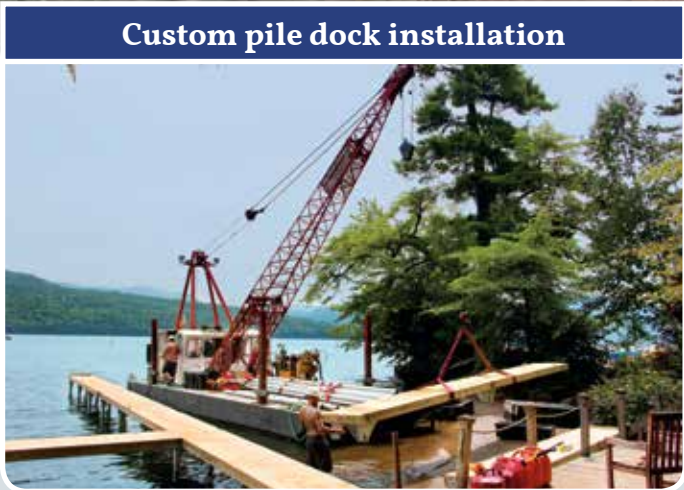
Our work boat "Doc" moves the pile dock sections into position.
