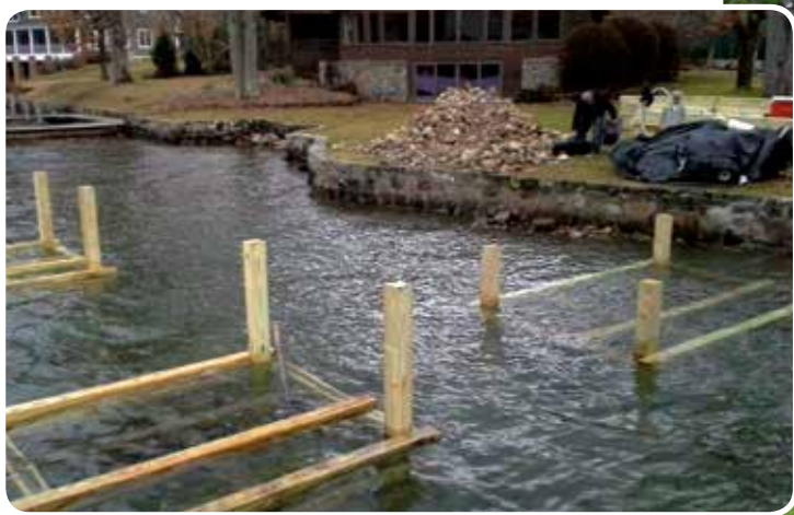
Cribs in place ready for upper timber and decking installation.
