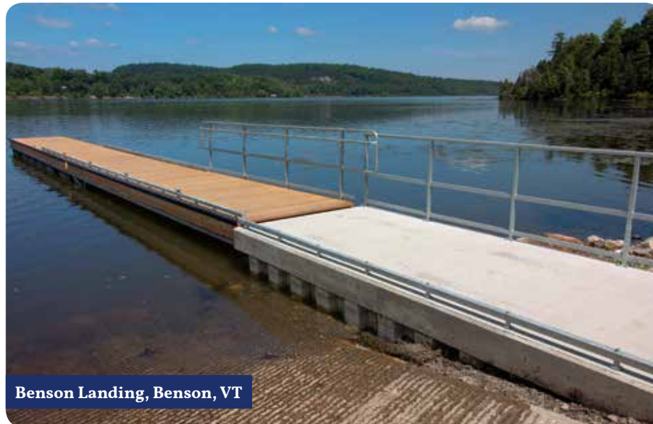
Example of a concrete ramp used as a shore-hitch for this public state boat launch.
