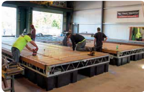
Decking being applied in our workshop.
