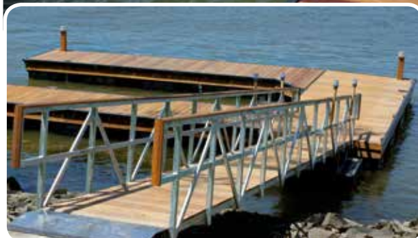
U-shaped heavy duty galvanized steel floating dock with Ipe decking & truss skirting (above & left).
