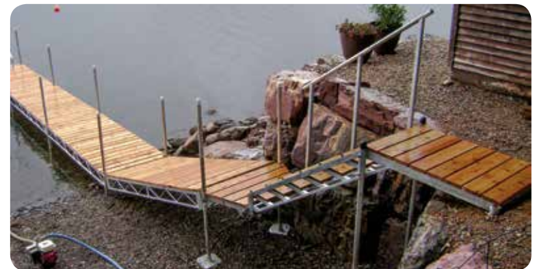
Right: Stairs with lower platform that connects directly to our steel truss leg dock.
