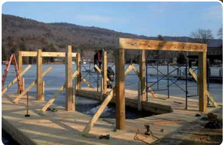
Cribs completed and boathouse structure in progress.
