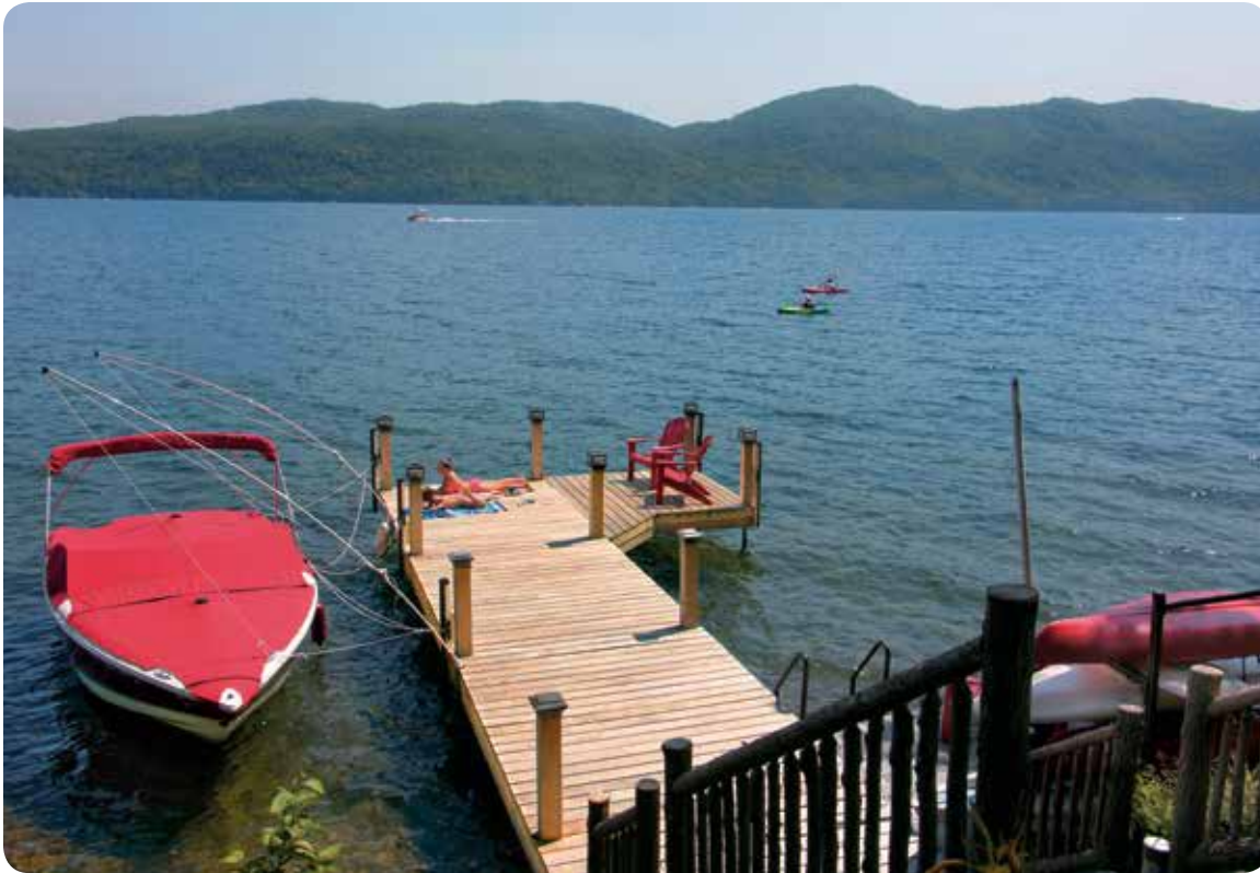
Articulating dock (above) with Ipe decking and custom post covers. Shown raised for winter (below).
