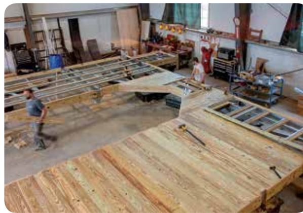
Pile dock in final stages during decking installation.
