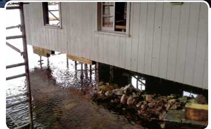
Above: Boathouse lifted with original crib dock foundation removed.
