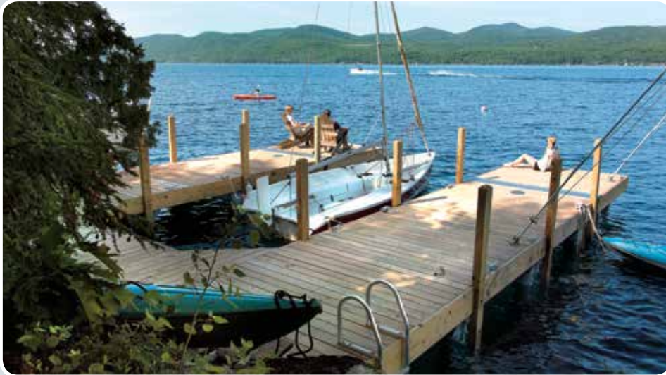
U-shaped pile dock with ends that articulate (raise for winter). End sections of the above dock will hinge for winter storage.
