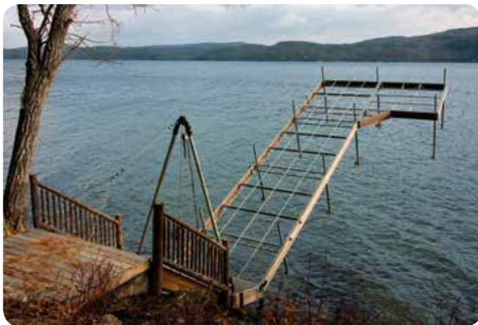
Articulating dock (above) with Ipe decking and custom post covers. Shown raised for winter (below).
