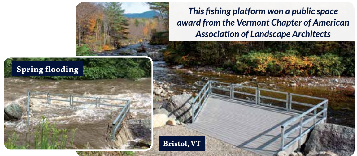
This fishing platform is designed to withstand seasonal flooding.
