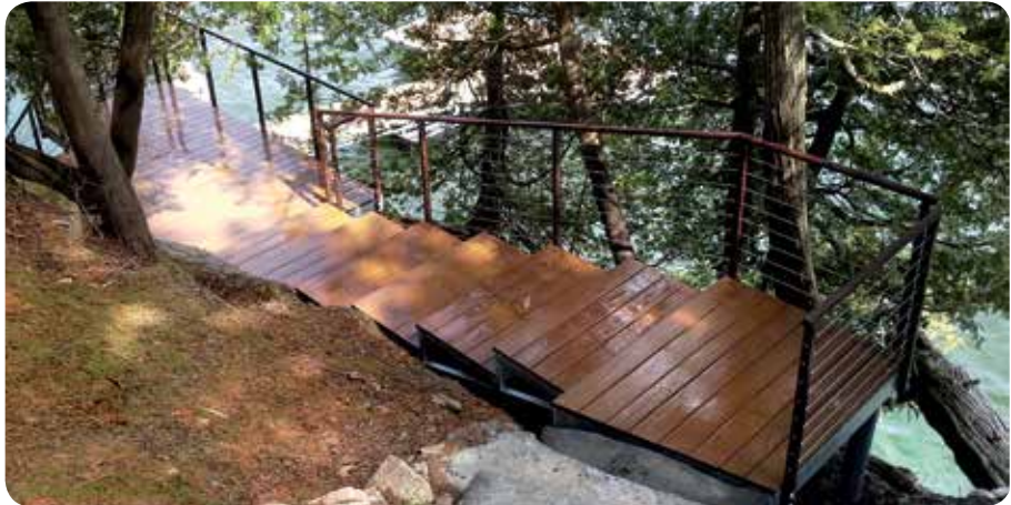
Stainless steel cable rail system provides safety and an open aesthetic appearance.
