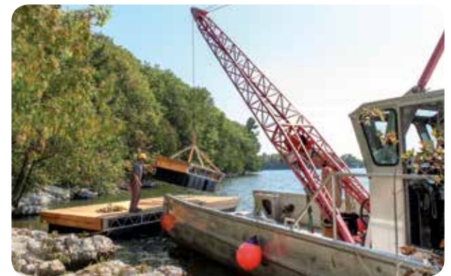
Delivery and installation with our workboat.
