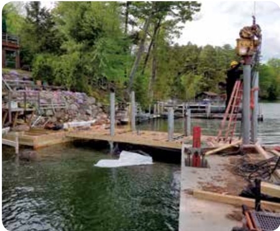
Pile driving typically from 4" to 12" in diameter (larger if necessary).
