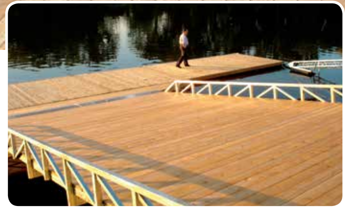
Custom 16' wide ramp.
