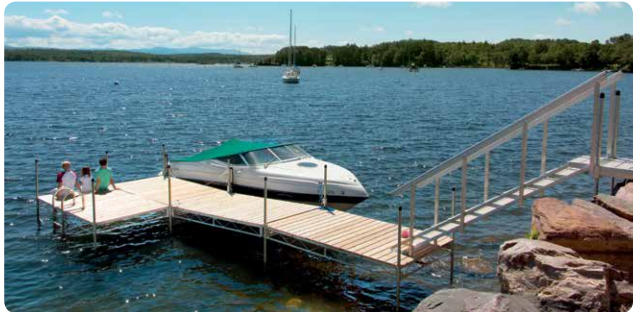
Above: Steel truss leg docks with 6' x 10' sections and cedar decking with our portable aluminum stairs (see p. 18-19) which are utilized as a transition over the rocky shoreline.
