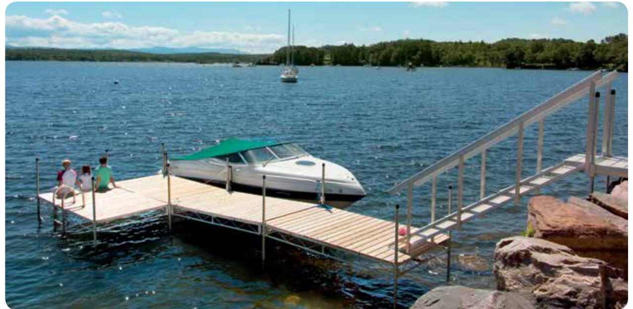
Above: Steel truss leg docks with 6' x 10' sections and cedar decking with our portable aluminum stairs (see p. 18-19) which are utilized as a transition over the rocky shoreline.
