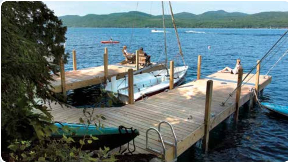
U-shaped pile dock with ends that articulate (raise for winter). End sections of the above dock will hinge for winter storage.
