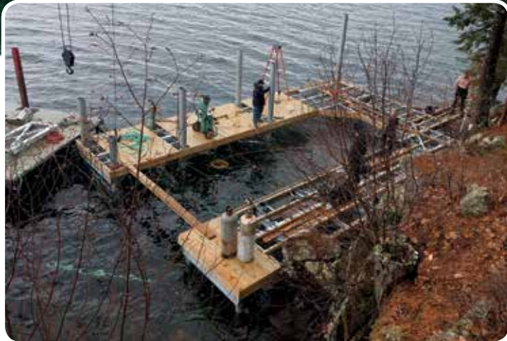
Above: Pile dock in progress prior to boathouse being constructed.
