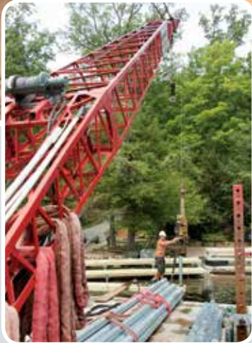
Piles (to support the dock frame) are then driven into the lake bed with our work boat and pile driver.
