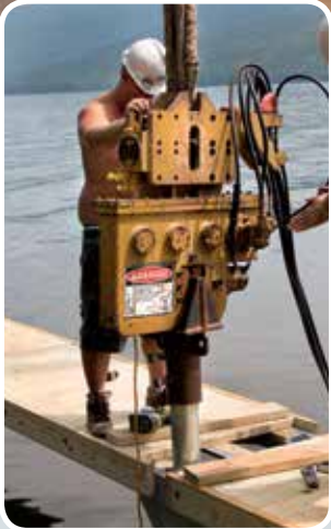
Piles (to support the dock frame) are then driven into the lake bed with our work boat and pile driver.
