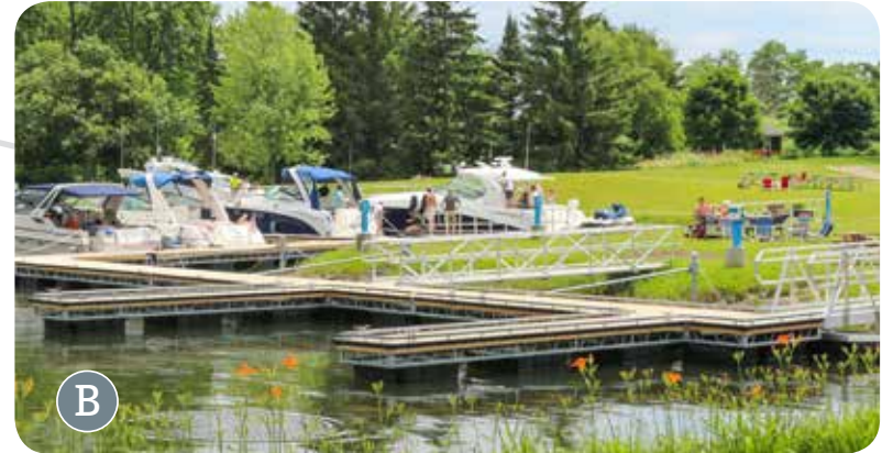
ADA accessible dock with aluminum gangways and ADA curbing on the docks.
