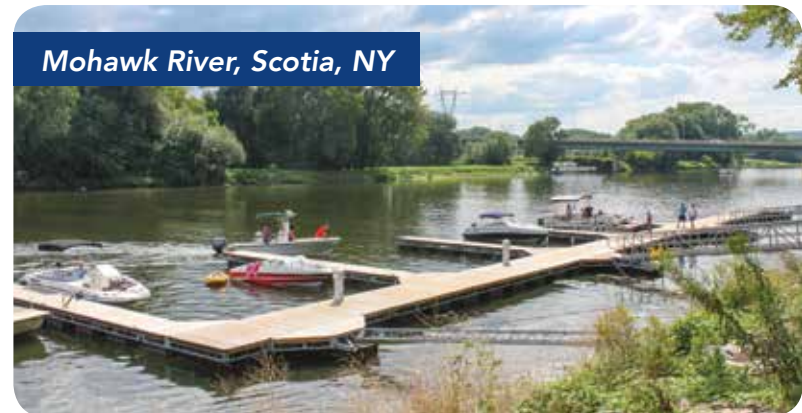
Public transient commercial floating dock anchored with truss style stiff arms mounted to concrete abutments on shore.
