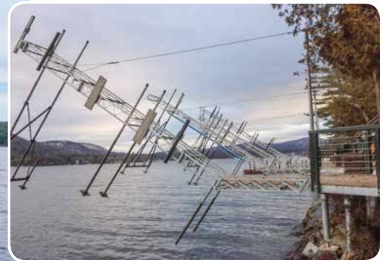
Several articulating docks attached to a shoreside platform at a homeowners association.
