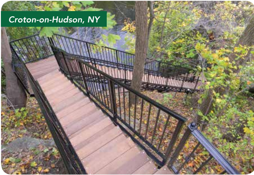
Above: Free span stairs with black powder coating and Ipe treads traversing a vertical drop of approximately 60 feet.
