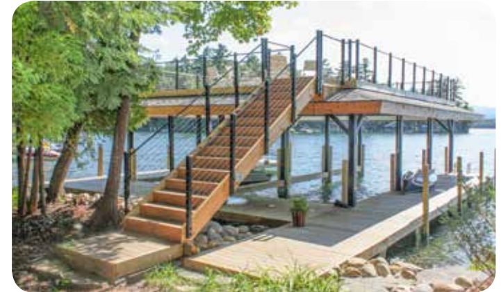
Pile dock with sundeck style boathouse with stainless steel cable rail.
