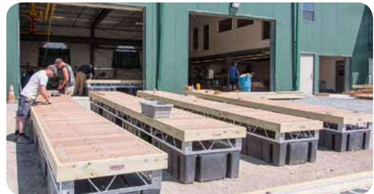
Decking being applied in our workshop.
