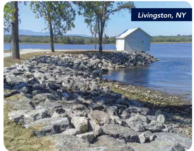
Rip-rap revitalization project on the Hudson River on a historic pier.
