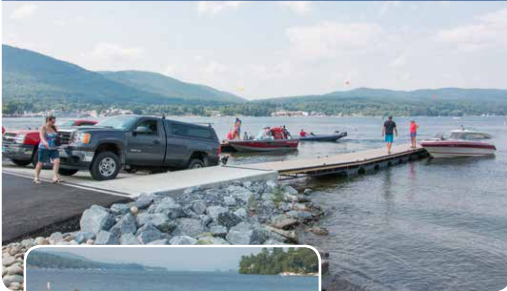
Commercial steel truss floating dock with powder coated finish in use at the boat access launch facility at The Village of Lake George.
