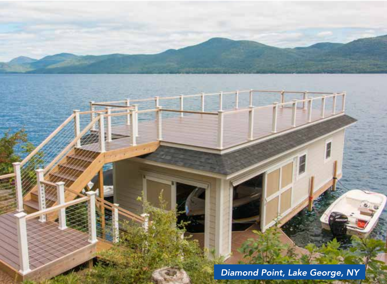
Pile dock with steel frame sundeck style boathouse & composite rails.
