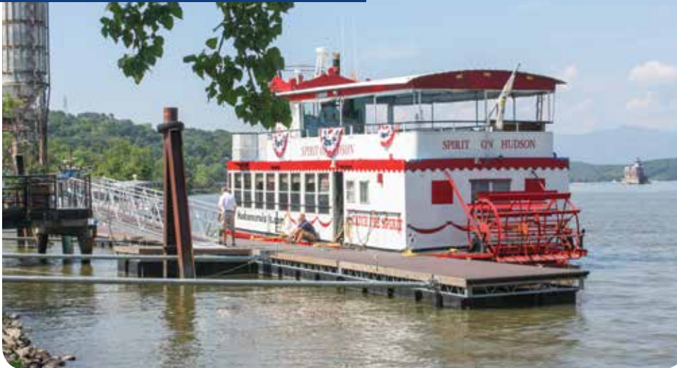
Commercial floating docks in use for tour boats at a municipal park.
