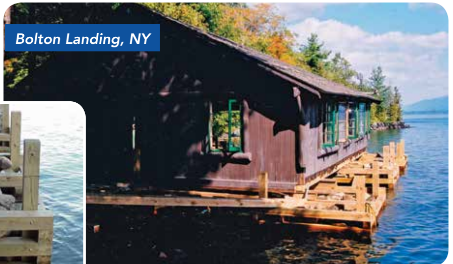
Replacement crib dock foundation for older boathouse.
