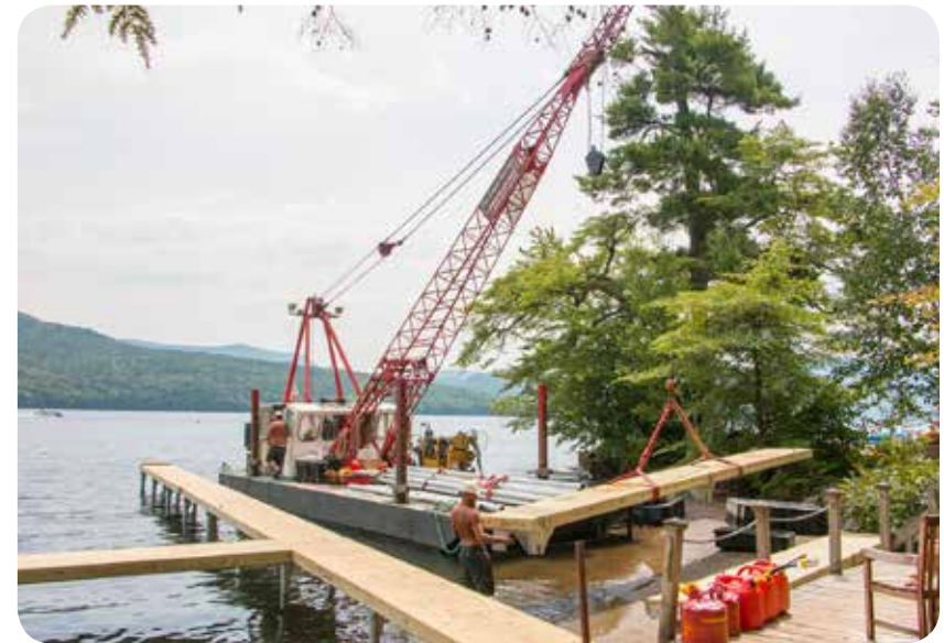
Our work boat "Doc" moving a pile dock section into position.
