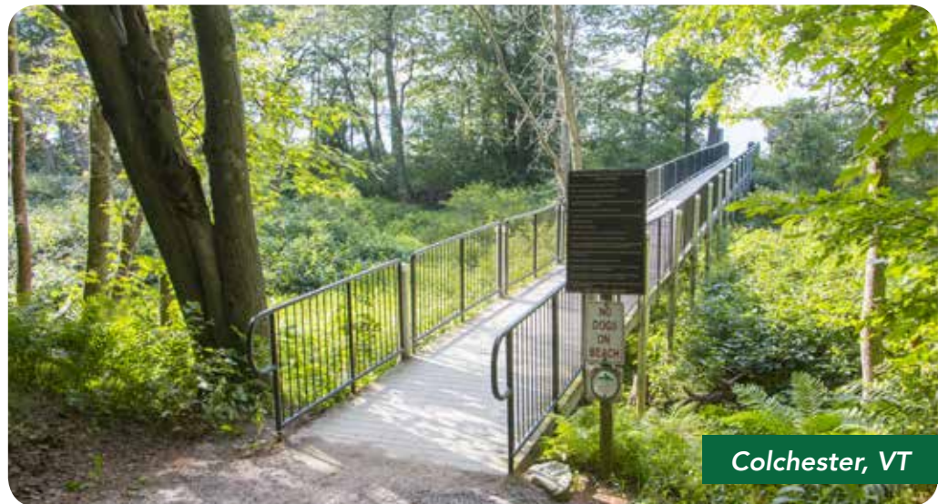
Pedestrian beach access through wetlands using our commercial pile dock system with powder coated handrails.
