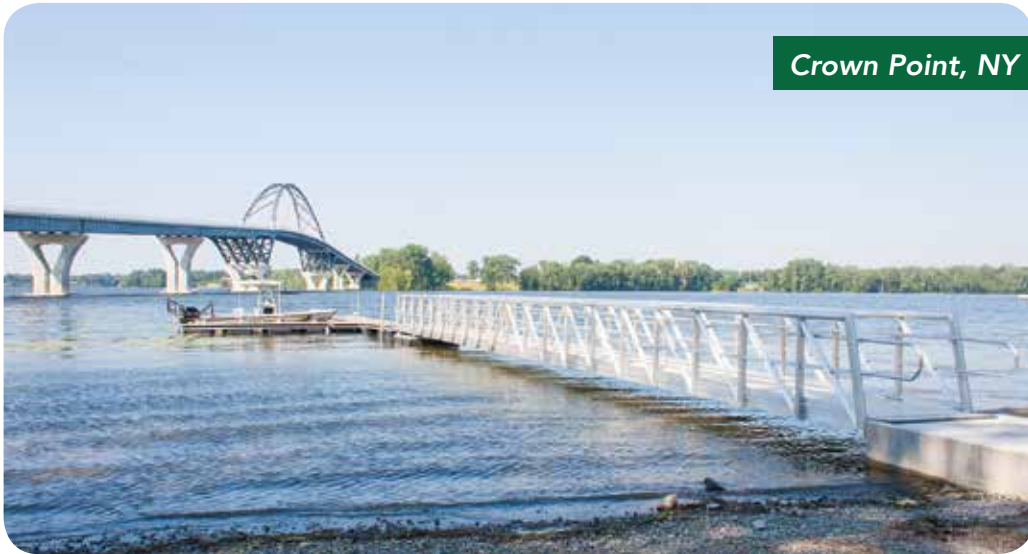
Above & Right: 5' x 80' ADA compliant gangway for NYSDEC boat launch.
