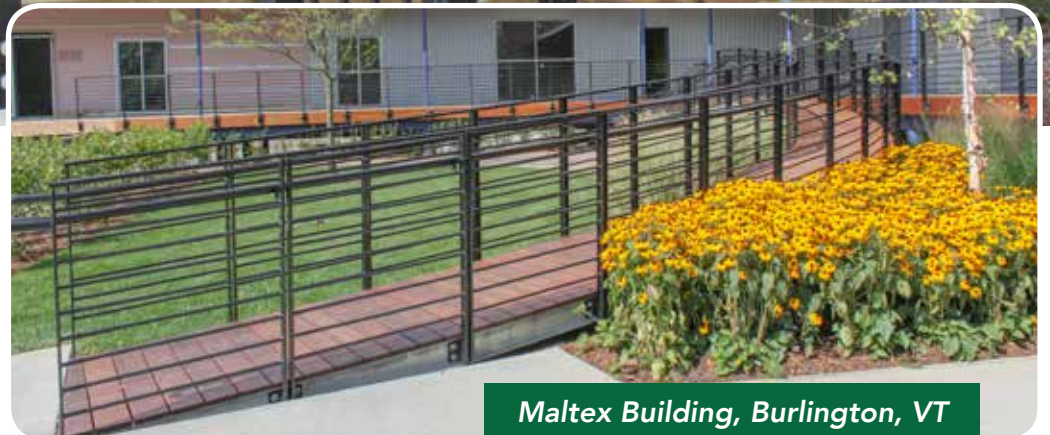
Commercial galvanized steel ADA access ramp with Ipe decking & black powder coated steel railings.
