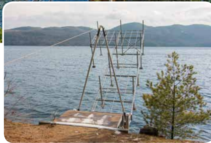
Above: Articulating dock attached to a shoreside platform and a 5,000 lb. hydraulic boat lift.
