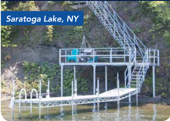
Shoreside platform used as a transition for the steel stair system and waterfront deck area for a site with no beach.
