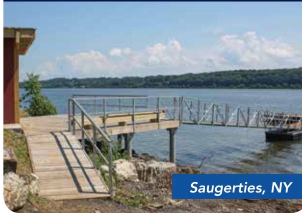
Combined use for a shoreside platform & a shore connection system for our heavy duty floating dock systems.
