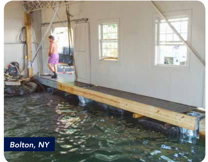
Below: Permanent pile dock system installed in place of original crib dock foundation.
