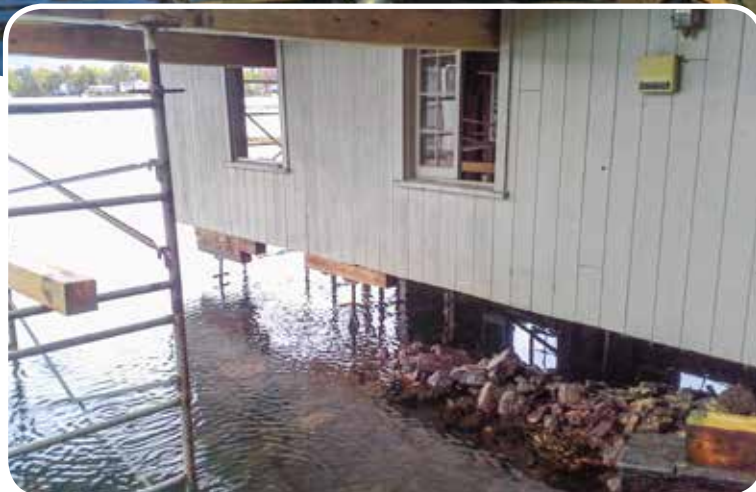
Boathouse lifted with original crib dock foundation removed.
