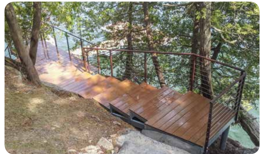
Stainless steel cable rail system provides safety and an open aesthetic appearance.
