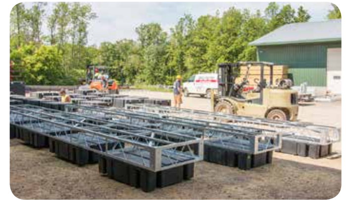
Installation of floats onto galvanized dock frames.
