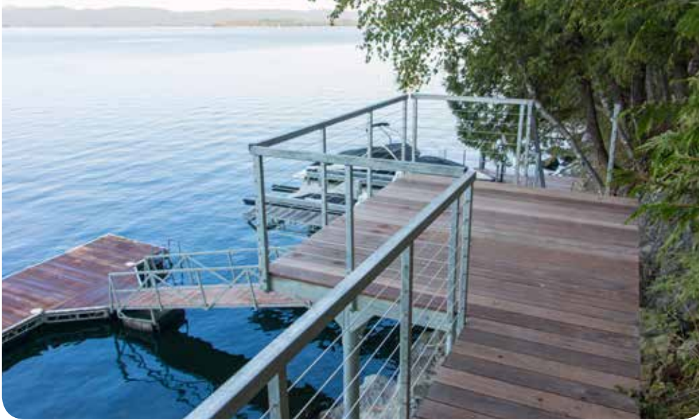
Shoreside platform with stainless steel cable rail.
