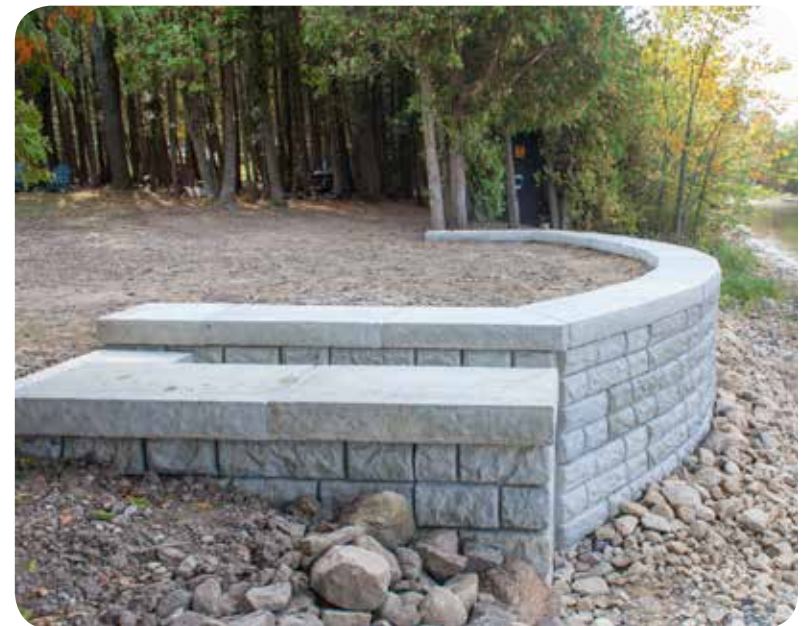
Pre-cast decorative stacked concrete wall.
