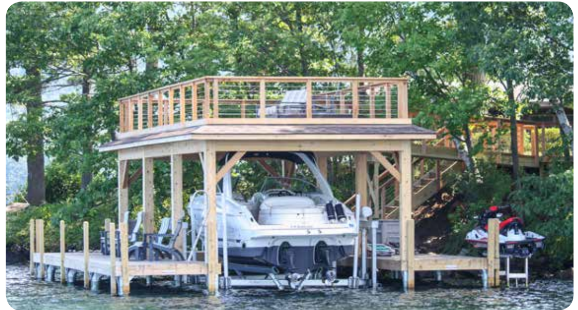
U-shaped pile dock, 9,000 lb. Ultimate boat lift & sundeck style boathouse with stainless steel cable rail.
