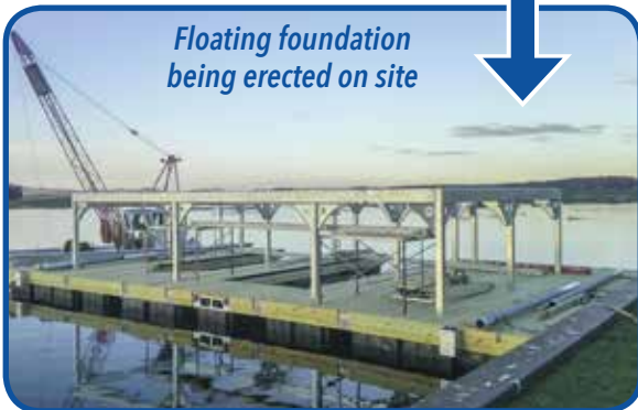
Above: Floating foundation and boathouse support structure during production in our shop.
