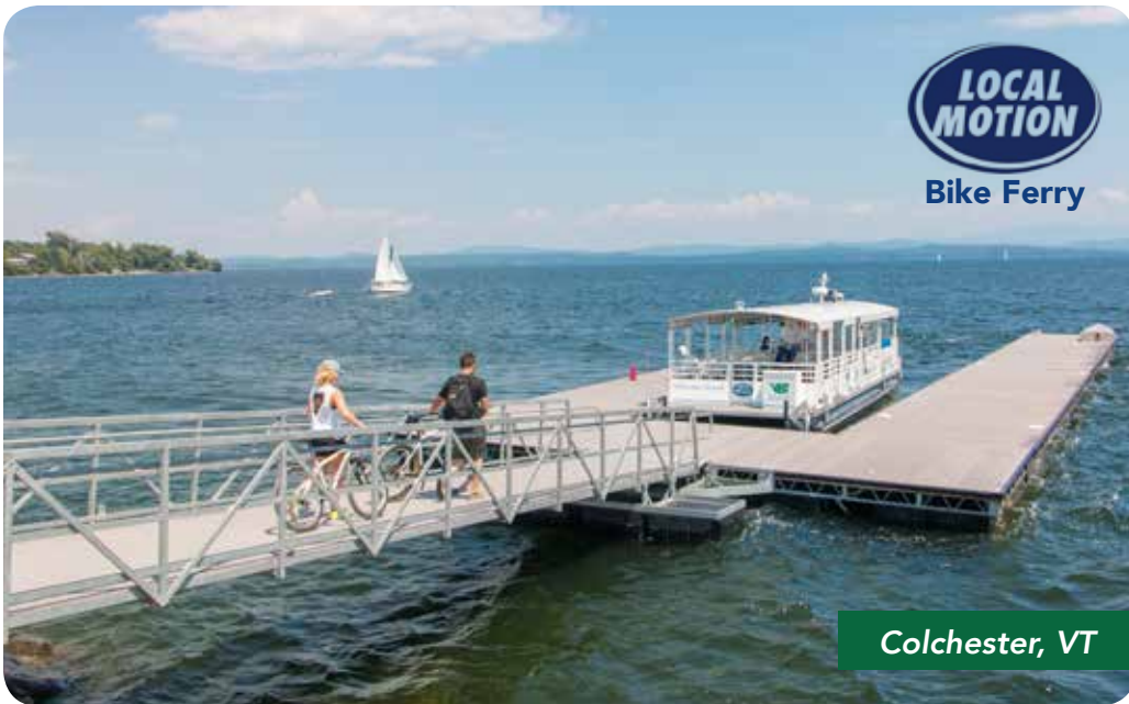
Industrial grade galvanized steel truss frame with built-in wave attenuator for a very exposed area of the lake.
