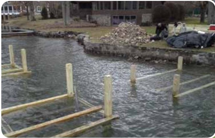
Cribs in place for new boathouse foundation.
