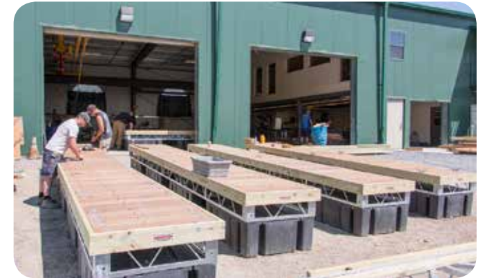
Final decking being installed at our production facility.
