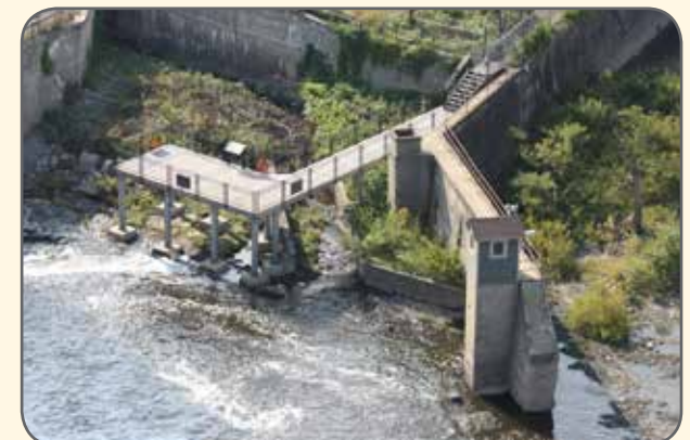
Observation platform at hydro-power plant
