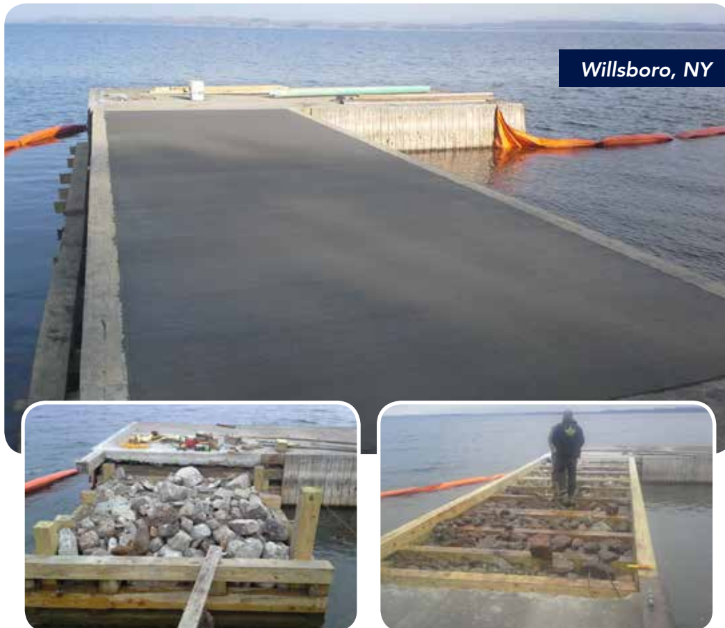
Total reconstruction of a concrete pier.
