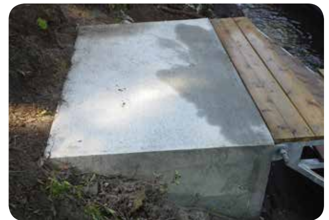
Above: Concrete pad shore mount.
