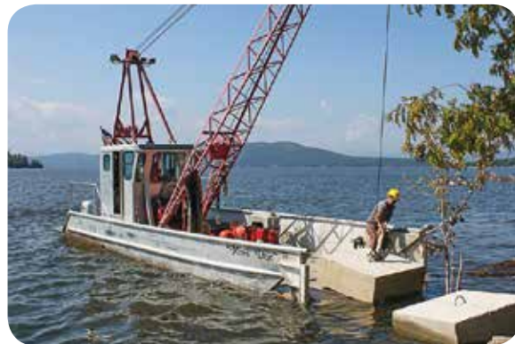
Our work boat "Miss Doc" setting anchors for a floating dock system.
