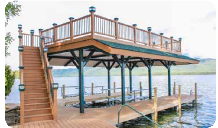
Pile dock with steel frame sundeck style boathouse & composite rails.
