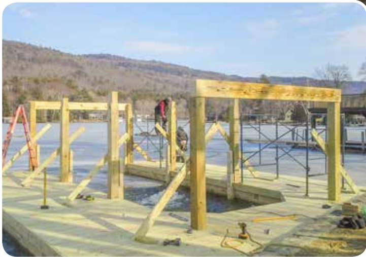
Cribs completed and boathouse structure in progress.
