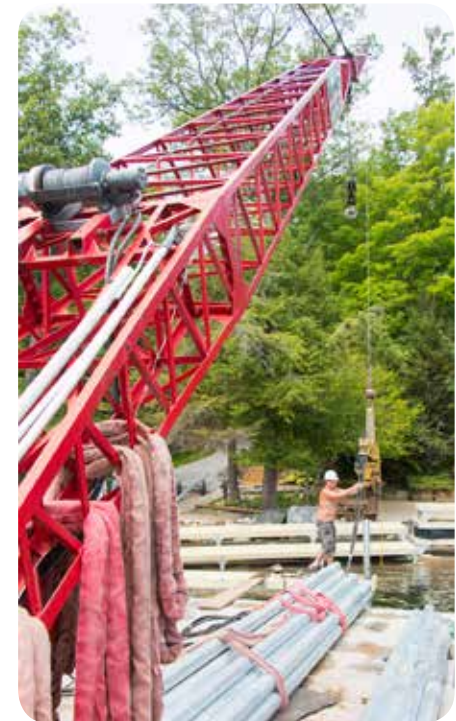
Piles (to support the dock frame) being driven into the lake bed with our work boat and pile driver.
