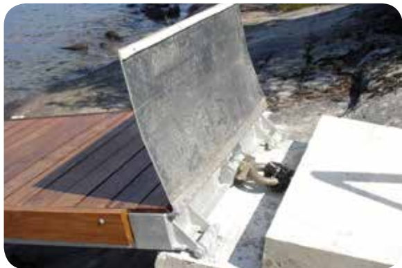
Concrete hitch pad with pintle hitch - aluminum tread plate in raised position.
