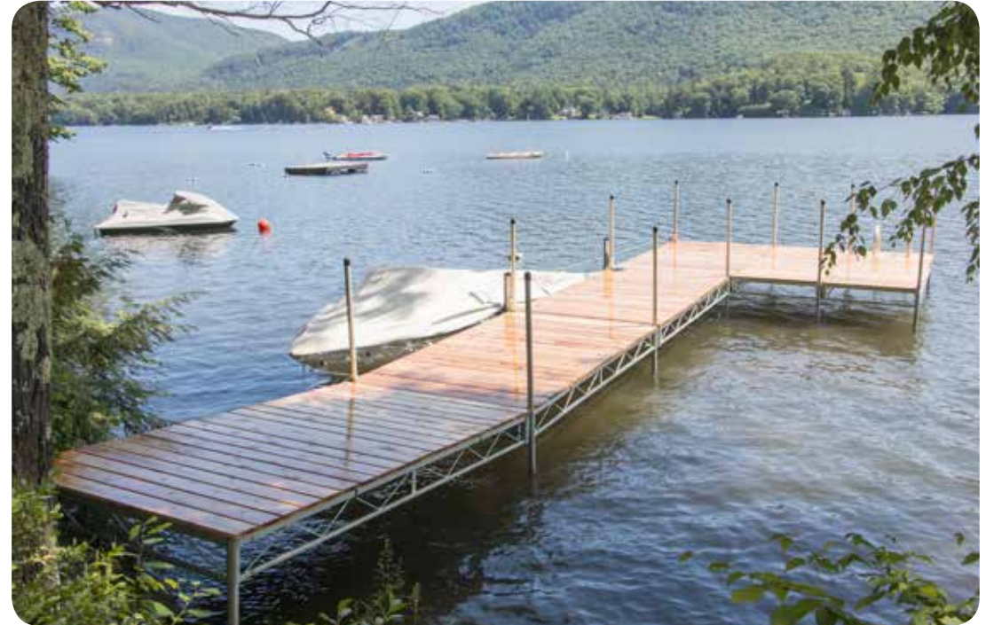
Heavy duty steel truss dock with 6' x 10' sections and cedar decking.
