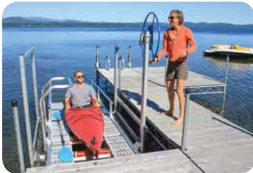
30" handwheel easily raises & lowers the launch platform.
