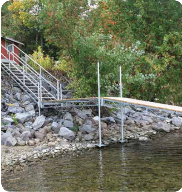
Steel truss leg docks used to transition over a rocky shoreline.
