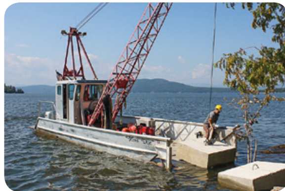
Our work boat "Miss Doc" setting anchors for a floating dock system.
