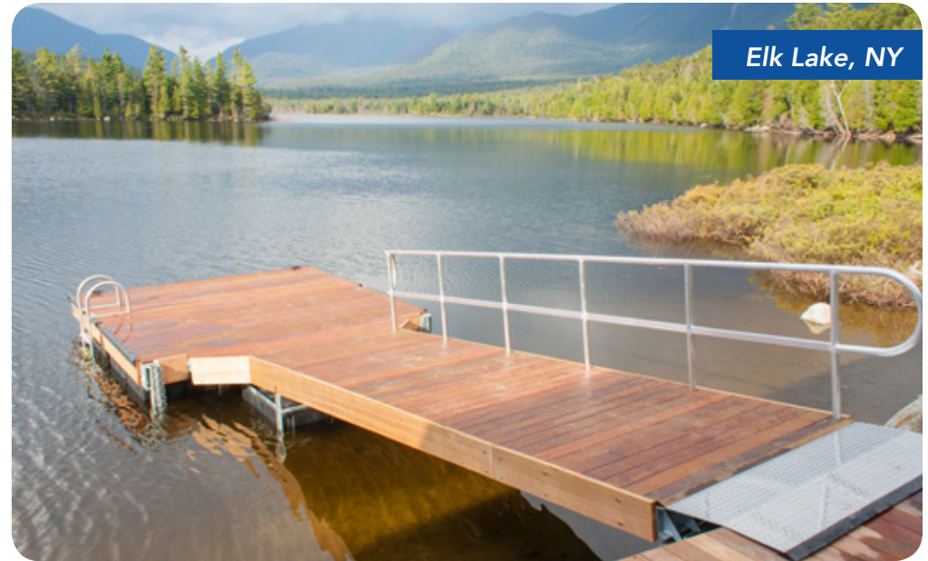
T-shaped floating dock with Ipe decking & truss skirt board.
