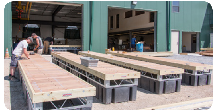
Decking being applied in our workshop.
