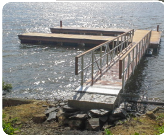
U-shaped heavy duty galvanized steel floating dock with Ipe decking & truss skirting (above & left).
