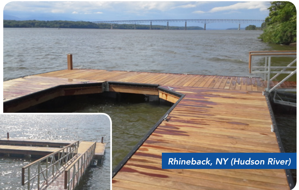
U-shaped heavy duty galvanized steel floating dock with Ipe decking & truss skirting (above & left).
