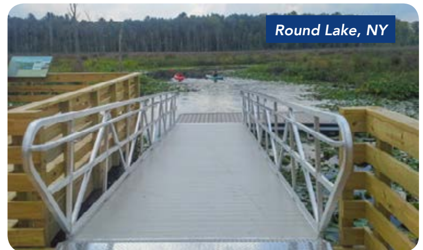
Aluminum gangway & our heavy duty aluminum floating dock at a NYSDEC public access for paddle crafts.
