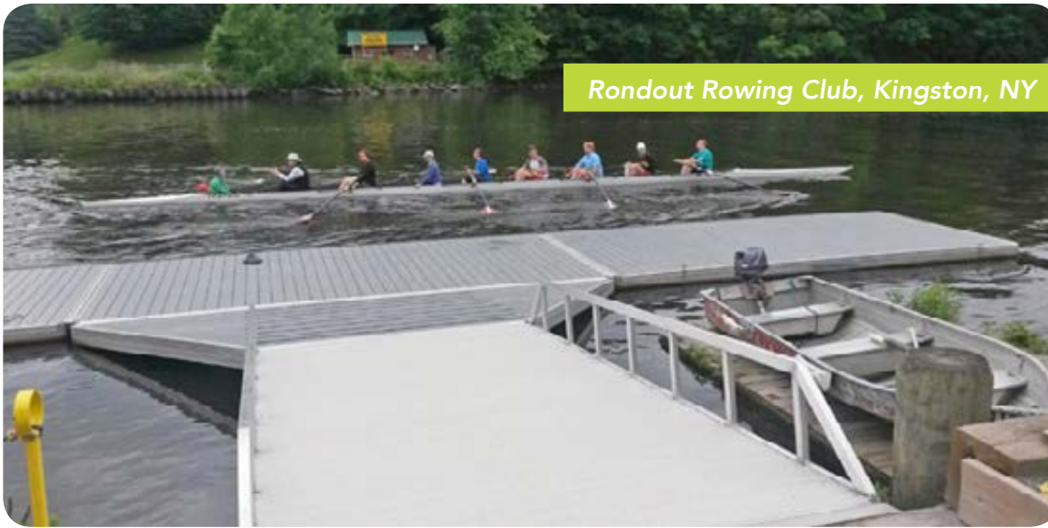
16' x 8' aluminum gangway with float frame for tidal fluctuations.
