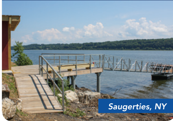
Combined use for a shoreside platform & a shore connection system for our heavy duty floating dock systems.
