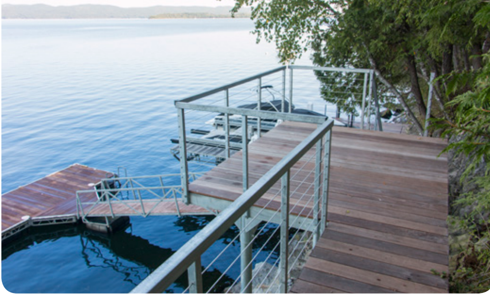
Shoreside platform with stainless steel cable rail.
