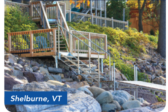
Shoreside platform transitioning to a heavy duty steel truss leg dock.
