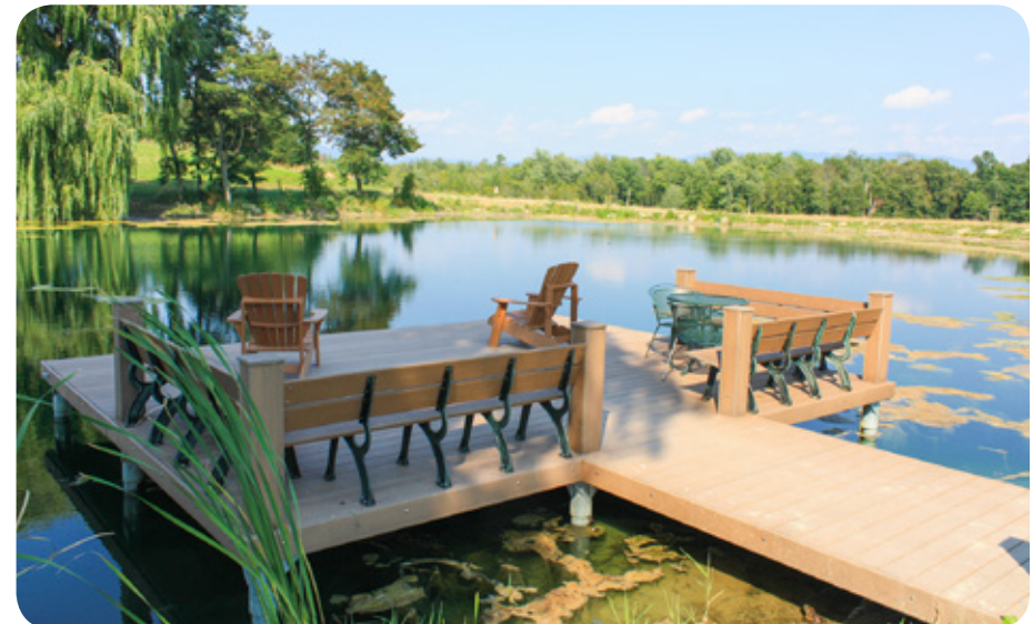
Pile dock on a man-made pond.
