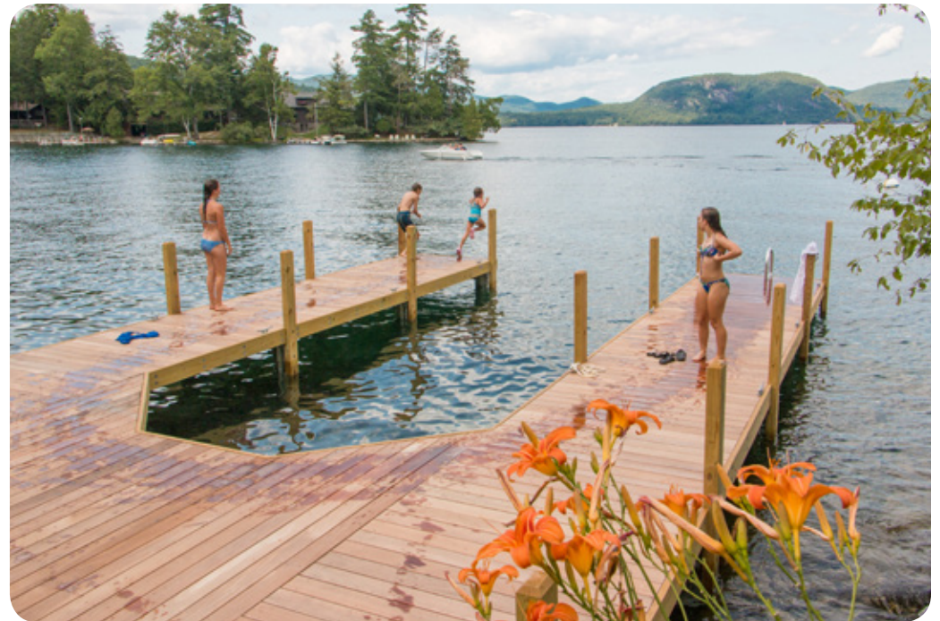
U-shaped pile dock with Ipe decking – pilings cut below decking.
