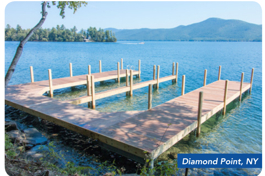
U-shaped pile dock with a slip divider / catwalk.
