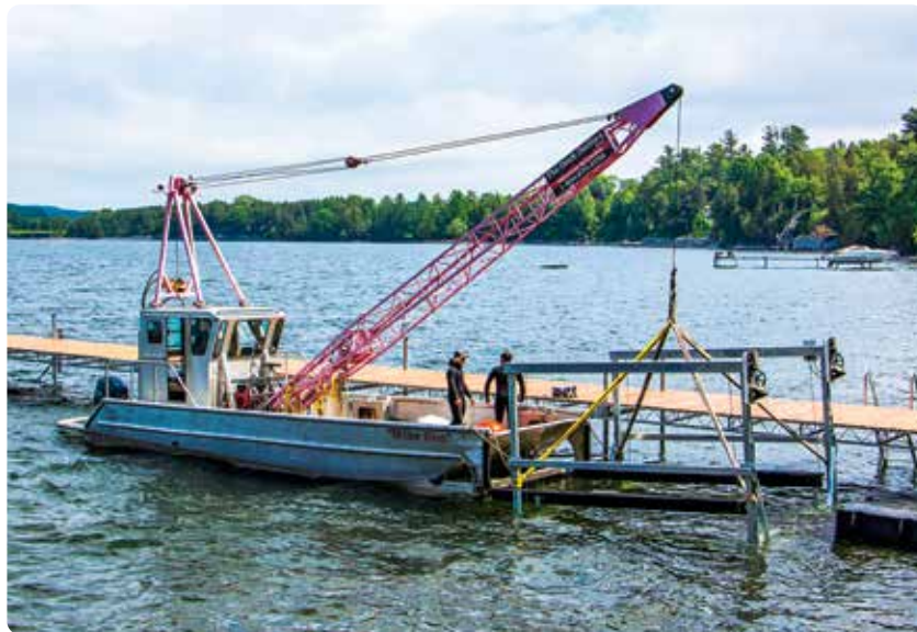
Ultimate lift being installed by one of our crews using our portable workboat "Miss Doc".
