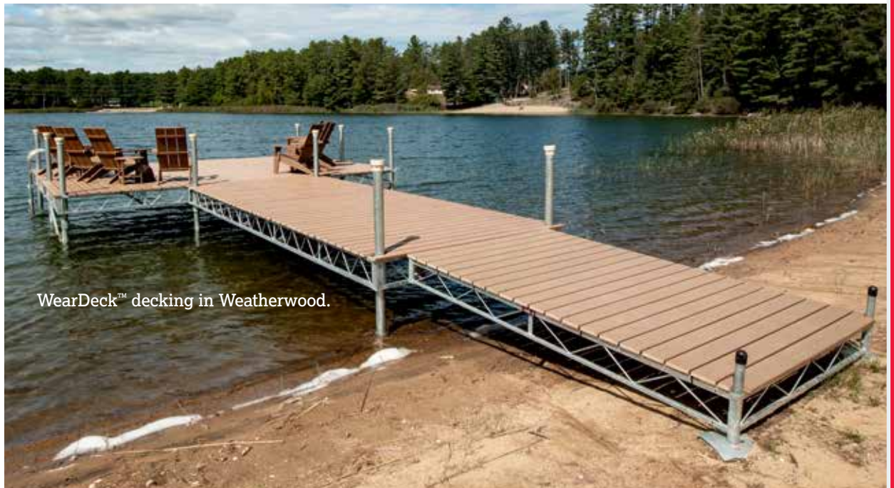
Mega Duty dock system, accessed by our custom steel stairs and shoreside platform, which provides deck space on this steep shoreline ( see our Custom Catalog ).
